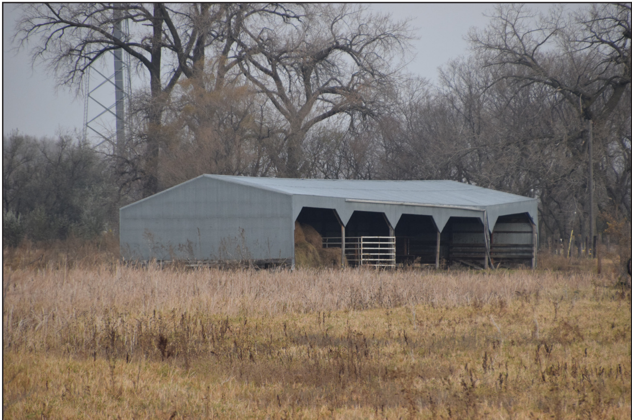
Figure 92. 32RI917, Feature 6, south and east elevations, view facing northwest.
