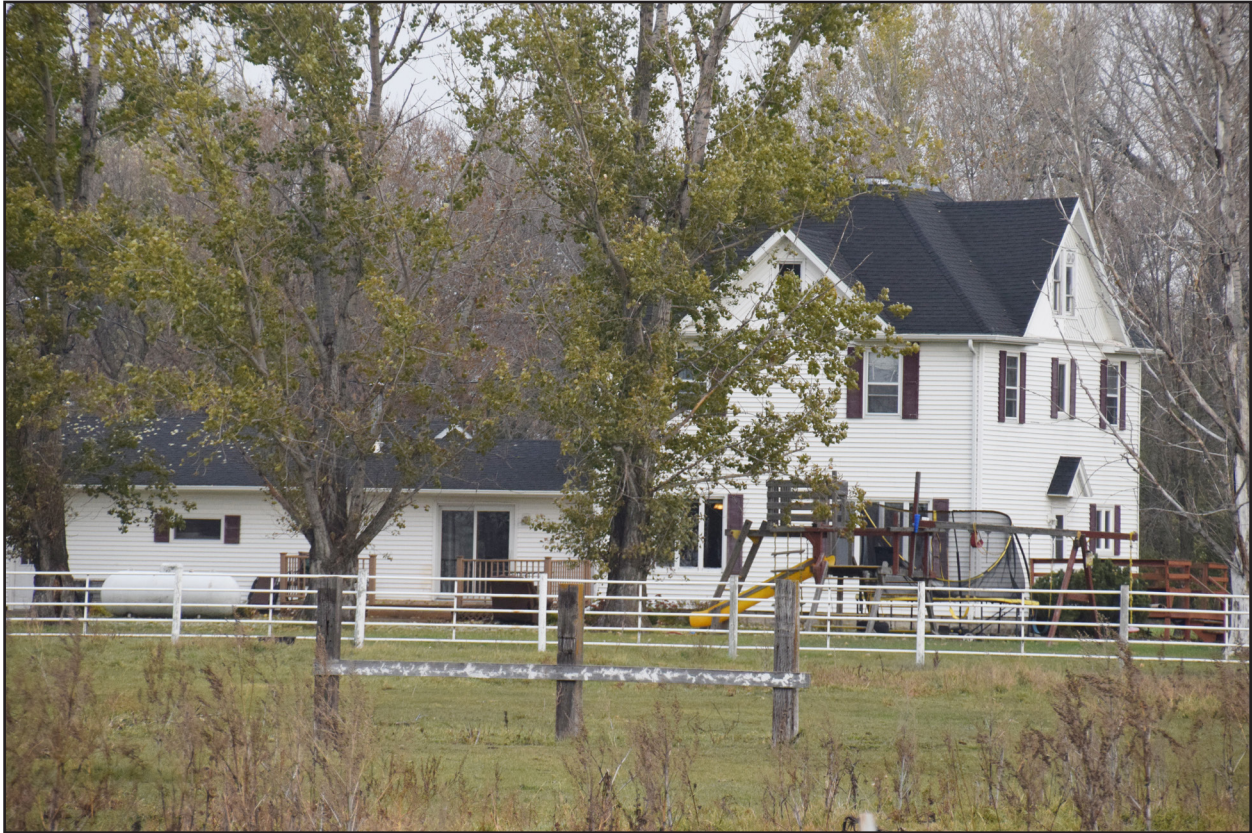
Figure 87. 32RI917, Feature 1, south and east elevations, view facing northwest.
