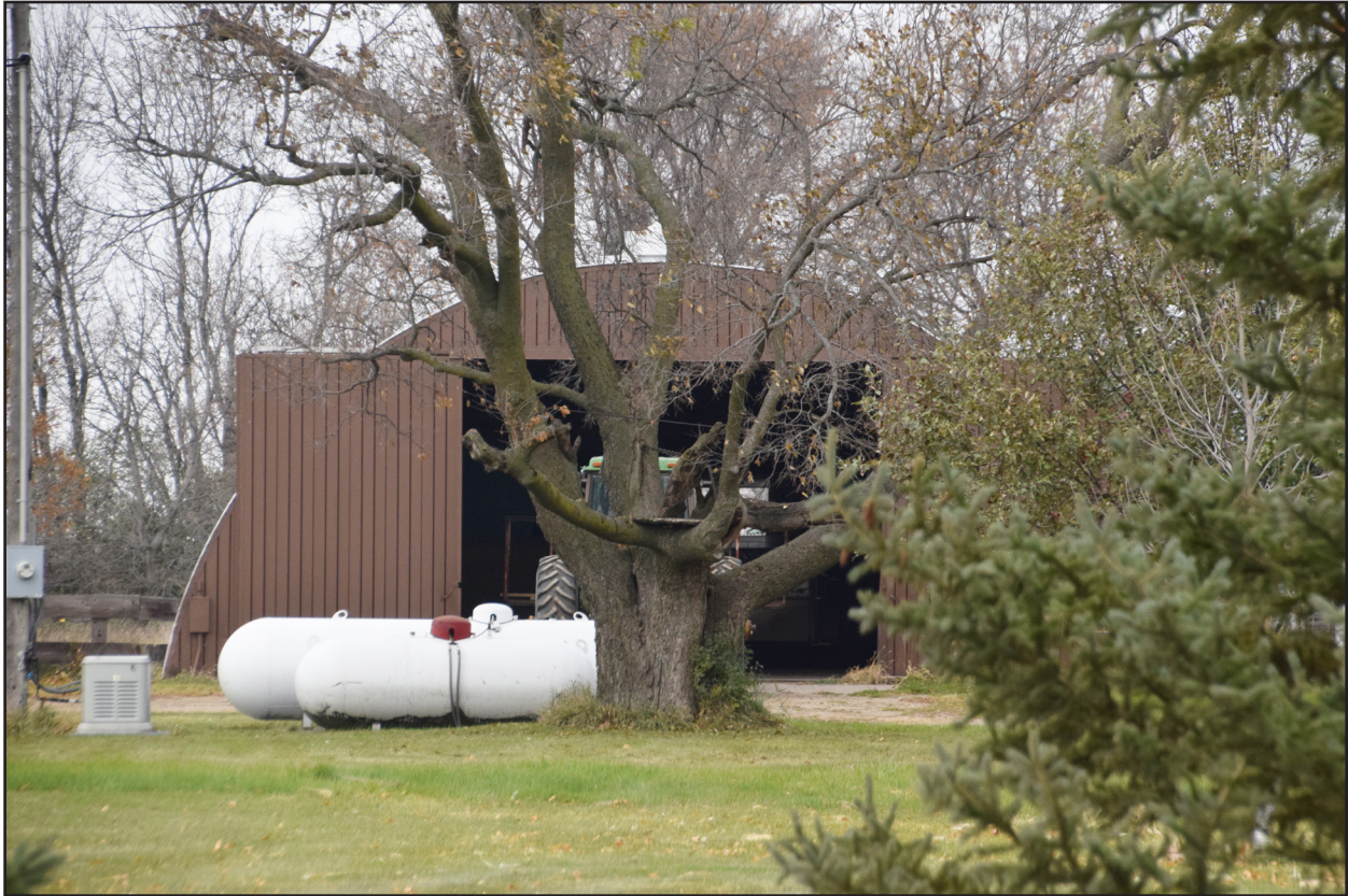
Figure 108. 32RI919, Feature 3, east elevation, view facing west
