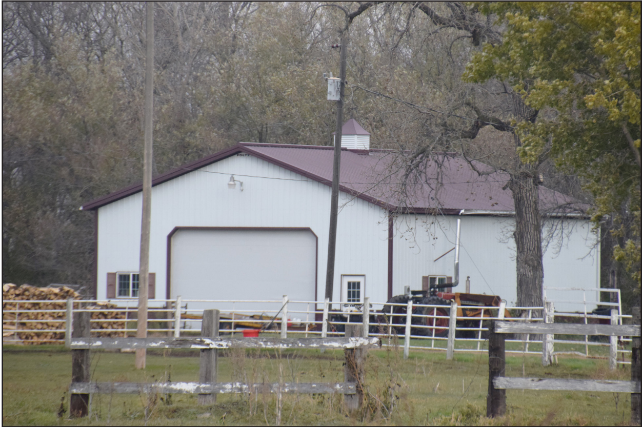
Figure 93. 32RI917, Feature 7, south and east elevations, view facing northwest.
