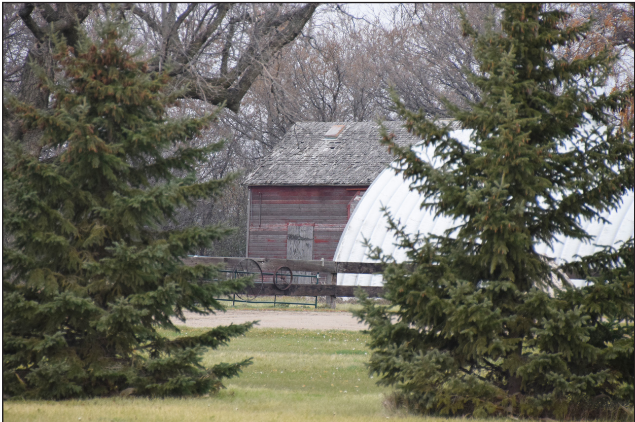
Figure 109. 32RI919, Feature 4, south elevation, view facing northwest.
