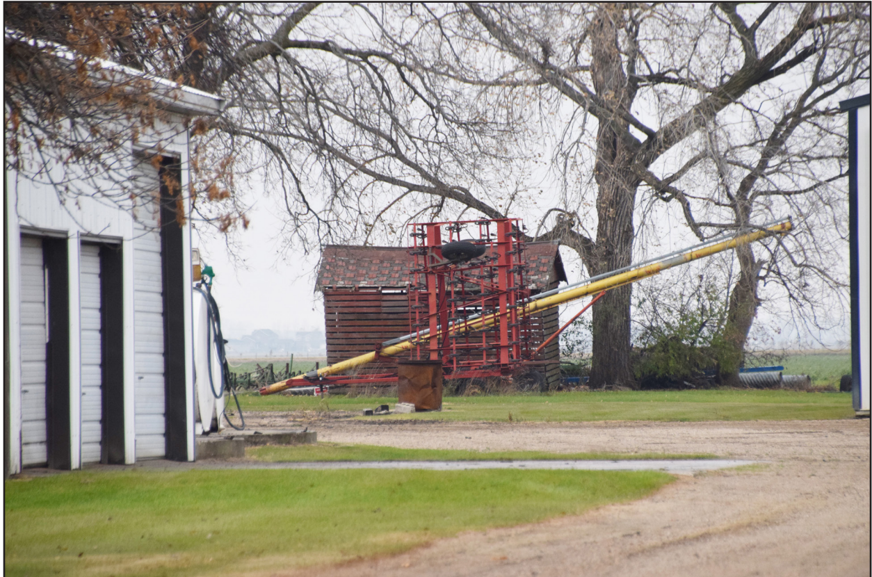
Figure 103. 32RI918, Feature 7, north and east elevations, view facing southwest.
