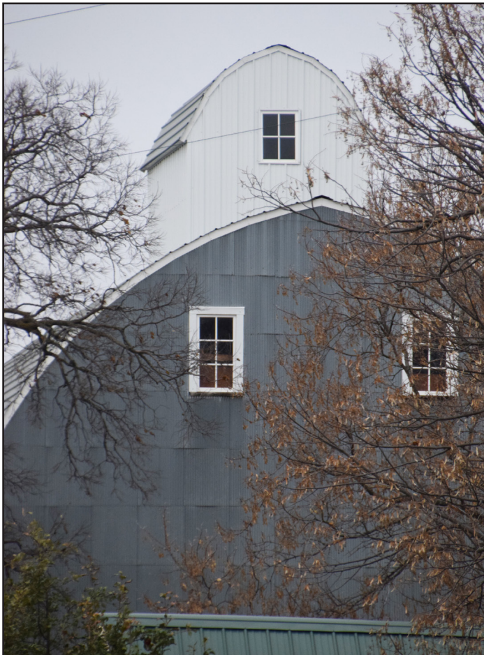
Figure 111. 32RI919, Feature 6, east elevation, view facing west.
