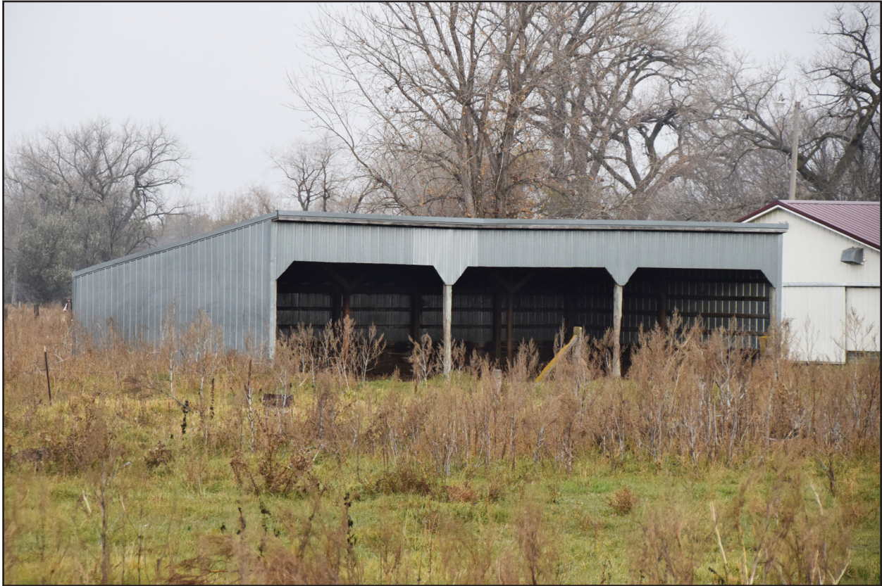
Figure 91. 32RI917, Feature 5, south and east elevations, view facing northwest.
