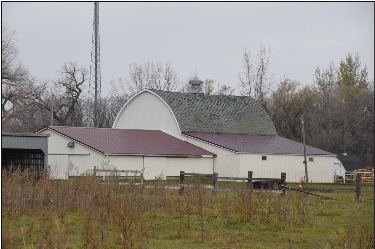
Figure 88. 32RI917, Feature 2, south and east elevations, view facing northwest.
