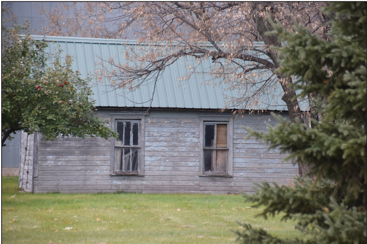
Figure 107. 32RI919, Feature 2, east elevation, view facing west.
