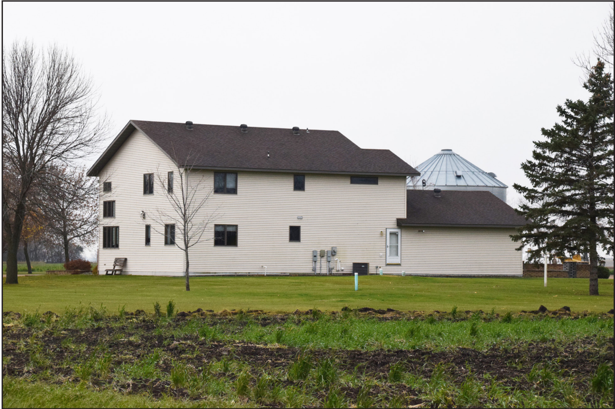
Figure 97. 32RI918, Feature 1, north and east elevation, view facing southwest.
