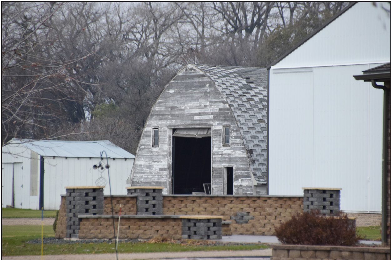
Figure 100. 32RI918, Feature 4, south and east elevations, view facing northwest.
