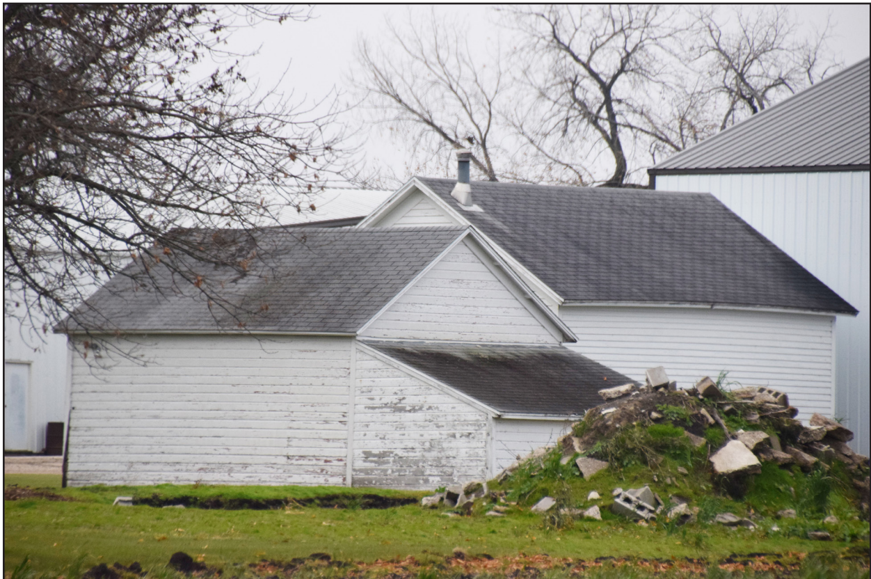
Figure 98. 32RI918, Feature 2 and Feature 3, north and east elevations, view facing southwest.
