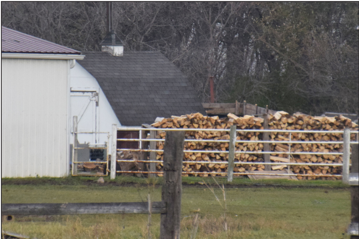
Figure 94. 32RI917, Feature 8, south and east elevations, view facing northwest.
