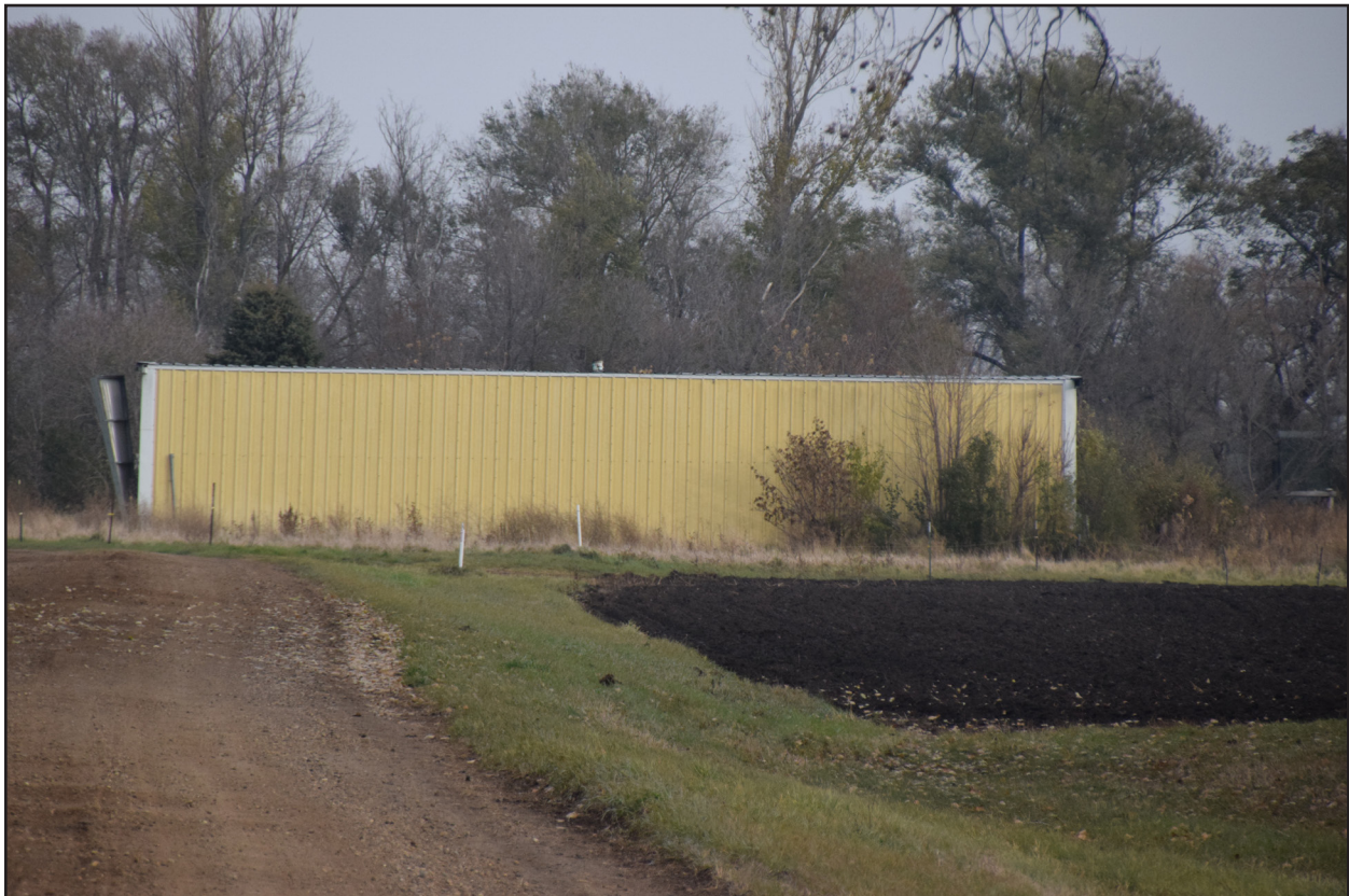
Figure 90. 32RI917, Feature 4, south elevation, view facing north.
