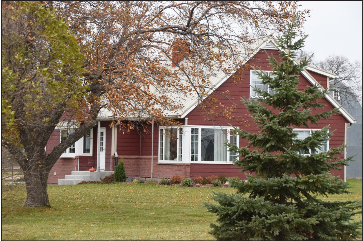
Figure 106. 32RI919, Feature 1, east and south elevations, view facing northwest.
