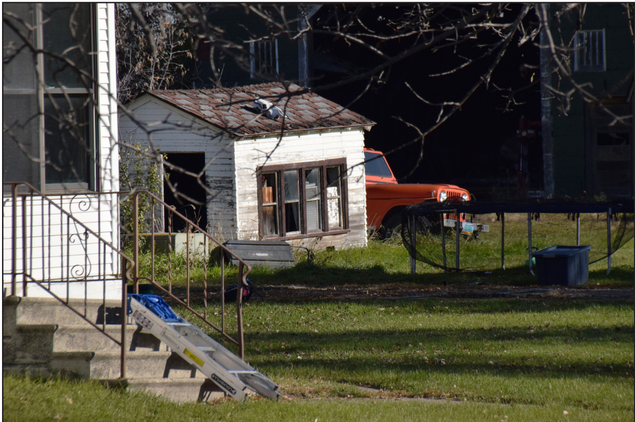
Figure 81. 32RI916, Feature 2, south and west elevations, view facing northeast.
