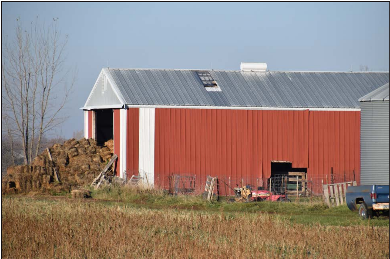
Figure 44. 32CS5357, Feature 2, east and south elevations, view facing northwest.
