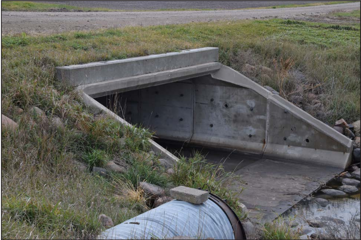
Figure 62. 32RI814, west opening, view facing southeast.
