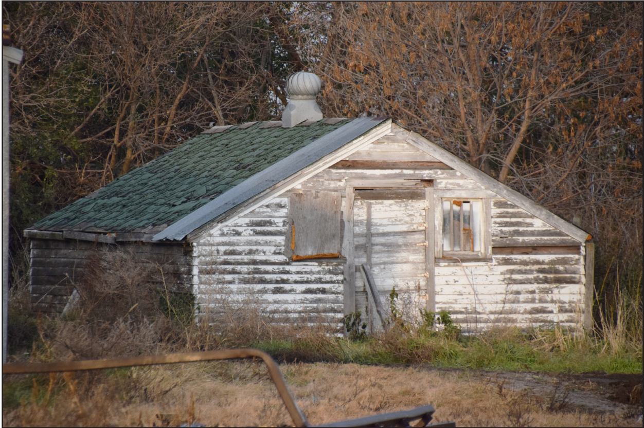
Figure 73. 32RI915, Feature 9, east and south elevations, view facing slightly northwest.
