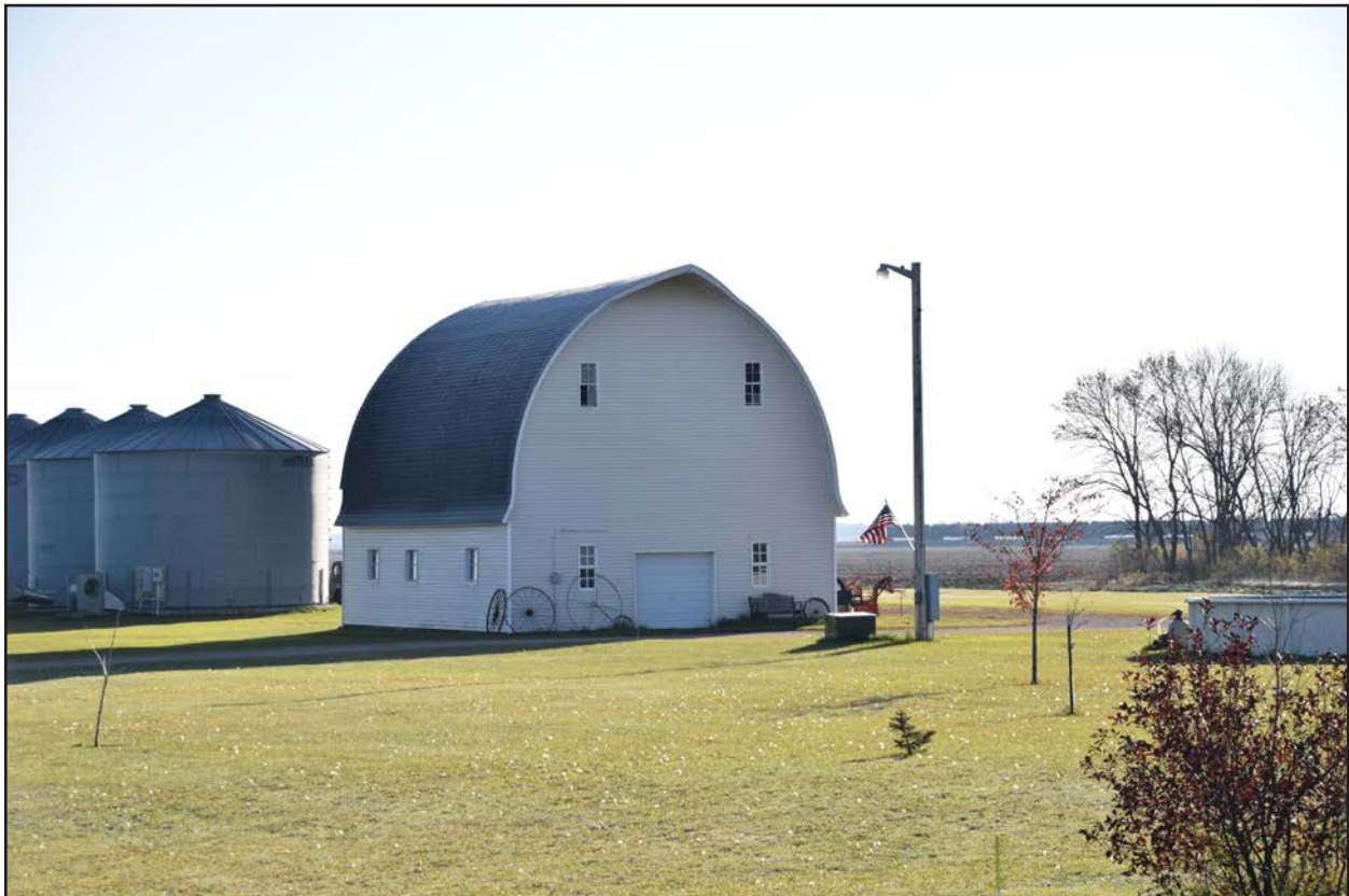
Figure 20. 32CS5354, Feature 2, barn, north and west elevations, view to the southeast.
