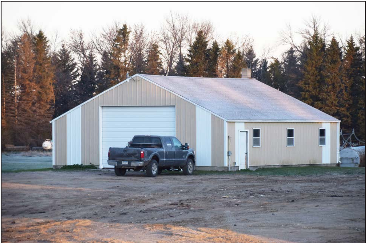
Figure 9. 32CS5284, Feature 3, south and east elevations, view to the northwest.
