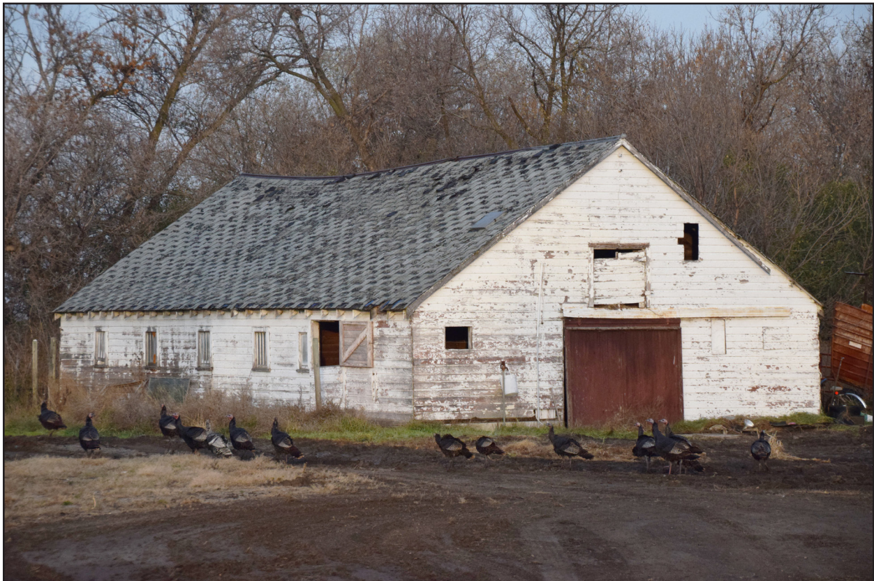
Figure 74. 32RI915, Feature 10, east and south elevations, view facing slightly northwest.
