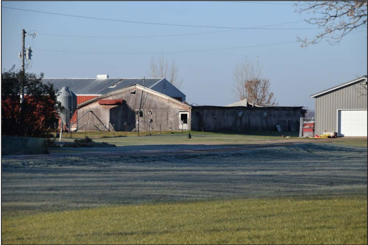
Figure 45. 32CS5357, Feature 3, north and east elevations, view facing southwest.
