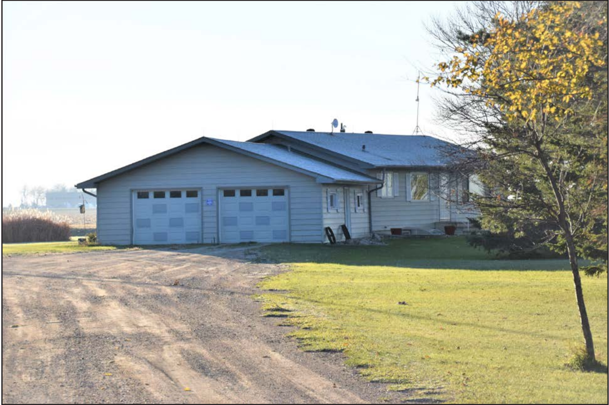
Figure 15. 32CS5353, Feature 1, north and west elevations, view to the southeast.
