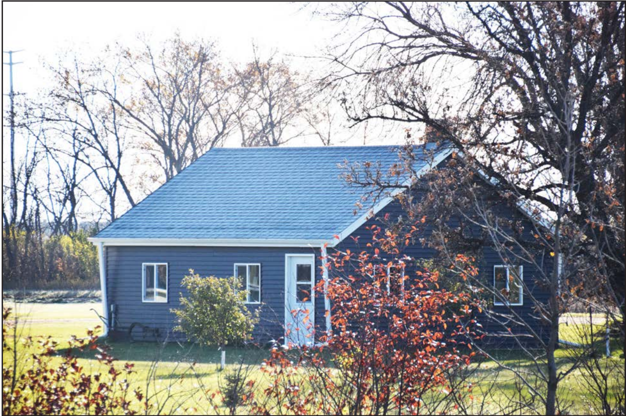
Figure 19. 32CS5354, Feature 1, north and west elevations, view to the southeast.
