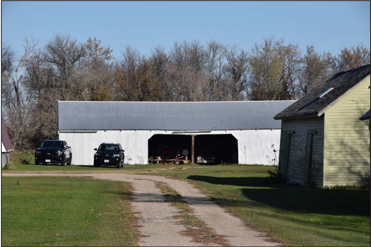
Figure 31. 32CS5355, Feature 7, south elevation, view facing north.
