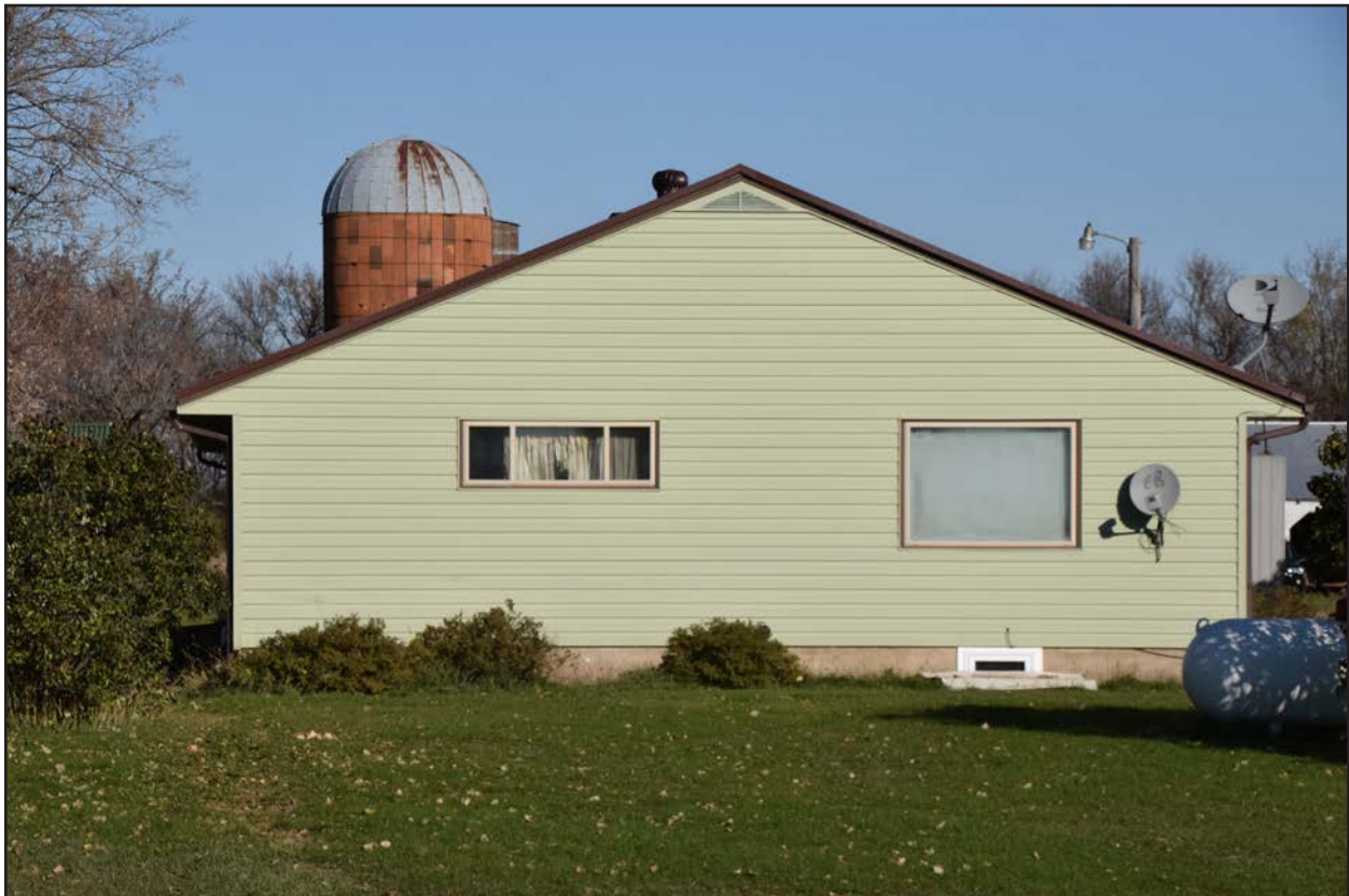
Figure 26. 32CS5355, Feature 1, Linear Ranch dwelling, south elevation, view facing north.
