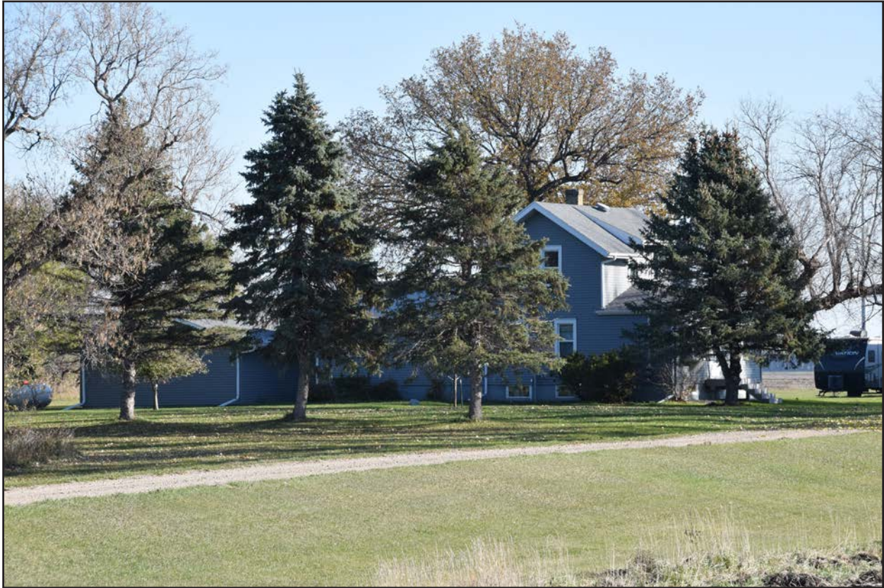
Figure 37. 32CS5356, Feature 1, west and south elevations, view facing northwest.
