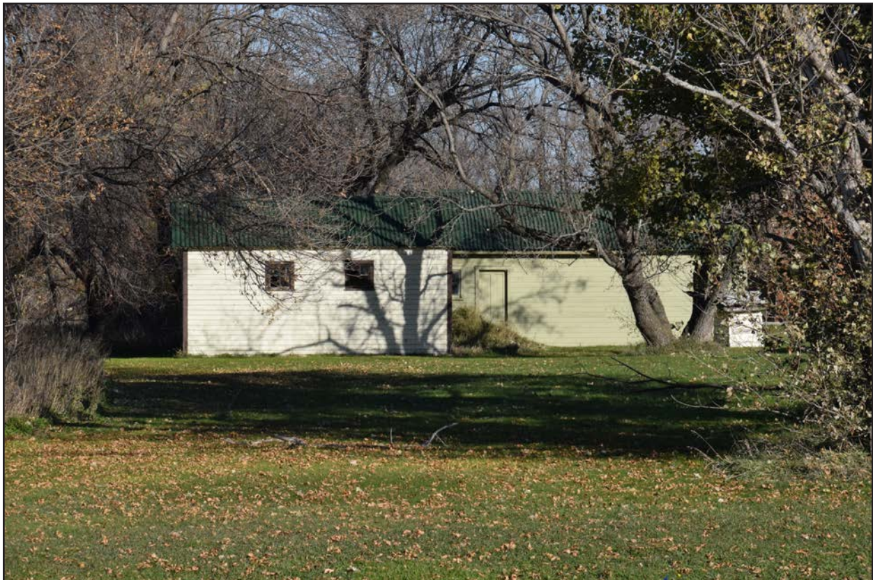
Figure 28. 32CS5355, (from left to right) Features 3, 4, 12, view facing north.
