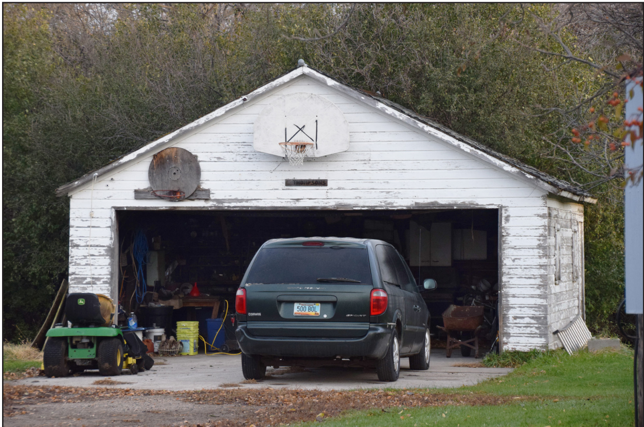
Figure 76. 32RI915, Feature 12, south and east elevations, view facing slightly northwest.
