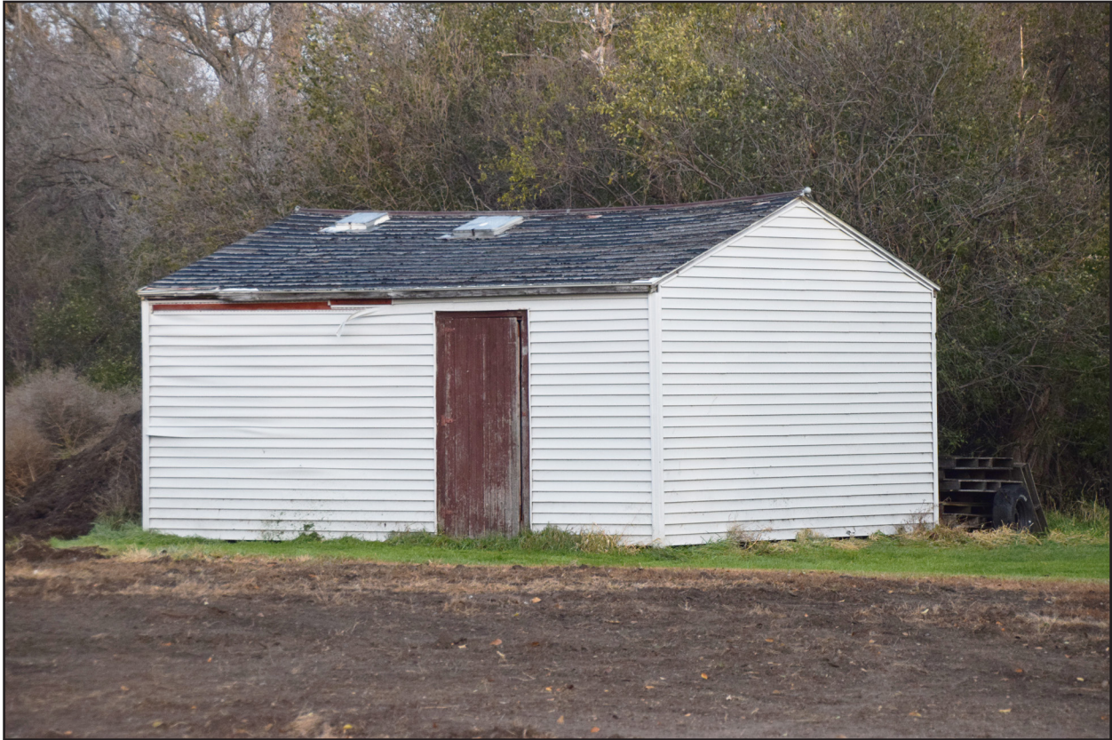
Figure 75. 32RI915, Feature 11, south and east elevations, view facing northwest.
