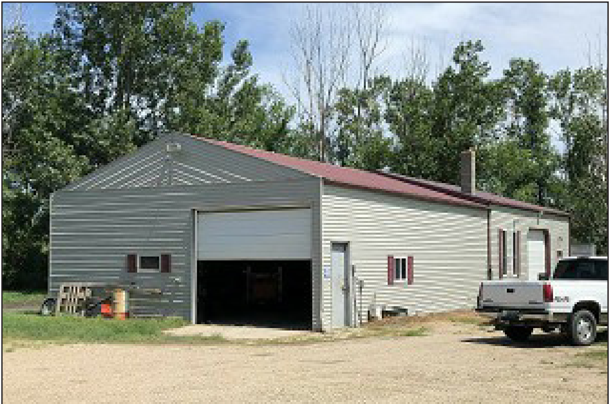
Figure 16. 32CS5353, Feature 2, west and south elevations, view to the northeast.
