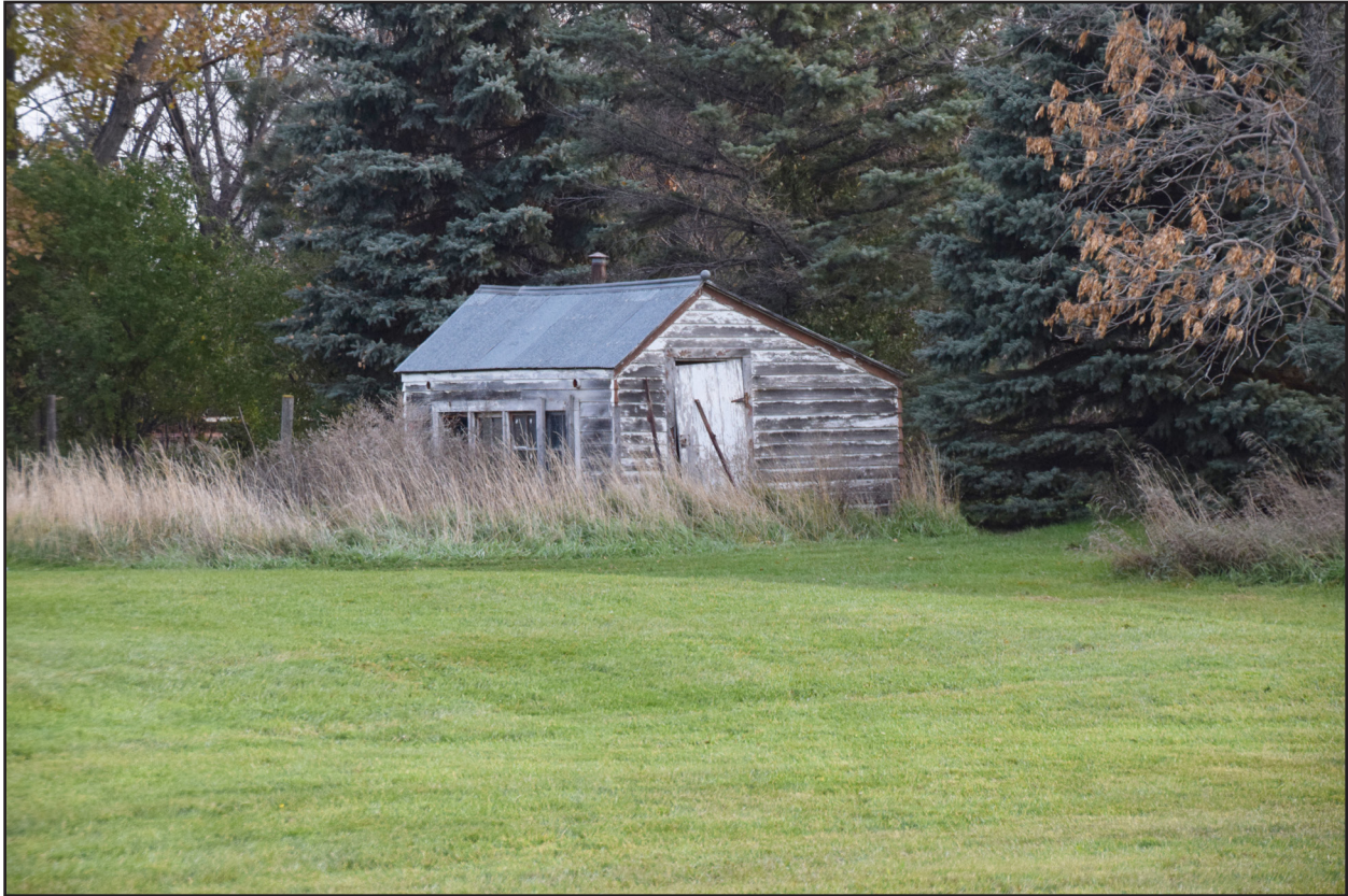
Figure 67. 32RI915, Feature 3, south and west elevations, view facing northeast.
