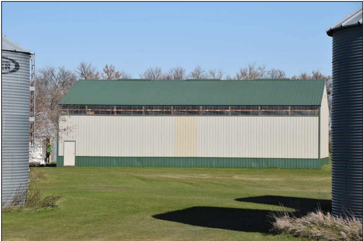
Figure 34. 32CS5355, Modern barn, south elevation, view facing north.
