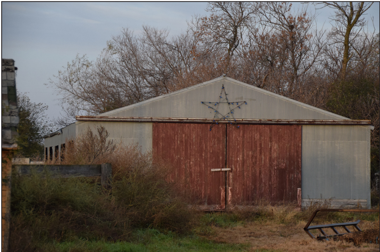
Figure 72. 32RI915, Feature 8, east and south elevations, view facing slightly northwest.
