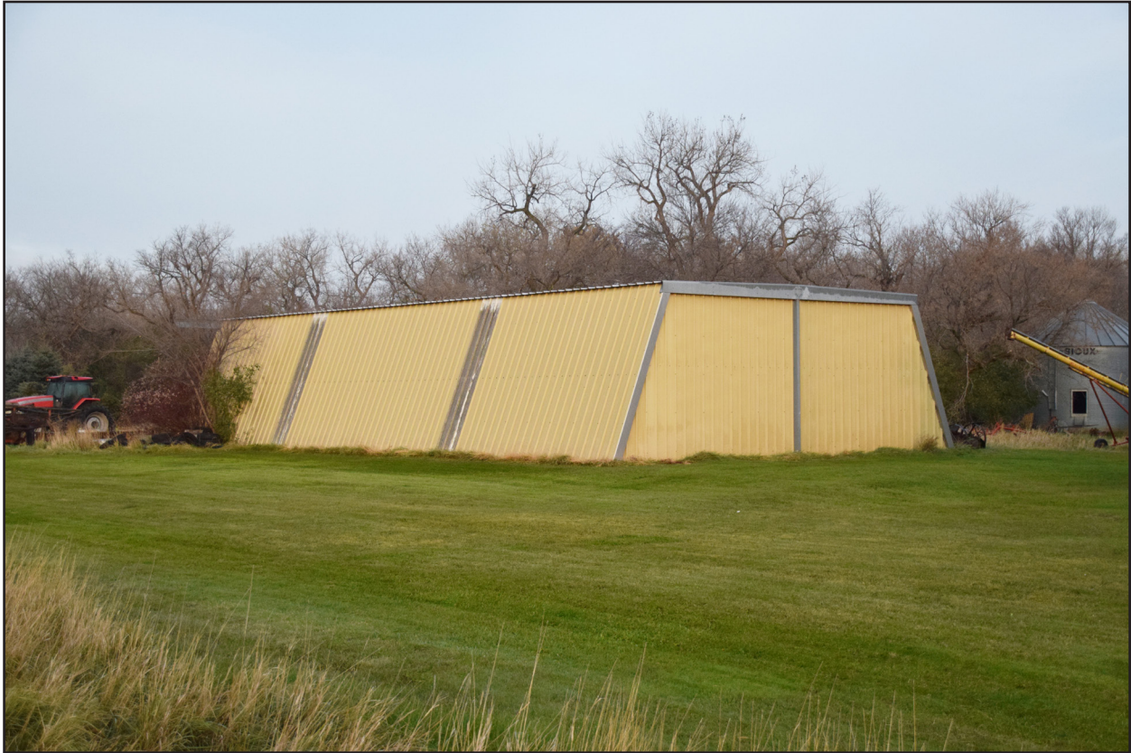
Figure 69. 32RI915, Feature 5, south and east elevations, view facing northwest.
