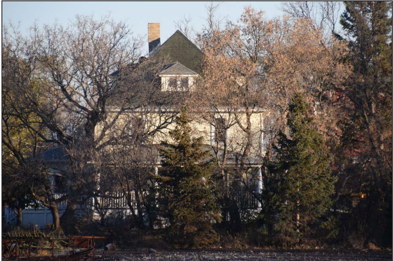
Figure 2. 32CS5119, American Foursquare dwelling, south elevation.
