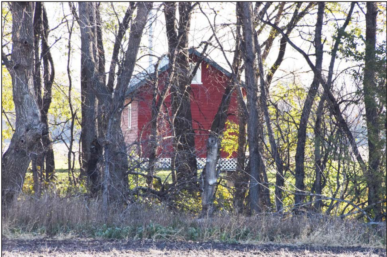
Figure 38. 32CS5356, Feature 2, west elevation, view facing east.
