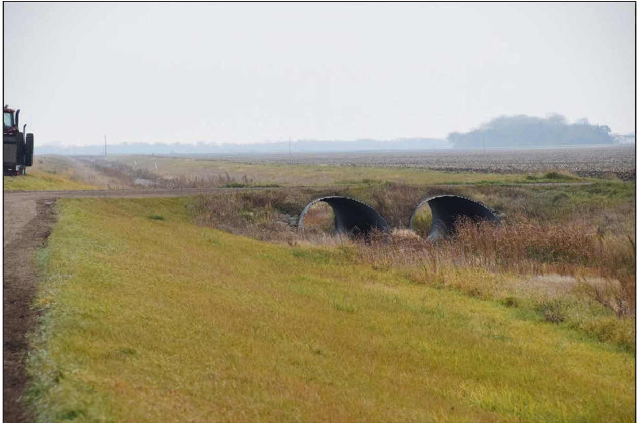
Figure 60. 32RI813, west openings, view facing east-southeast.
