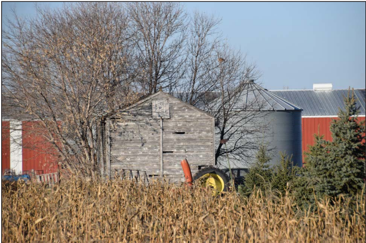
Figure 46. 32CS5357, Features 4 (right) and 5 (left), east elevations, view facing west.
