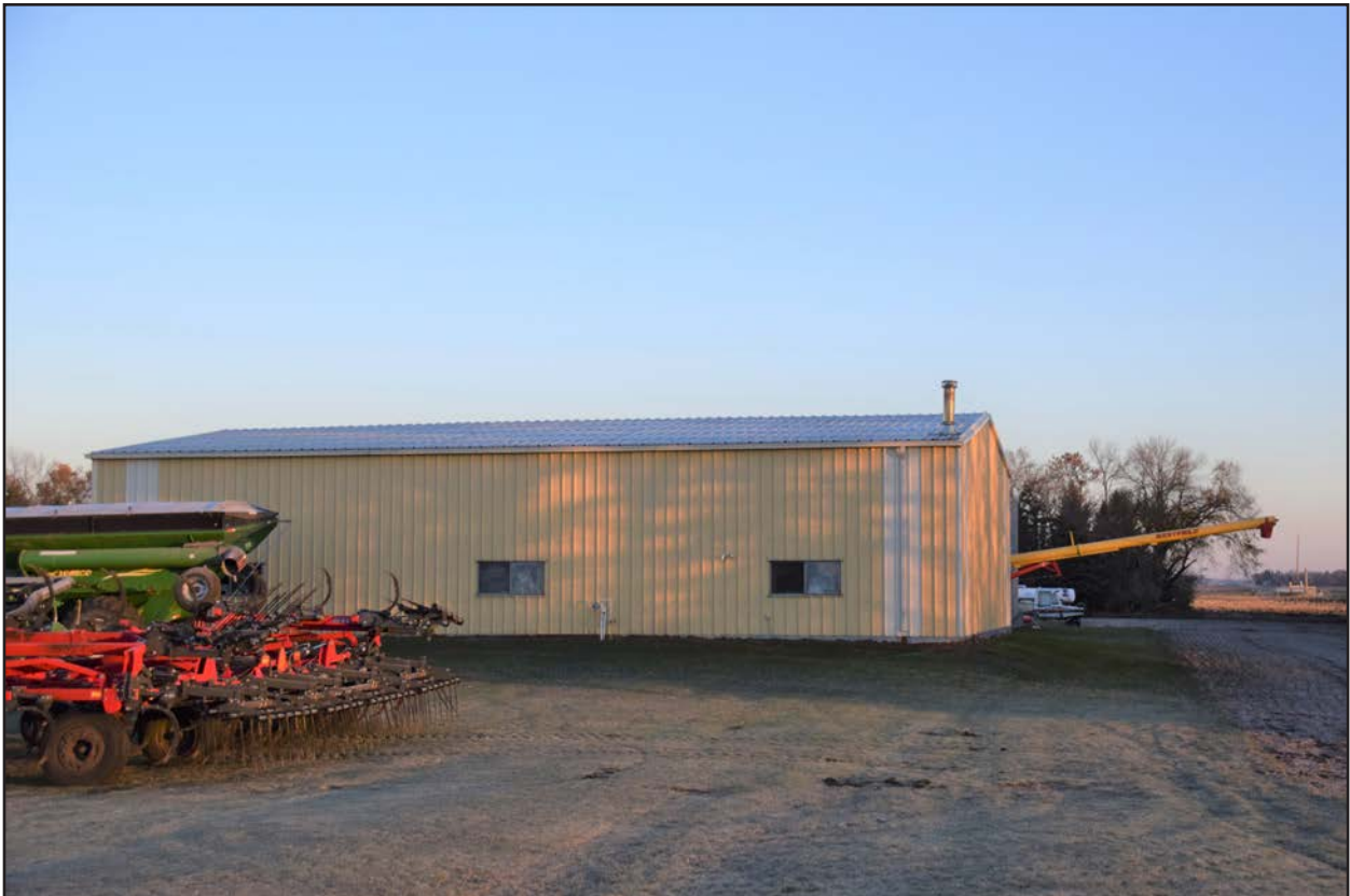
Figure 11. 32CS5284, Feature 5, south and east elevations, view to the northwest.
