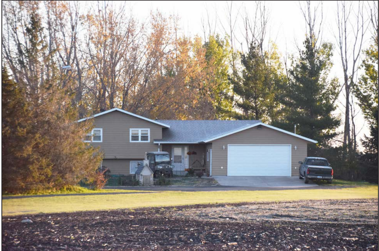
Figure 5. 32CS5283, Feature 1, southwest elevation, view to the northeast.
