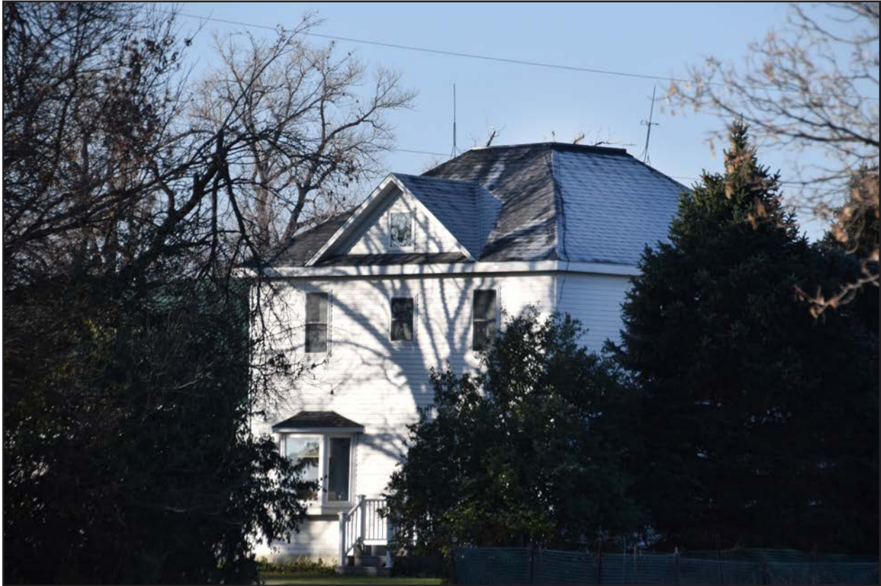
Figure 43. 32CS5357, Feature 1, north and east elevations, view facing southwest.
