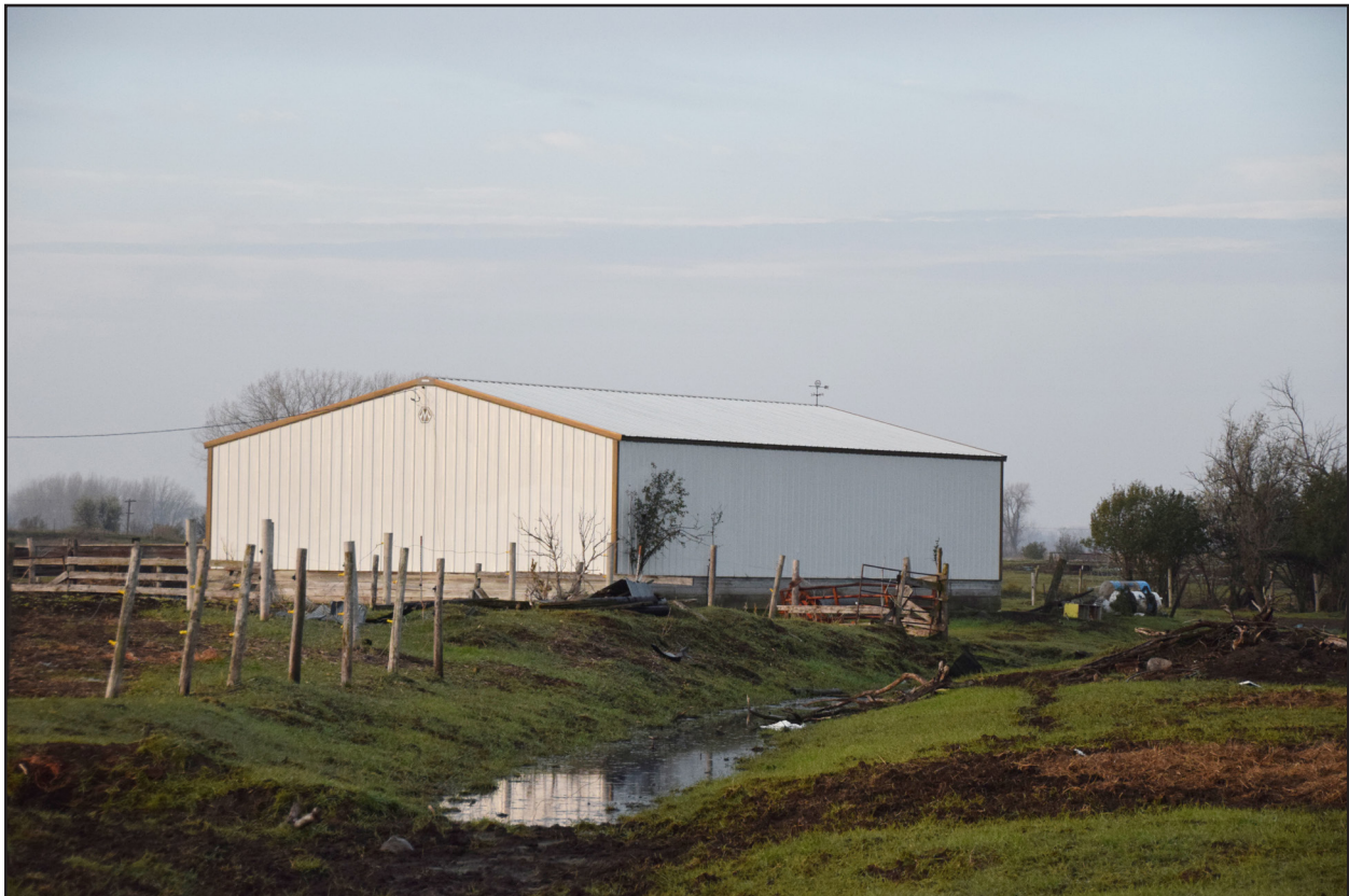
Figure 70. 32RI915, Feature 6, east and north elevations, view facing southwest.
