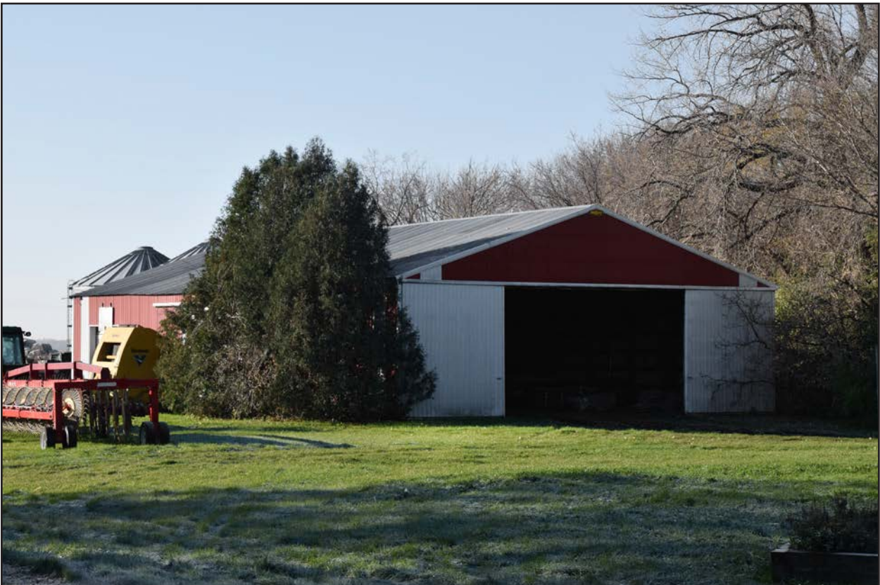
Figure 51. 32CS5358, Feature 3, north and east elevations, view facing southwest.
