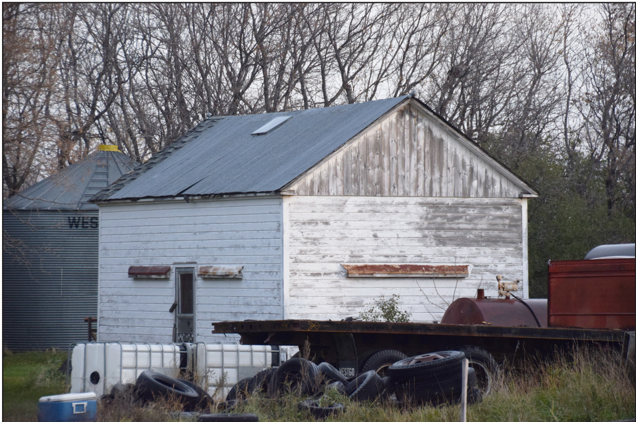
Figure 68. 32RI915, Feature 4, south and west elevations, view facing northeast.
