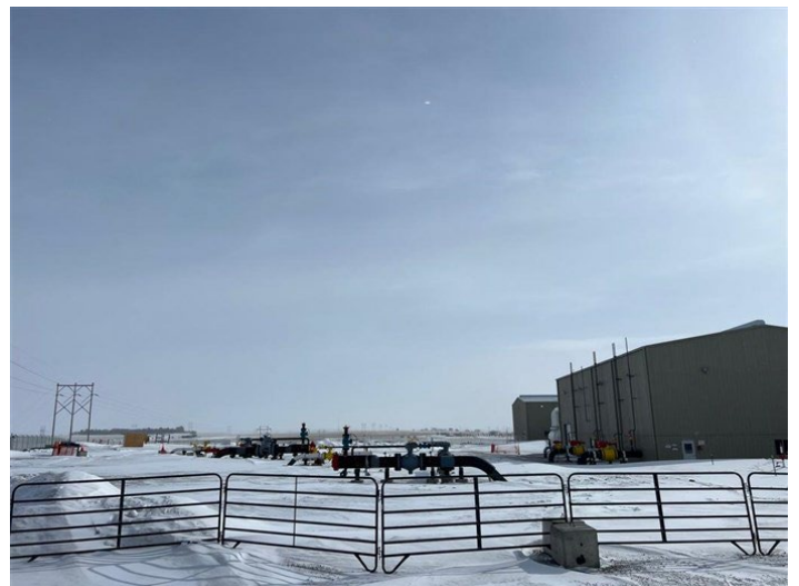
Tioga Compressor Station and Line Section 25 Loop Header – Stable conditions (March 9, 2022) – Acceptable – MP 0
