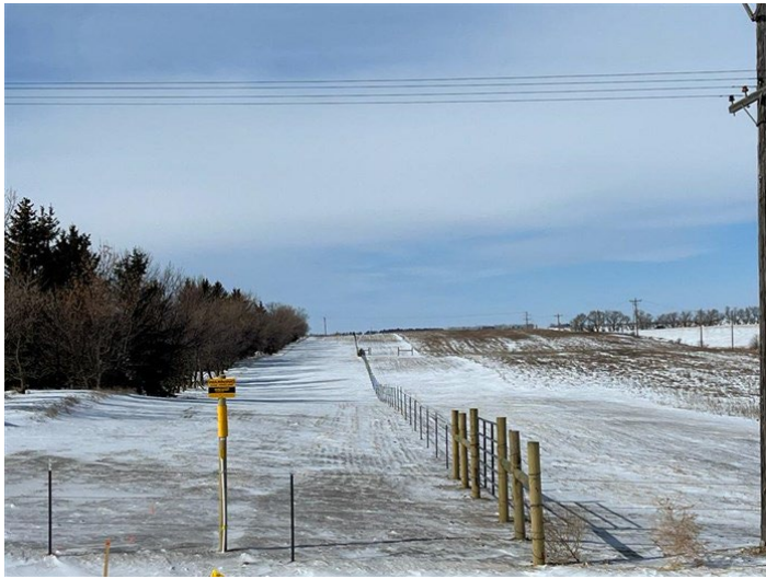
Line Section 30 Loop – Right-of-way stable and fences installed (March 10, 2022) – Acceptable – MP 6.3
