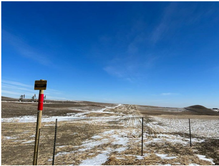
Tioga Elkhorn Creek PL Spread 2 – Right-of-way stable and fences restored (March 7, 2022) – Acceptable – MP 59.8
