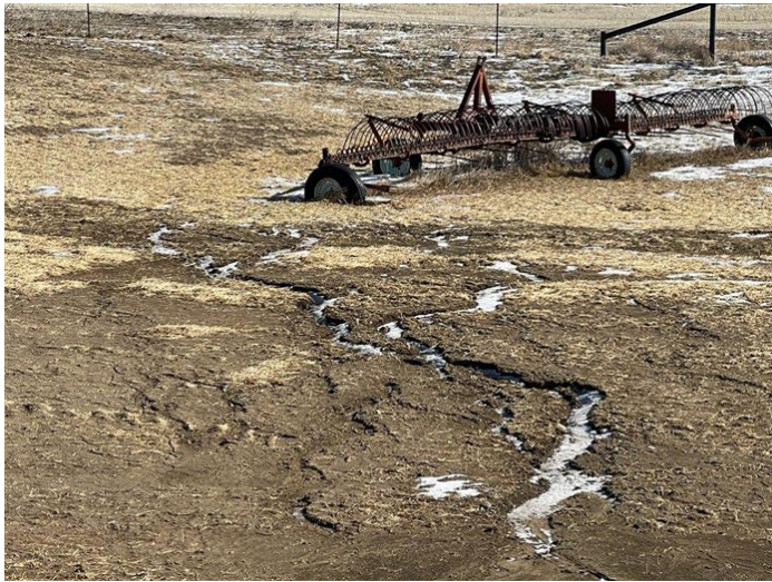
Tioga Elkhorn Creek PL Spread 2 – Minor scouring within the right-of-way near County Road 122 (March 7, 2022) – Acceptable (was already on EI’s punch list for repair when winter weather conditions improve) – MP 58.0
