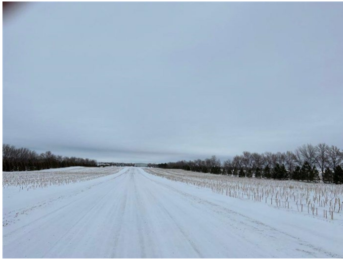
Tioga Elkhorn Creek PL Spread 1 – Private driveway over the new Tioga Elkhorn Creek pipeline (January 26, 2022) – Acceptable – MP 5.3
