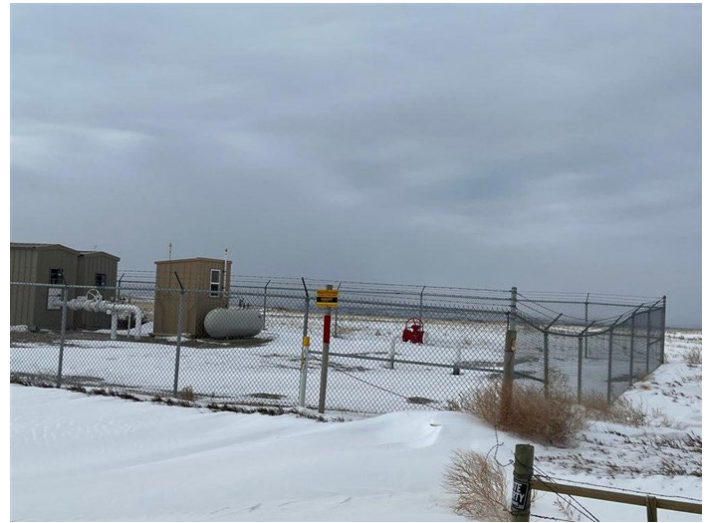
Springbrook Plant Receipt Station – WBI Line Section 30 Loop into the Springbrook Plant Receipt Station (January 18, 2022) – Communication – MP 0.0
