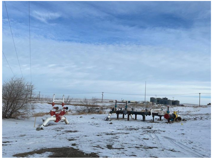
Line Section 30 Loop – Old Temple Valve setting to be removed. New upgrades to the Line Section 30 Loop valves and launcher/receiver. Installation of permanent fences around the new facilities is pending until Spring (January 17, 2022) – Acceptable – MP 0.0
