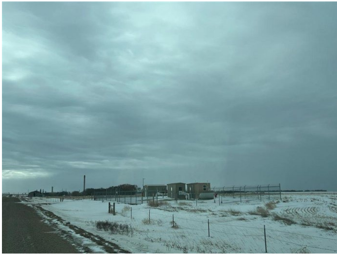
Springbrook Plant Receipt Station – Existing WBI Springbrook Plant Receipt Station in Williams County without any construction upgrades (January 18, 2022) – Communication – MP 0.0
