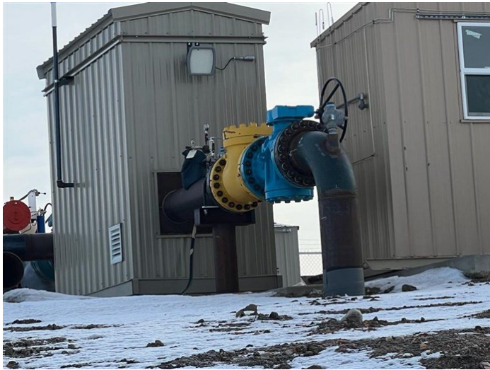
Line Section 30 Loop – Nesson Station updated control valve (January 17, 2022) – Acceptable – MP 0.0
