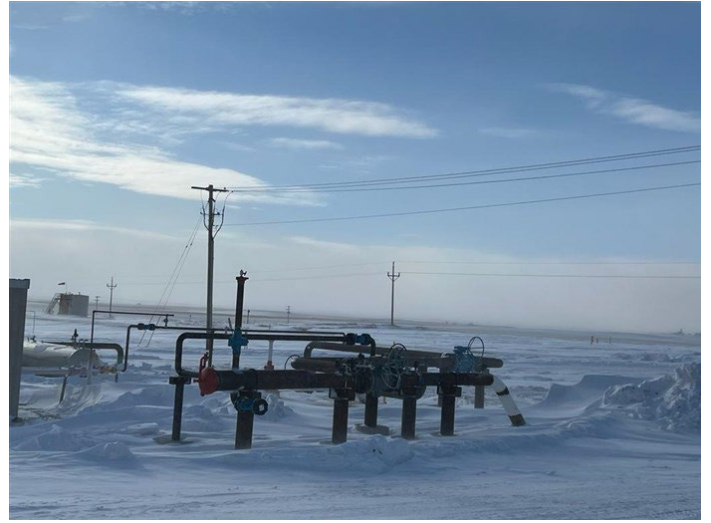
Lignite Plant and Border Stations – New Lignite launcher/receiver (January 5, 2022) – Acceptable – MP 0.0
