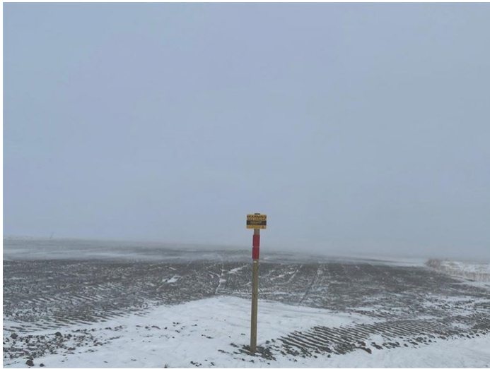
Tioga Elkhorn Creek PL Spread 2 – Line marker over the new Northern Border Interconnect pipeline (January 4, 2022) – Communication – MP 0.1
