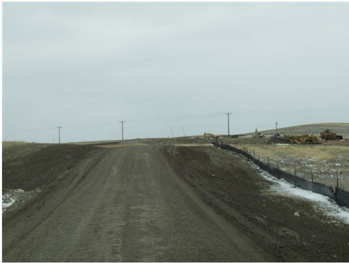
Northern Border Interconnect – Erosion control devices installed on the southern side of the access road leading into the interconnect site (December 13, 2021) – Acceptable – MP 0.3
