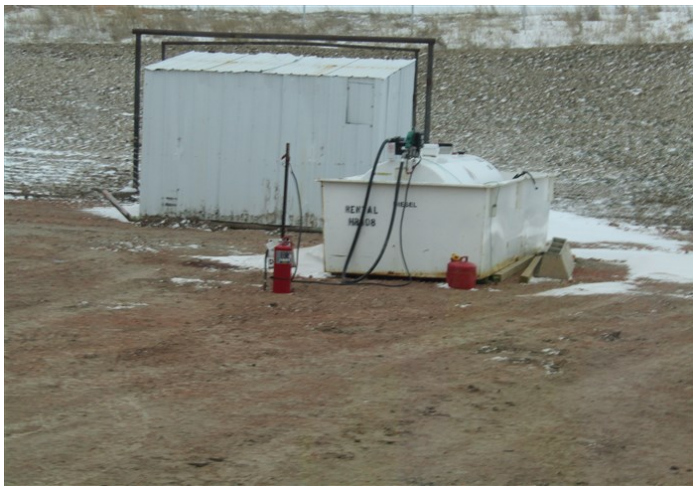
Elkhorn Creek Compressor Station – Fuel storage inside secondary containment with a fire extinguisher on-site (December 10, 2021) – Acceptable – MP 61.7
