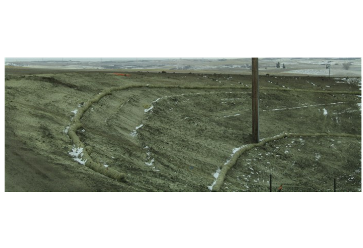
Elkhorn Creek Compressor Station – Erosion control devices installed at the site entrance and sloped area on the south side of the Station (December 10, 2021) – Acceptable – MP 61.7
