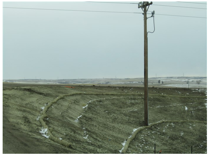
Northern Border Interconnect – Erosion control devices installed at the western bank of the access road entrance to the site (November 17, 2021) – Acceptable – MP 0.3
