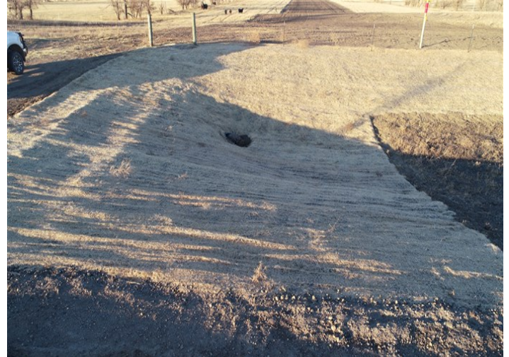
Tioga Elkhorn Creek PL Spread 2 – All construction activities including final clean-up are complete. Curlex was installed at ditch banks along Highway 10 (November 20, 2021) – Acceptable – MP 36.8
