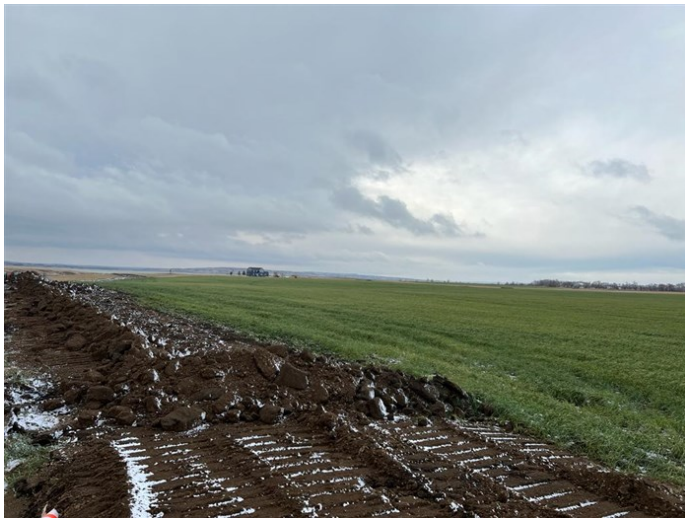
Lake Sakakawea HDD North – In progress removal and restoration of a temporary road that was constructed for landowner access to bypass the HDD site during construction (November 15, 2021) – Acceptable – MP 22.9
