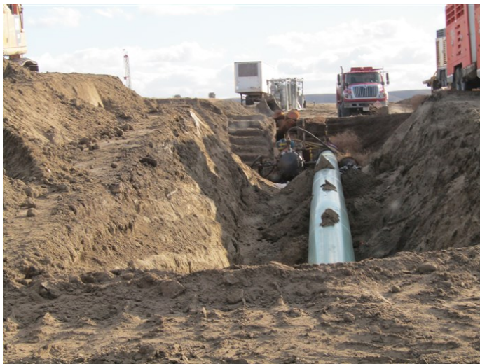
Lake Sakakawea HDD South – Ditch open and crews running pigs and drying lines with heaters after hydro-testing activities were completed (November 16, 2021) – Acceptable – MP 26.0
