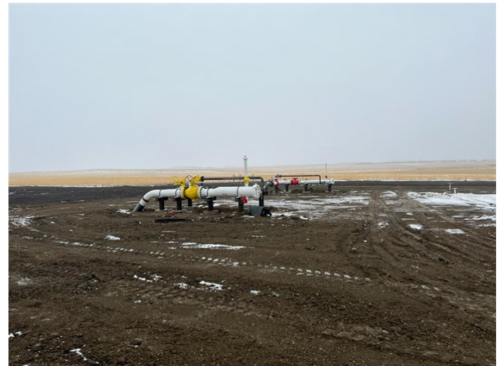
Uprates to Line Section 25 – Finished grade around new pig launcher. Receiver has been restored (November 16, 2021) – Acceptable – MP 0.0
