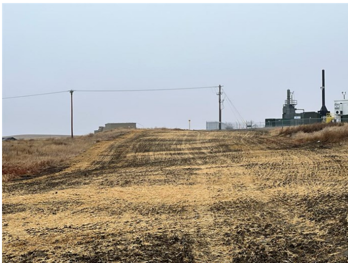
Line Section 30 Loop – Mulched and seeded right-of-way (November 18, 2021) – Acceptable – MP 0.0
