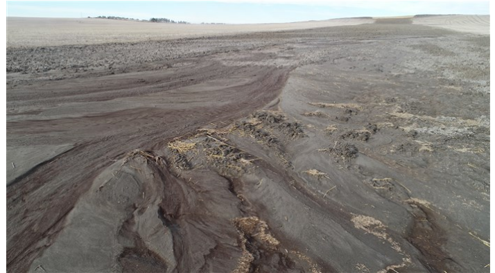
Tioga Elkhorn Creek PL Spread 2 – Right-of-way topsoil erosion and sediment migration occurring. Top of the sloped area of the right-of-way (November 24, 2021) – Communication – MP 44.4
