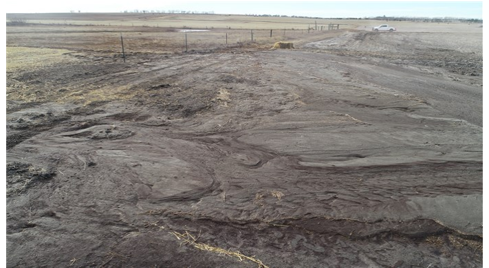
Tioga Elkhorn Creek PL Spread 2 – Topsoil erosion occurring (November 24, 2021) – Communication – MP 44.4
