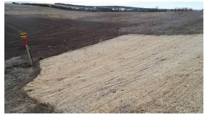
Tioga Elkhorn Creek PL Spread 2 – Curlex installed on the south side of Highway 12 at the downslope area of the road shoulder (November 23, 2021) – Acceptable – MP 43.5
