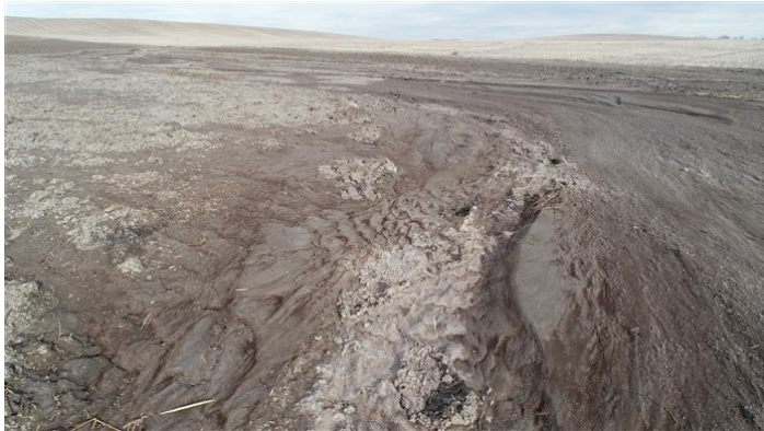
Tioga Elkhorn Creek PL Spread 2 – Flow of the sediment from the right-of-way (November 24, 2021) – Communication – MP 44.4
