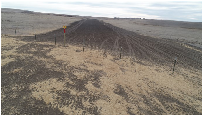
Tioga Elkhorn Creek PL Spread 2 – Final clean-up completed on this area of the right-of-way. Wetland w-mk-eb-003e and contours restored (November 23, 2021) – Acceptable – MP 41.1
