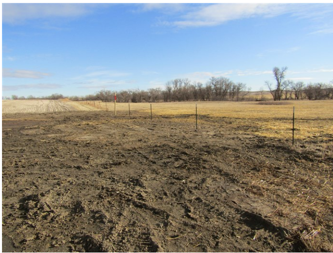
Tioga Elkhorn Creek PL Spread 2 – Eastern side of the right-of-way where the sediment was pulled back onto the right-of-way (November 27, 2021) – Acceptable – MP 44.4
