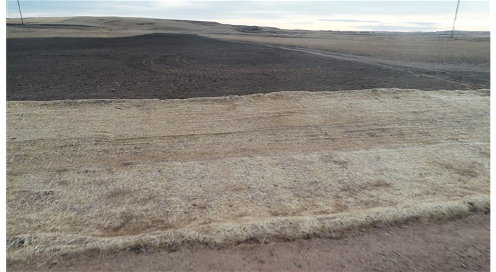
Tioga Elkhorn Creek PL Spread 2 – Curlex installed on both sides of 38 th Street NW (November 22, 2021) – Acceptable – MP 39.2
