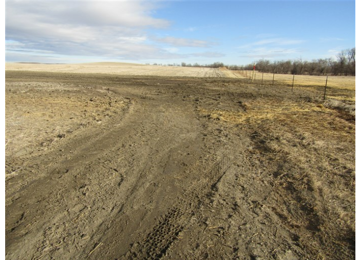
Tioga Elkhorn Creek PL Spread 2 – Field road to where sediment migrated. The sediment was cleaned up and pulled back onto the right-of-way (November 27, 2021) – Acceptable – MP 44.4
