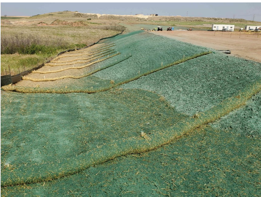
Date: 7/30/2021 Direction: East Notes: Hydro seeding and erosion control device installation.
