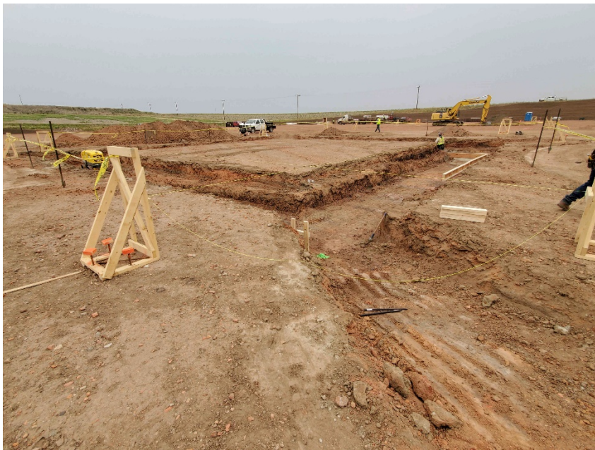
Date: 7/27/2021 Direction: Southeast Notes: Foundation excavation.
