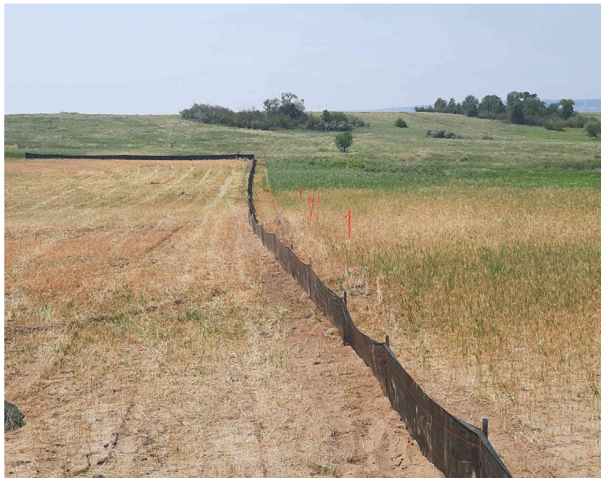
Date: 7/26/2021 Notes: Erosion control device installation on northern edge of HDD workspace looking west.
