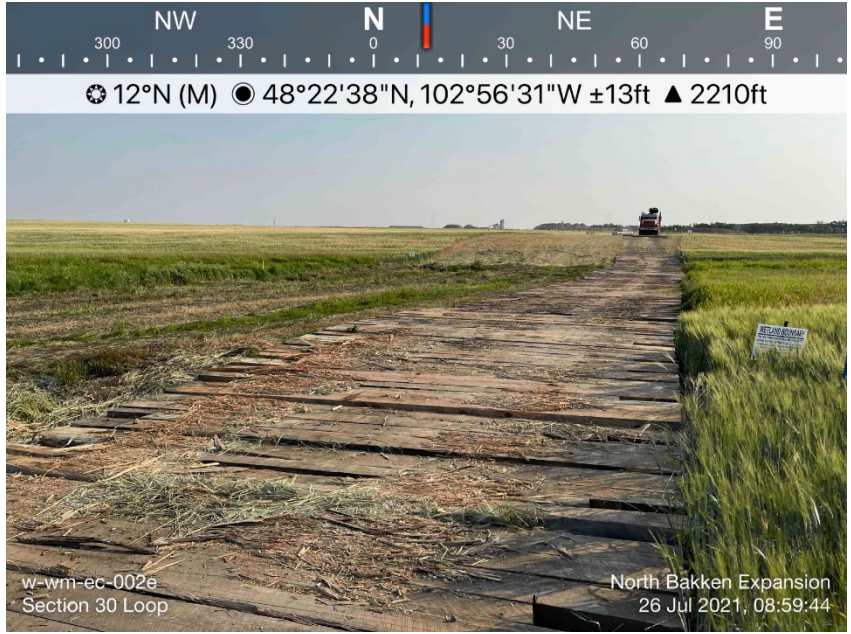
Date: 7/26/2021 Location: Sta. No.: 300+62 Notes: Mat installation at wetland w-wm-ec-002e
