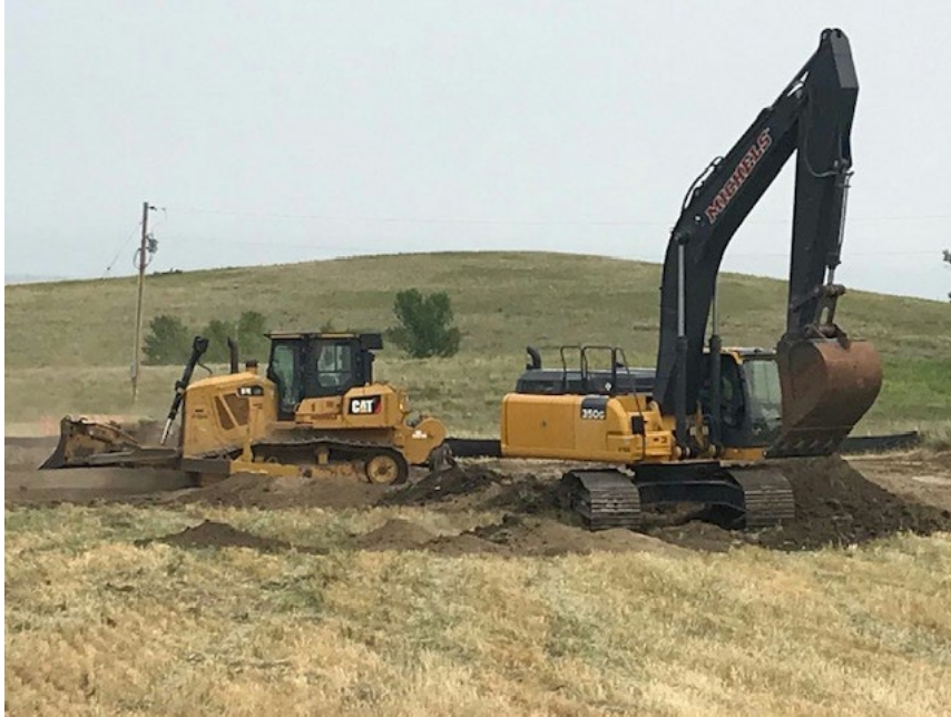
Date: 7/27/2021 Notes: Topsoil stripping.
