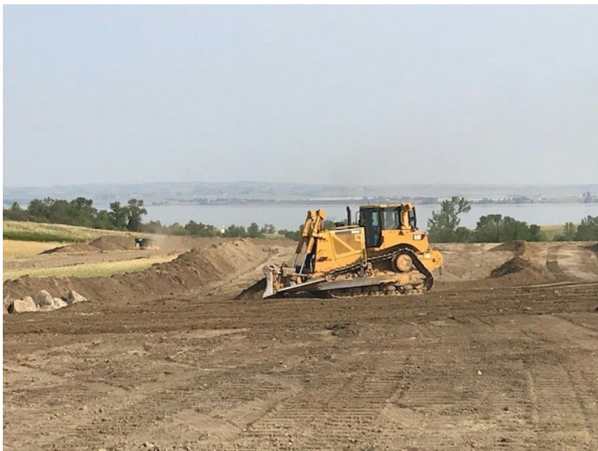
Date: 7/30/2021 Notes: Clearing/Grading activities.
