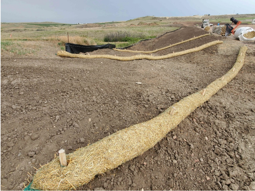
Date: 7/29/2021 Direction: East Notes: Erosion control device installation.
