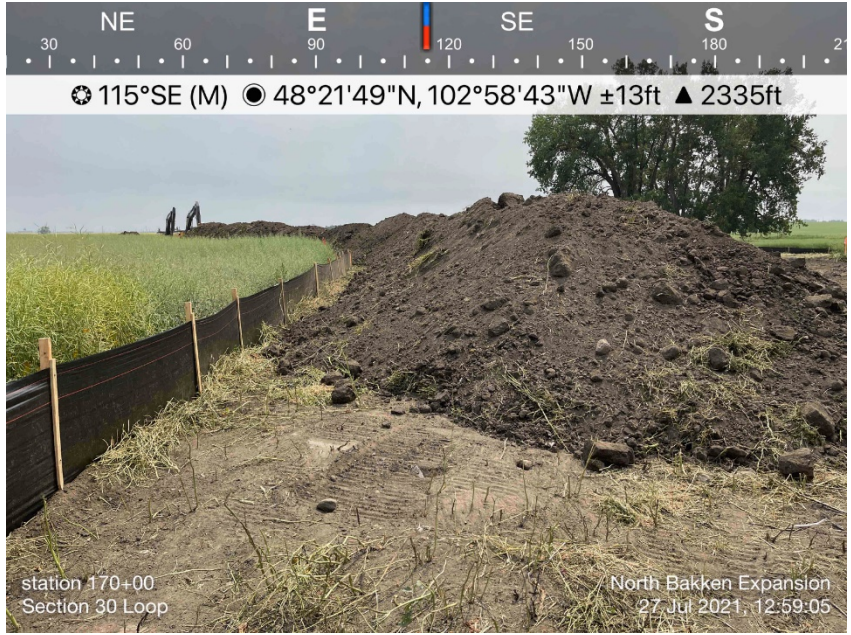
Date: 7/27/2021 Location: 170+00 Notes: Topsoil stockpiled inside of erosion control devices.
