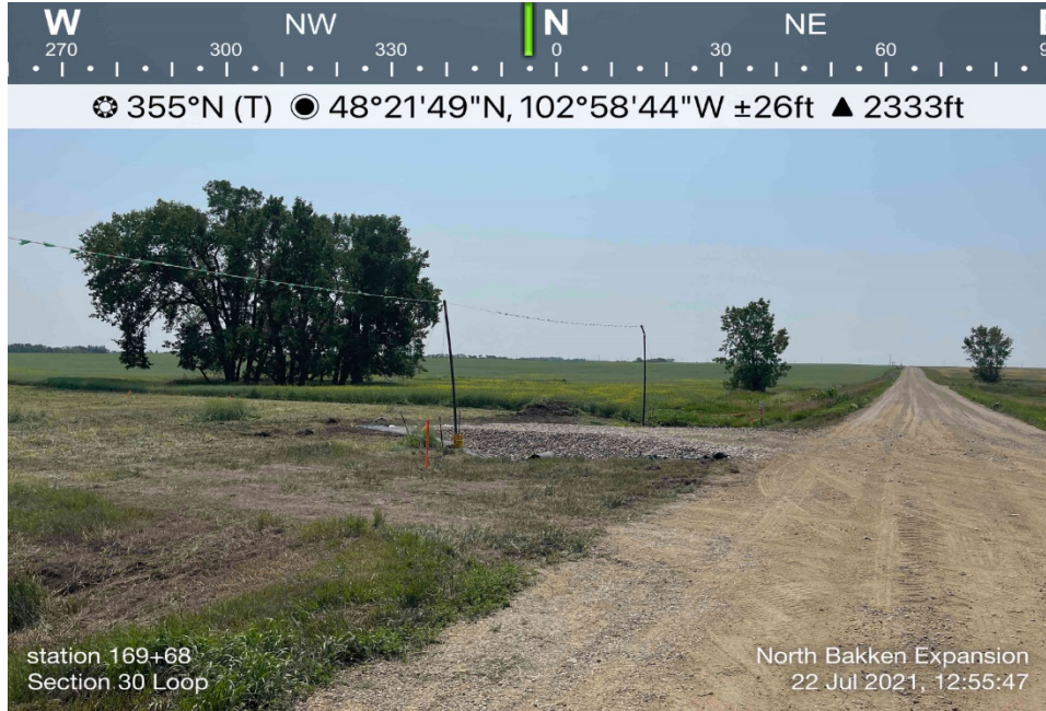
Road approach installed on the west side of 106 th Avenue along the Line Section 30 Loop.
