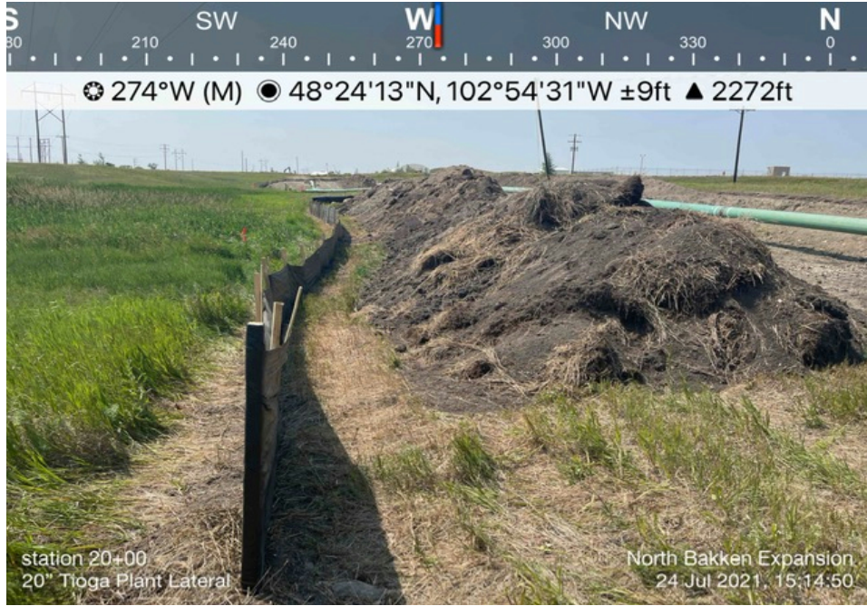
Stockpiled topsoil within the right-of-way and silt fence installed along the boundary of the Tioga Plant Lateral.
