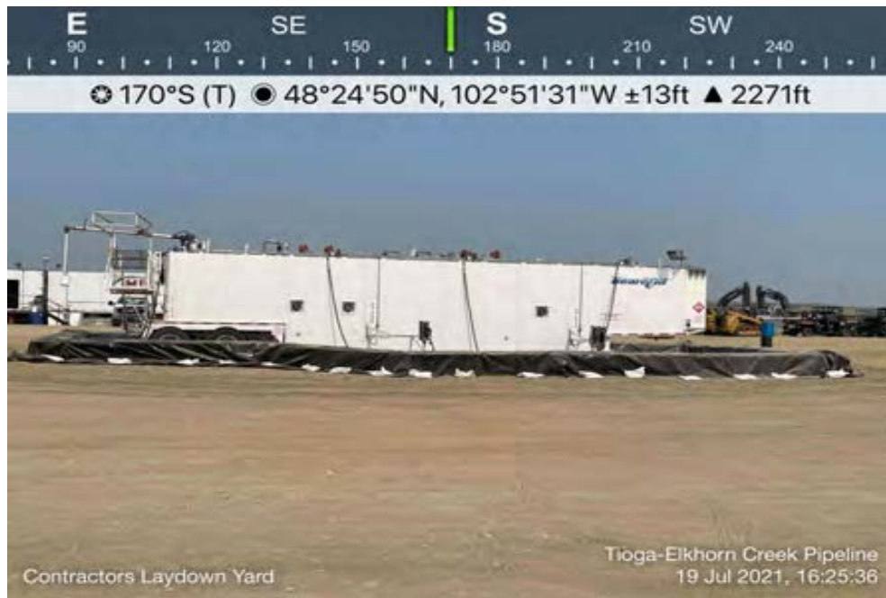
Fuel tank in secondary containment at the 69 th Street Staging Yard near Tioga, ND.
