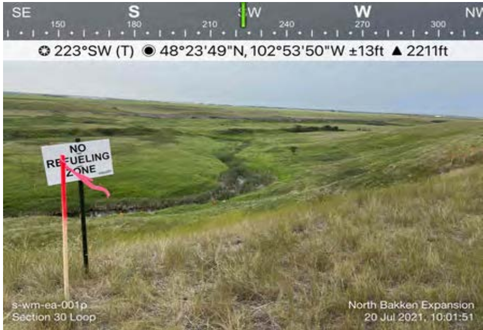
No Refueling sign installed at waterbody s-wm-ea-001p along the Line Section 30 Loop.
