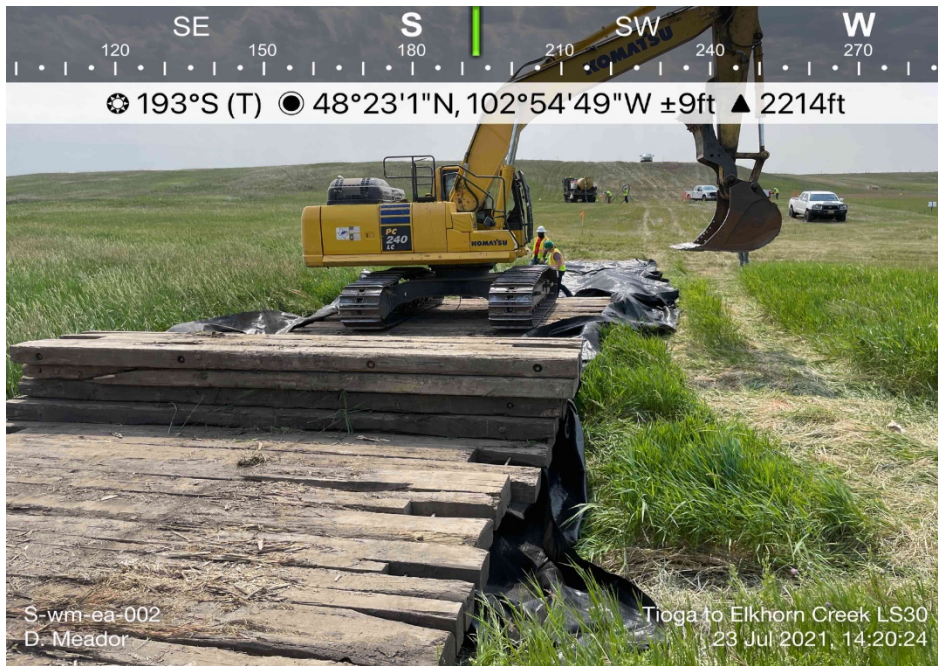
Timber mat bridge being installed at waterbody s-wm-ea-002 along the Line Section 30 Loop.
