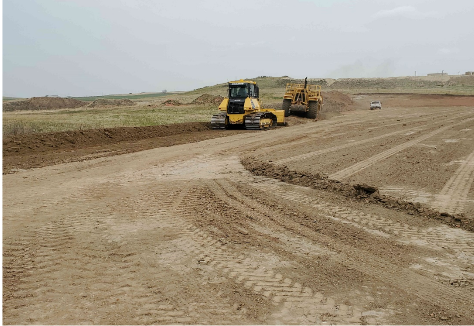
Grading of berm on the north side of the graded pad at the Elkhorn Creek Compressor Station.
