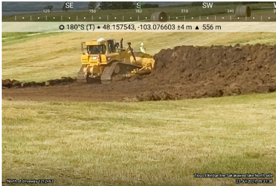
Stripping topsoil for HDD pad on the north side of Lake Sakakawea.
