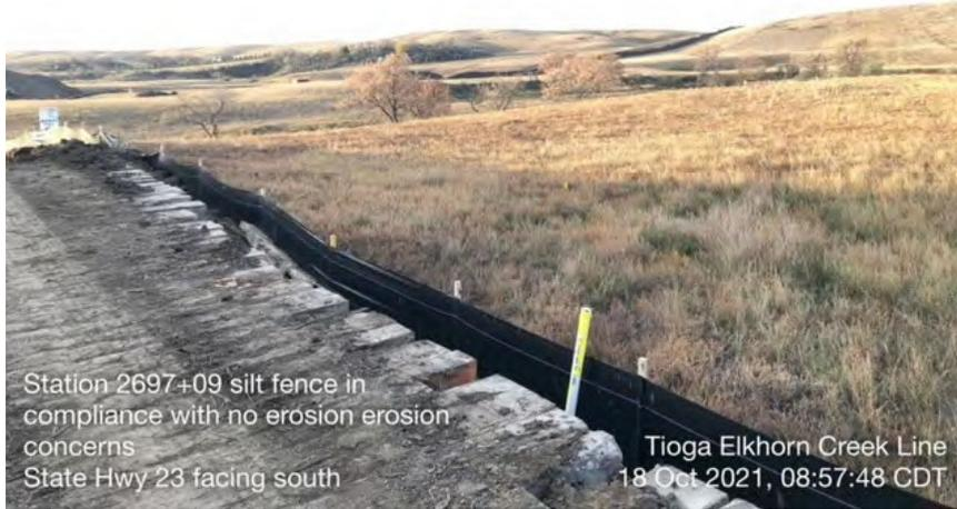
Station 2697+09 silt fence in compliance with no erosion concerns
