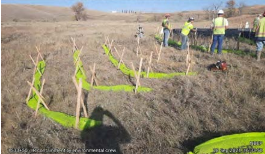
1533+50 - IR containment by environmental crew
