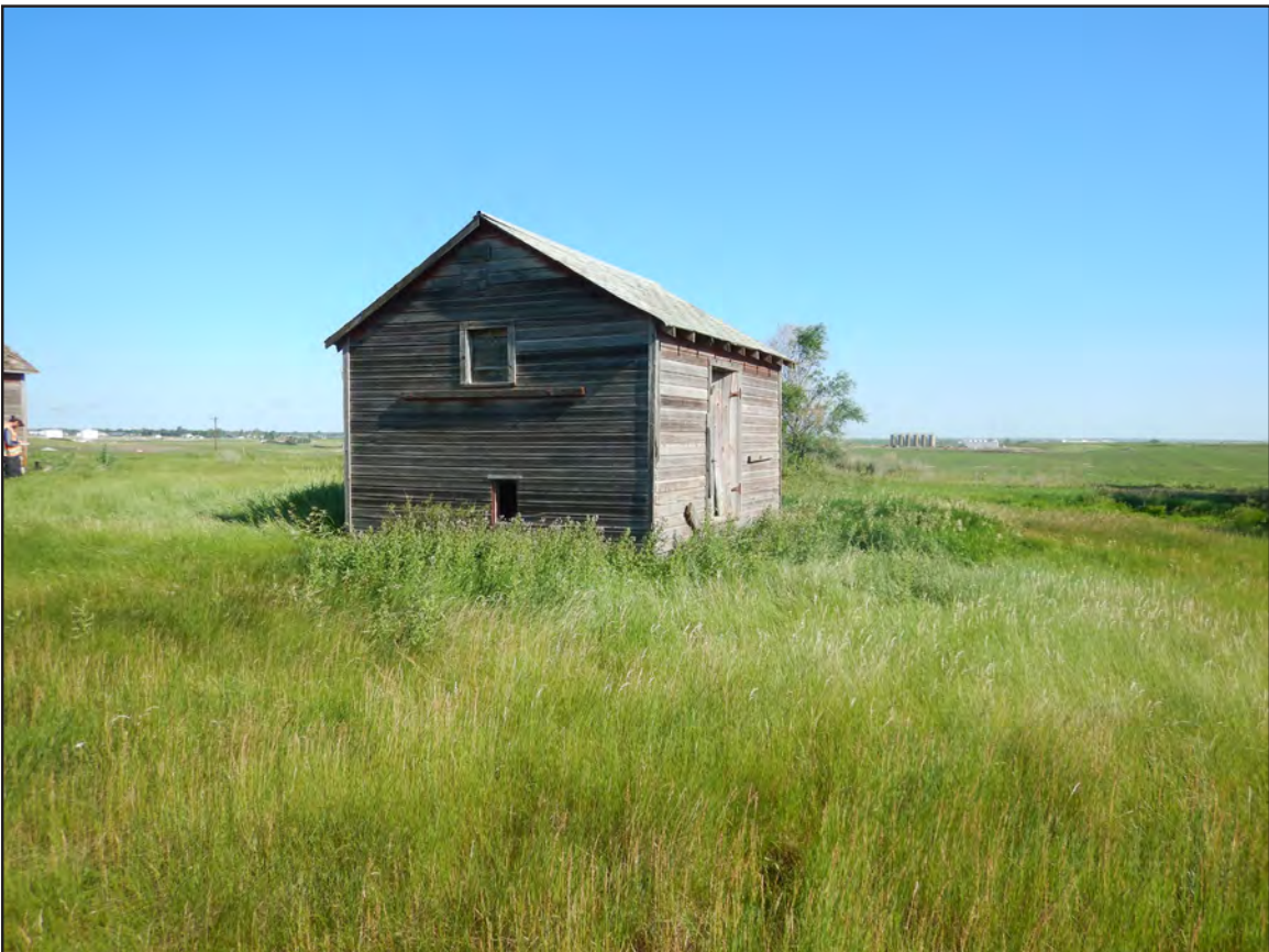
Figure 5. 32MN1338, Feature 3, south and east elevations, view to the northwest.
