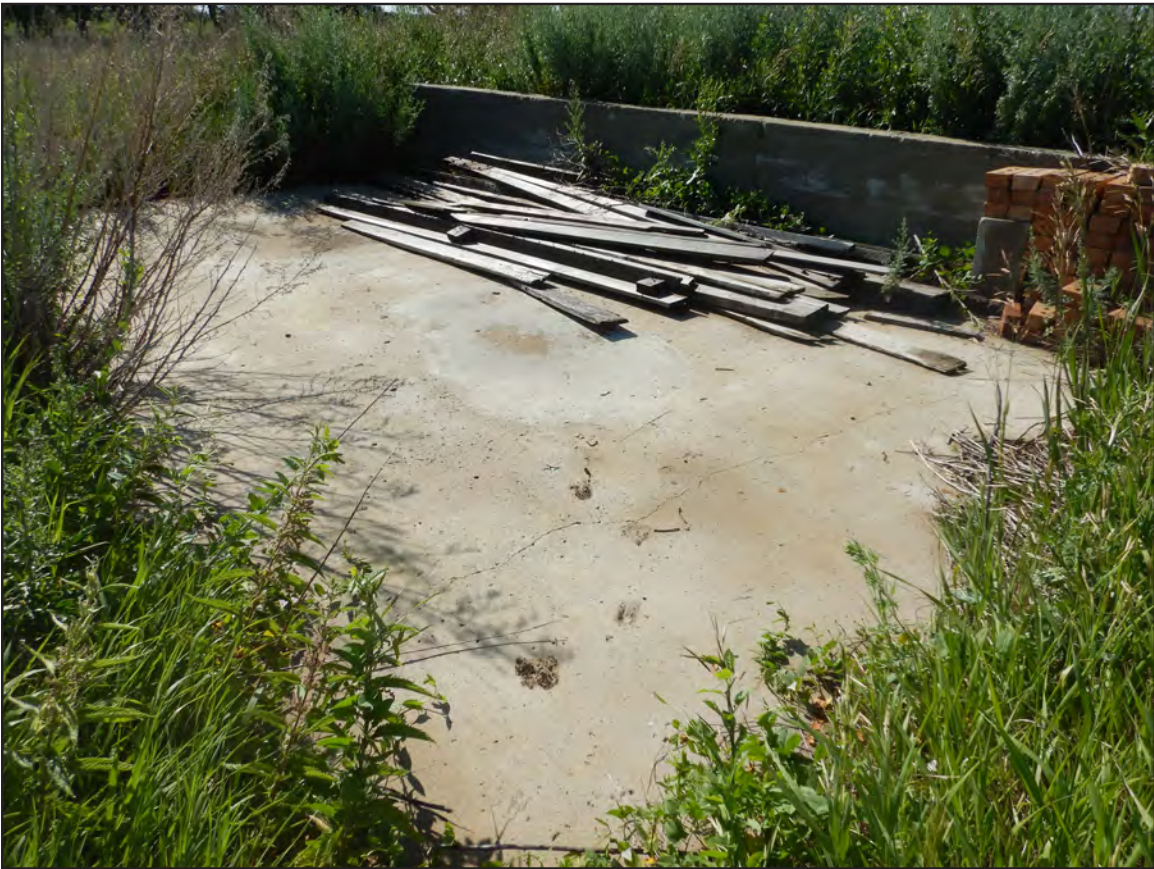
Figure 2. 32MN1338, Feature 1, concrete foundation remains, view to the south.
