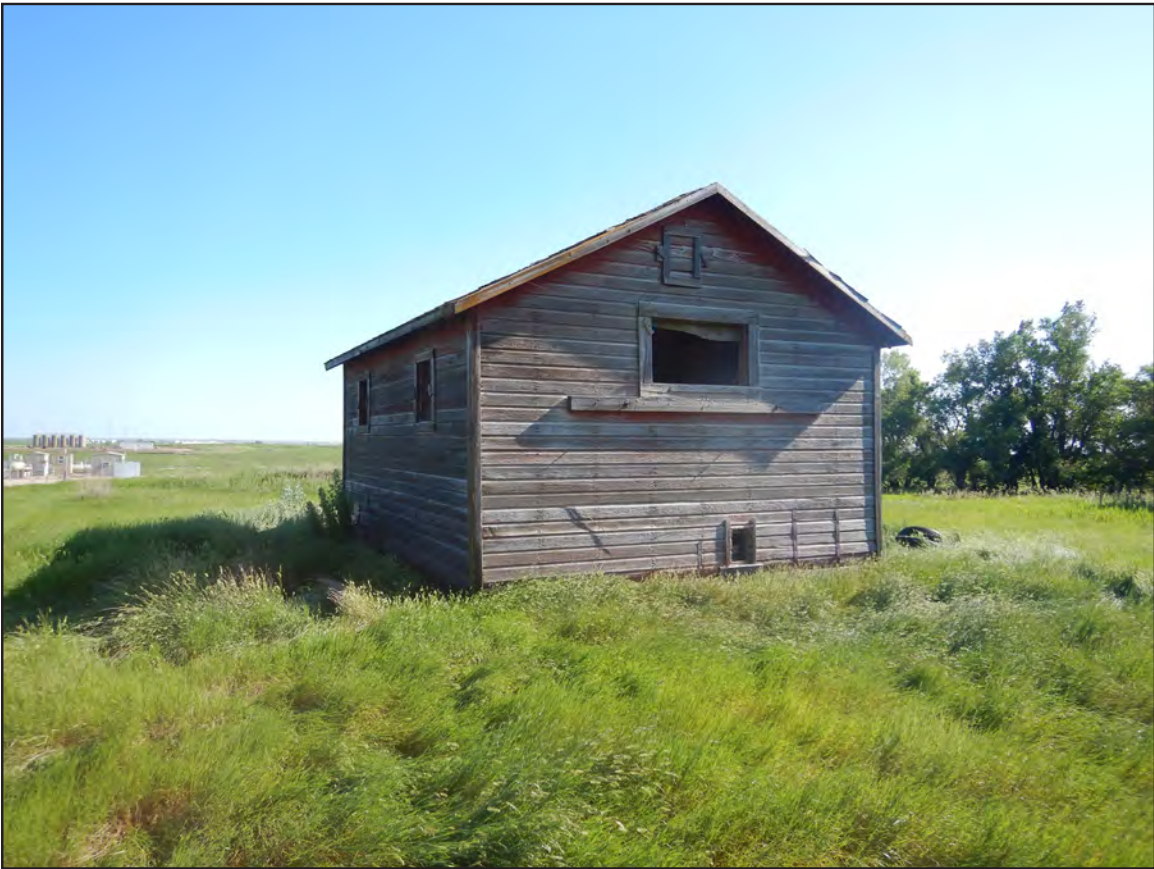
Figure 4. 32MN1338, Feature 2, south and west elevations, view to the northeast
