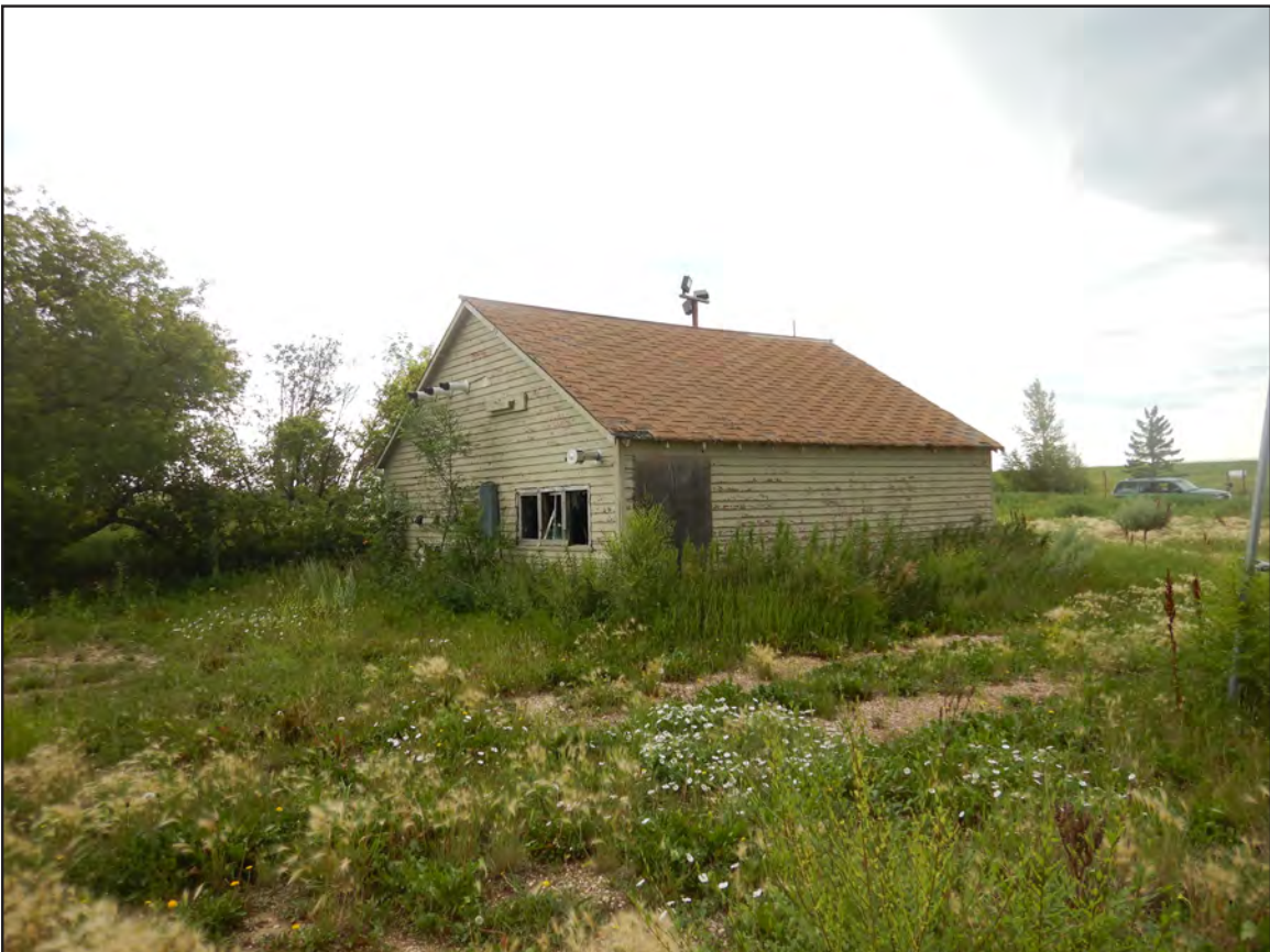
Figure 10. 32WI424, Feature 1, north and west elevations, view to the southeast.
