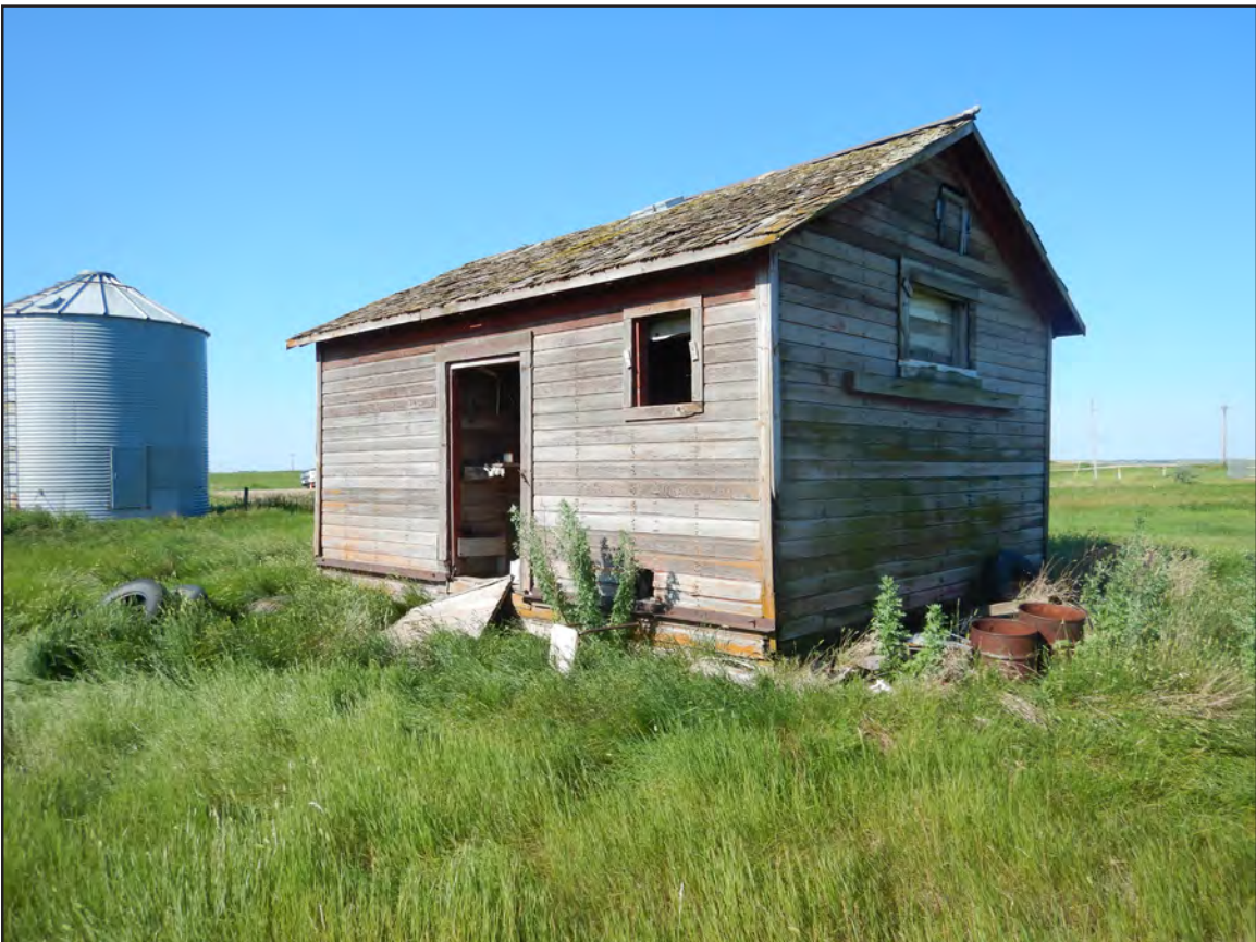
Figure 3. 32MN1338, Feature 2, east and north elevations, view to the southwest.
