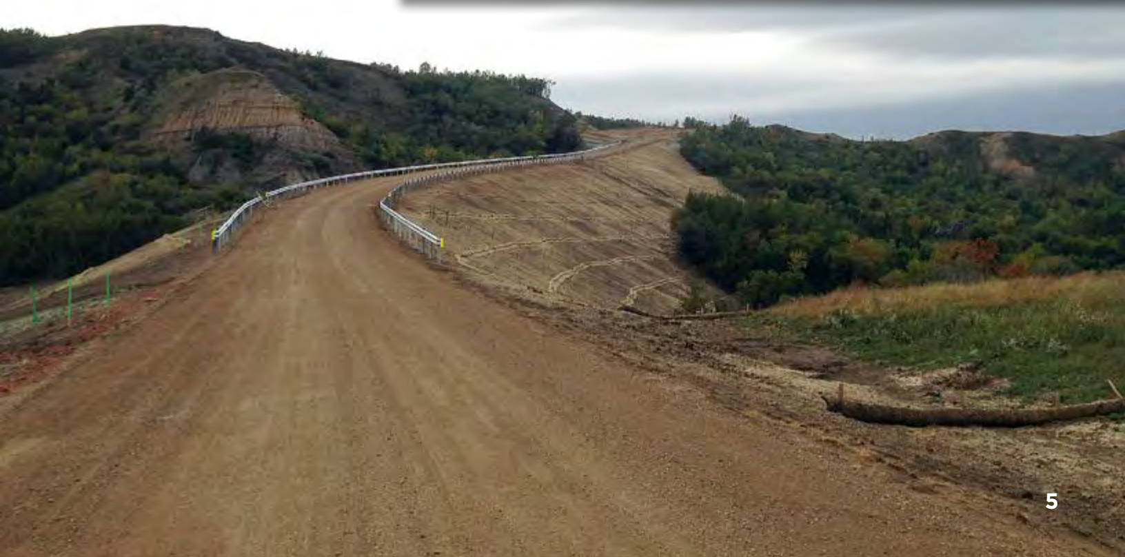
Example of construction and reclamation of an access road during and after construction.
