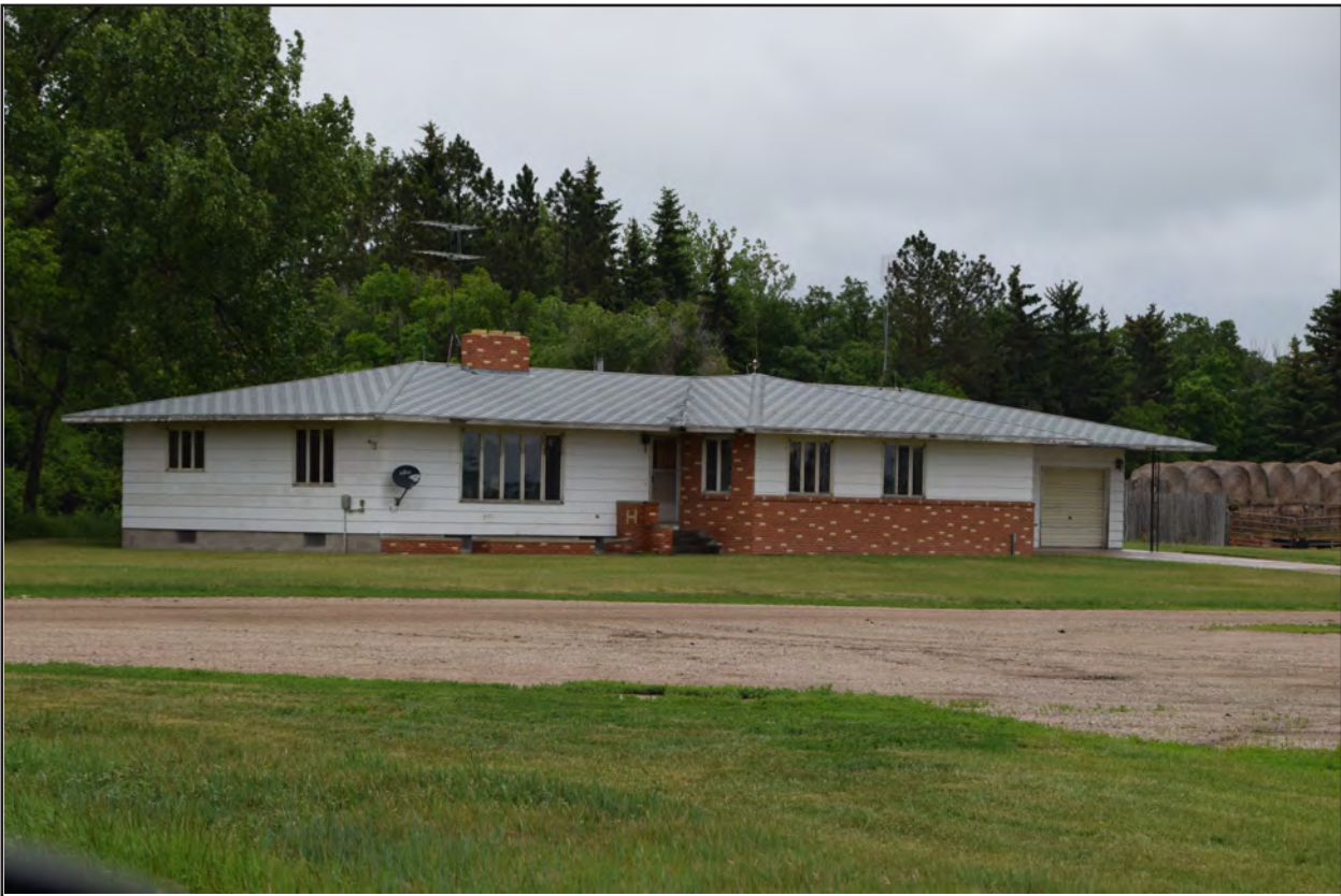
Figure 29. 32BK297, Feature 1, south and west elevations, view to the northeast.
