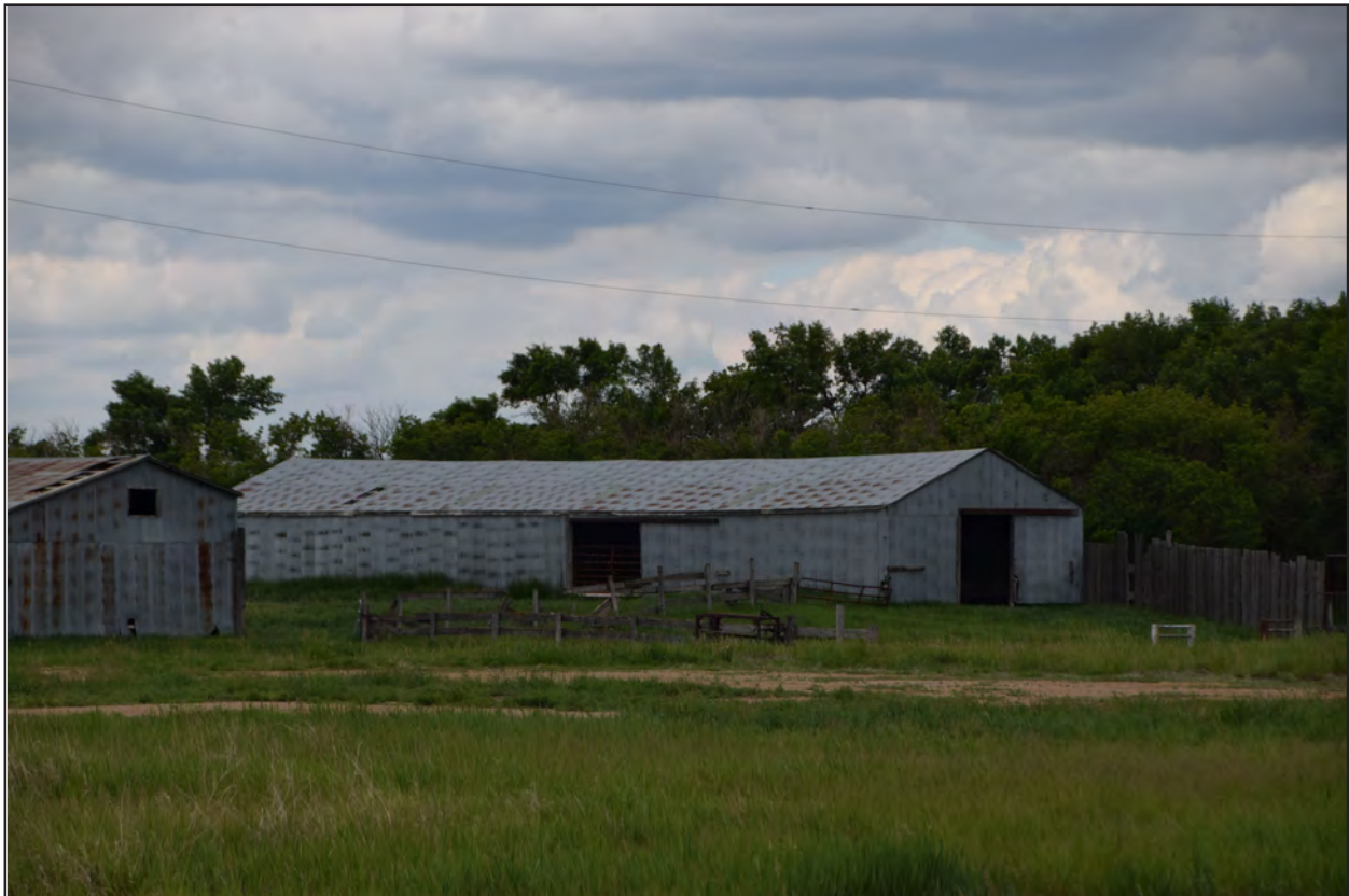
Figure 26. 32BK296, Feature 5, view to the southwest.
