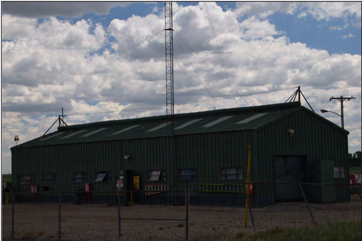
Figure 14. 32BK295, Feature 6, north and east elevations, view to the southeast.
