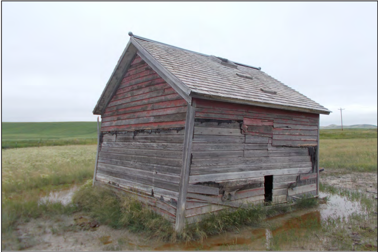
Figure 61. 32MZ3336, Feature 1, south and east elevations, view to the northwest.
