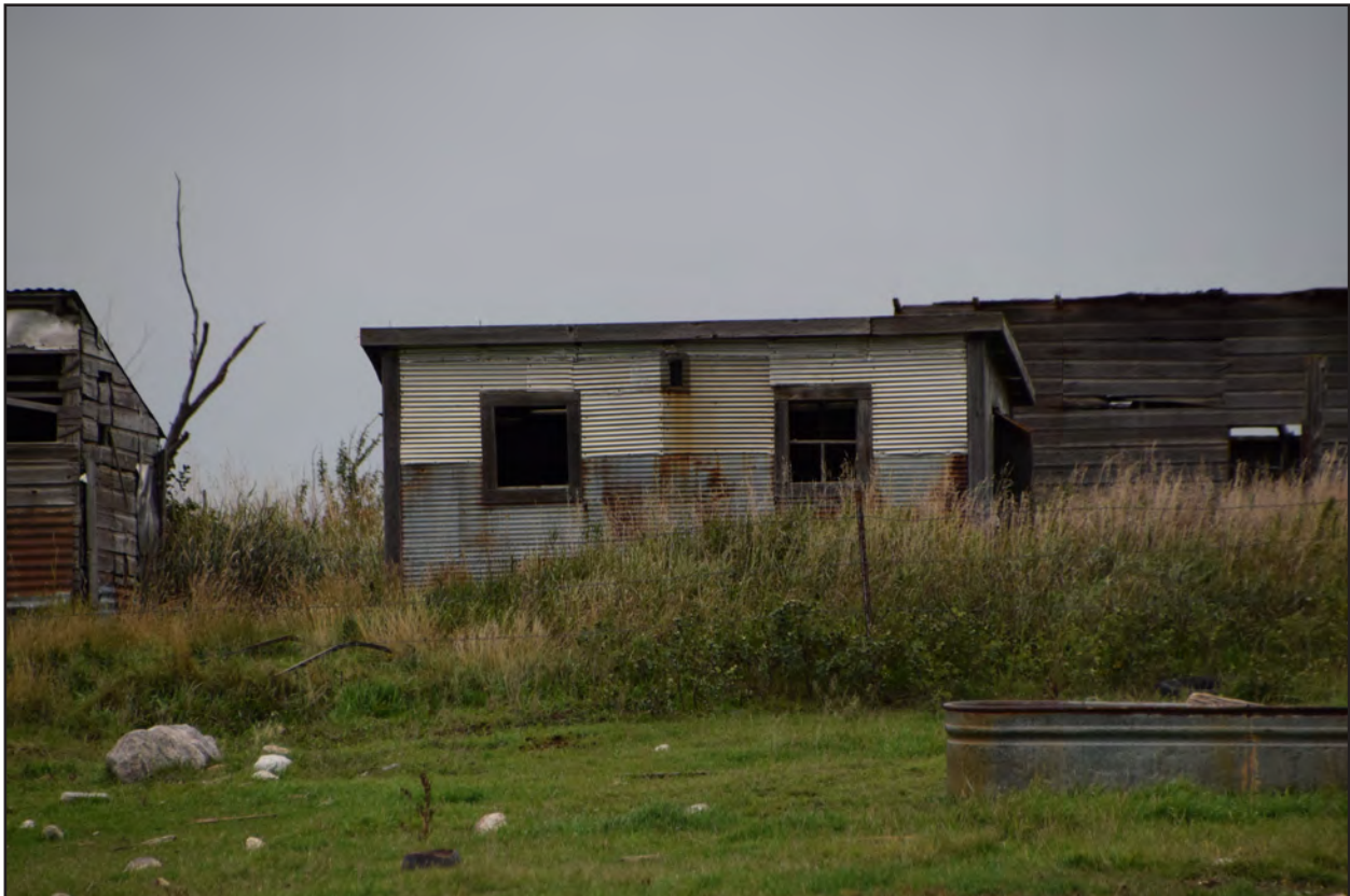
Figure 105. 32WI2411, Feature 21, south and east elevations, view to the northwest.
