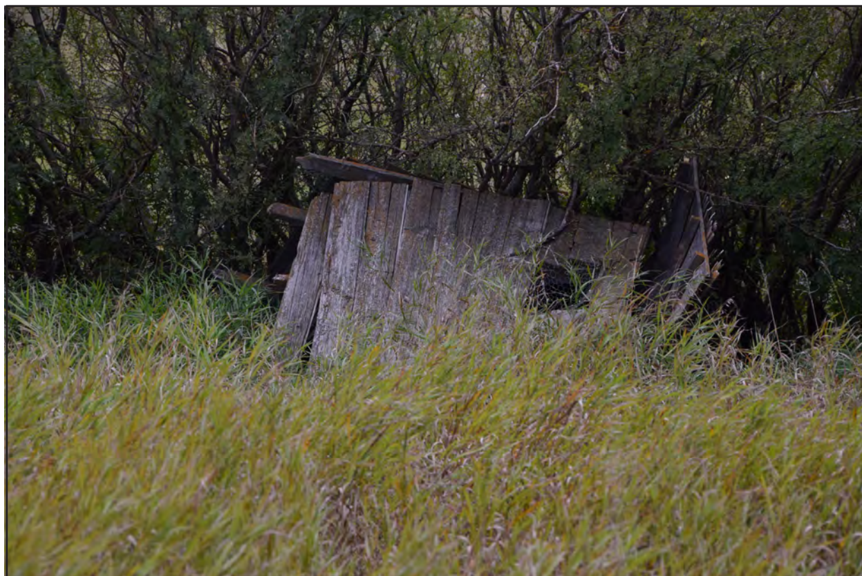
Figure 95. 32WI2411, Feature 8, east elevation, view to the west.
