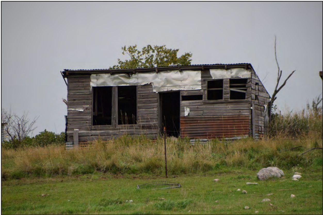
Figure 104. 32WI2411, Feature 20, south and east elevations, view to the northwest.
