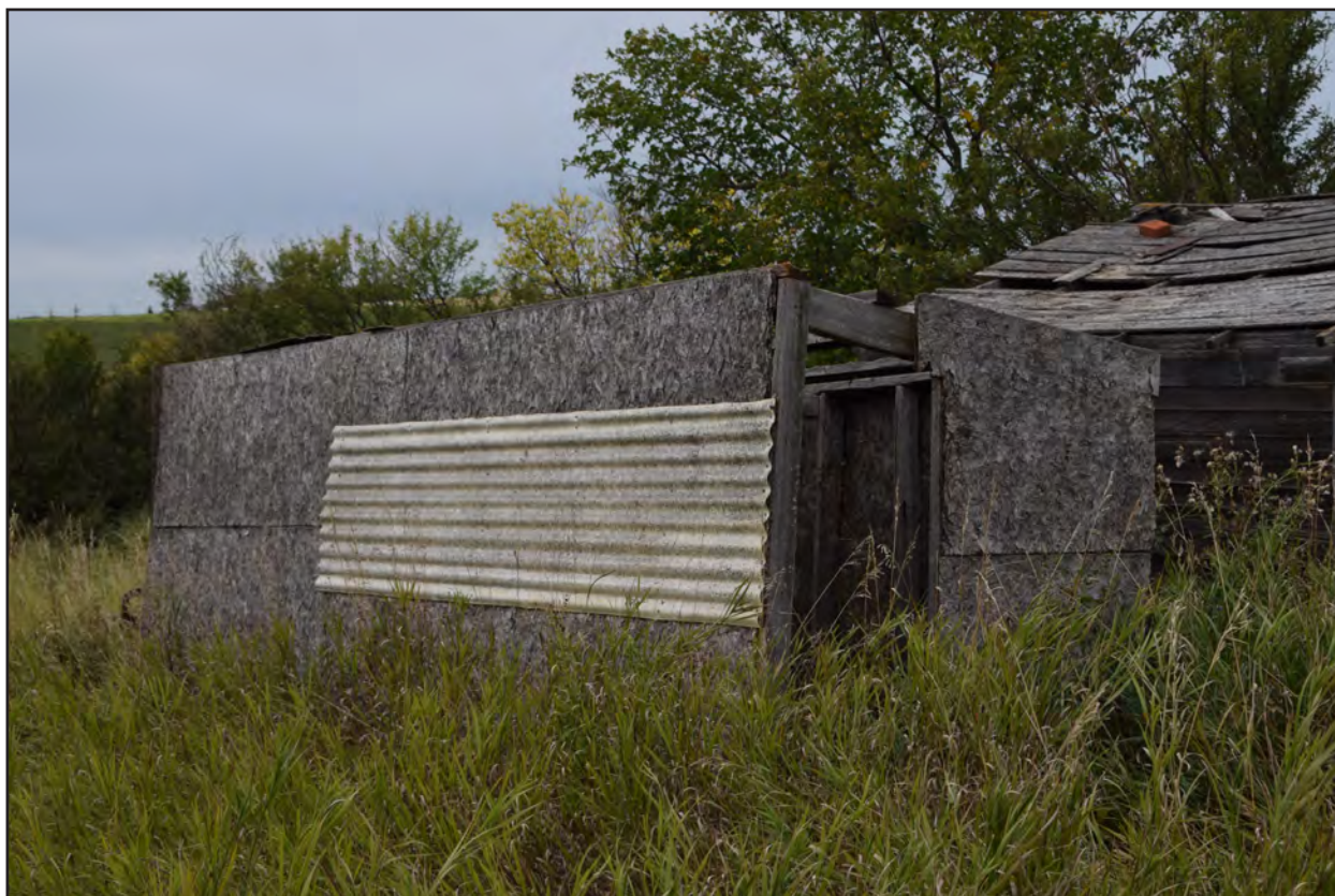
Figure 94. 32WI2411, Feature 7, south and east elevations, view to the northwest.
