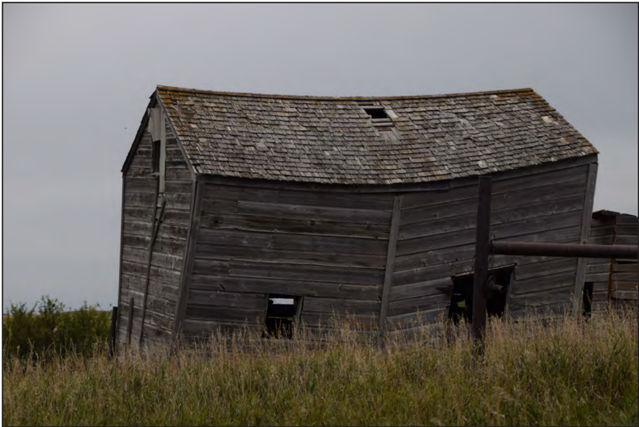
Figure 100. 32WI2411, Feature 15, east and south elevations, view to the northwest.
