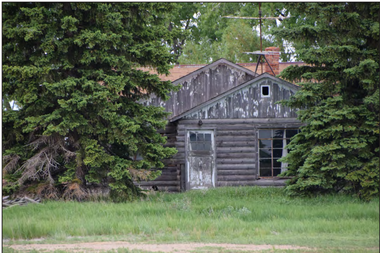
Figure 22. 32BK296, Feature 1, view to the west.
