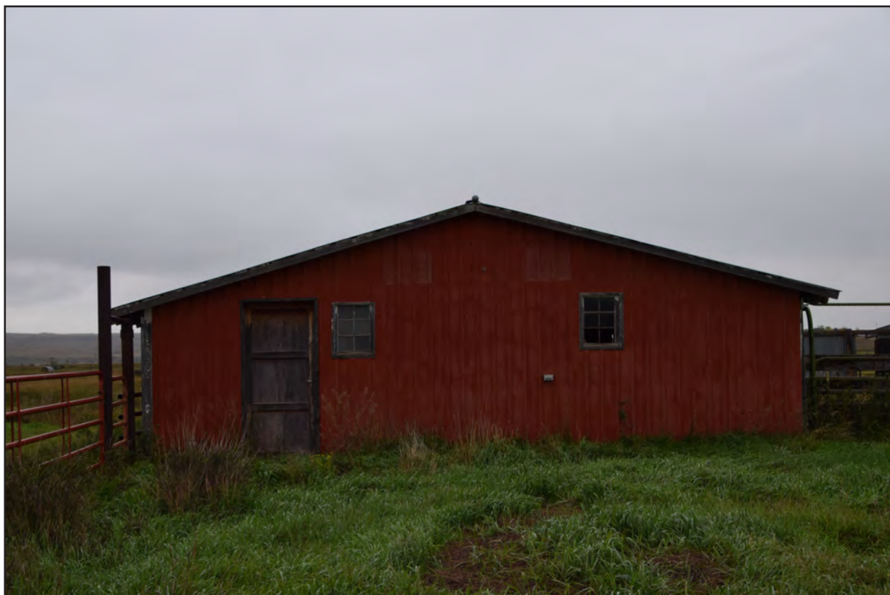
Figure 73. 32MZ3337, Feature 9, south elevation, view to the north.
