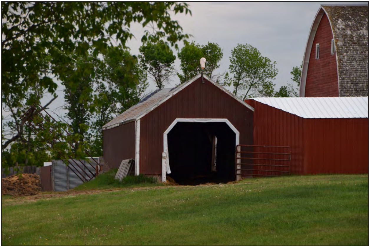
Figure 4. 32BK293, Feature 2, south and west elevations, view to the northeast.
