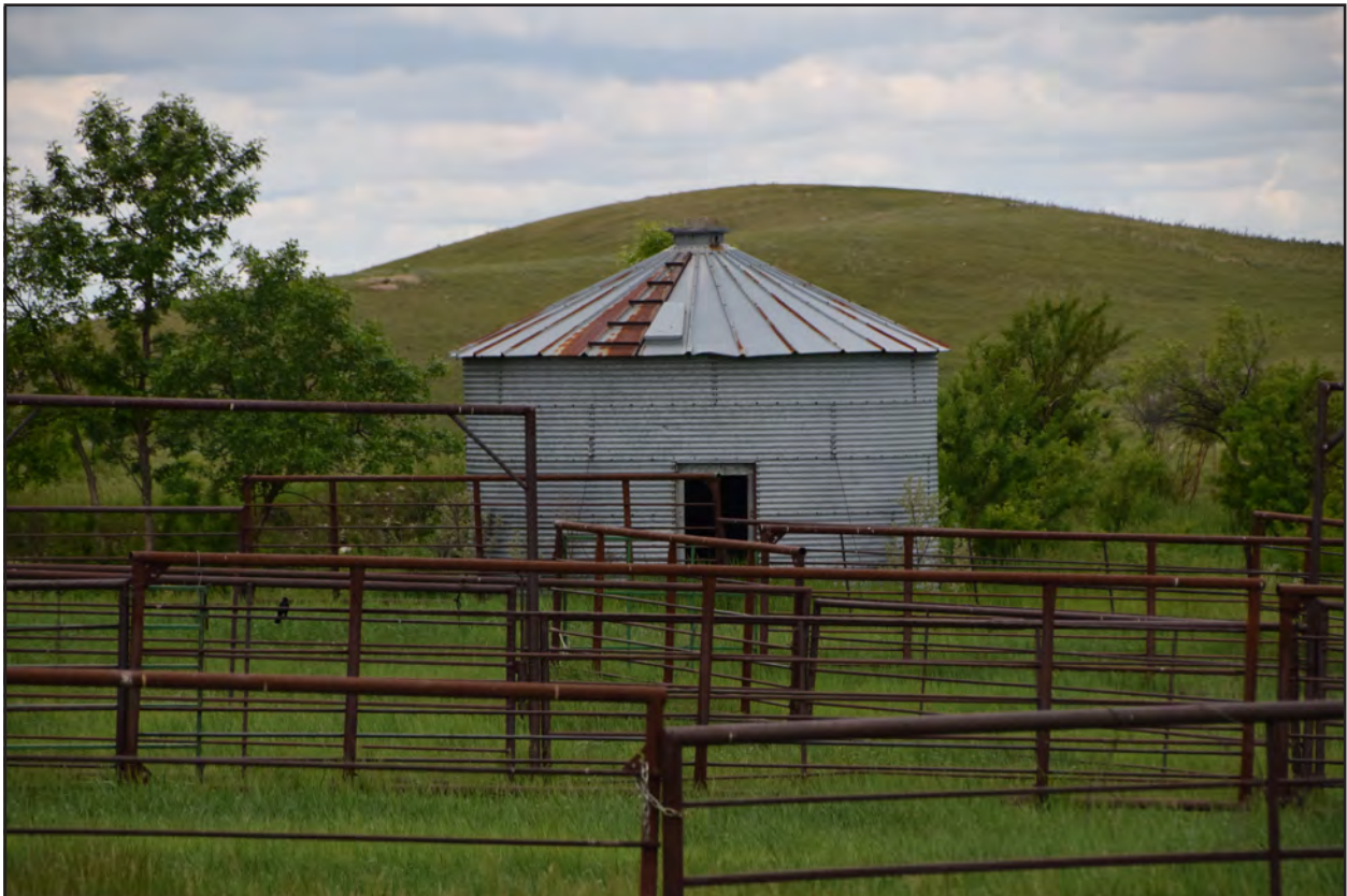
Figure 24. 32BK296, Feature 3, view to the west.
