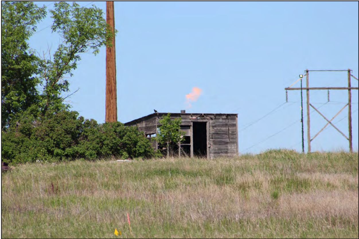
Figure 83. 32WI897, Feature 1, west and south elevations, view to the northwest. Photographed June 2019.
