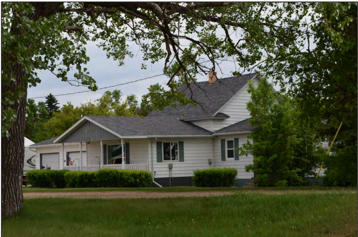
Figure 3. 32BK293, Feature 1 and west addition, south and west elevations, view to the northeast.
