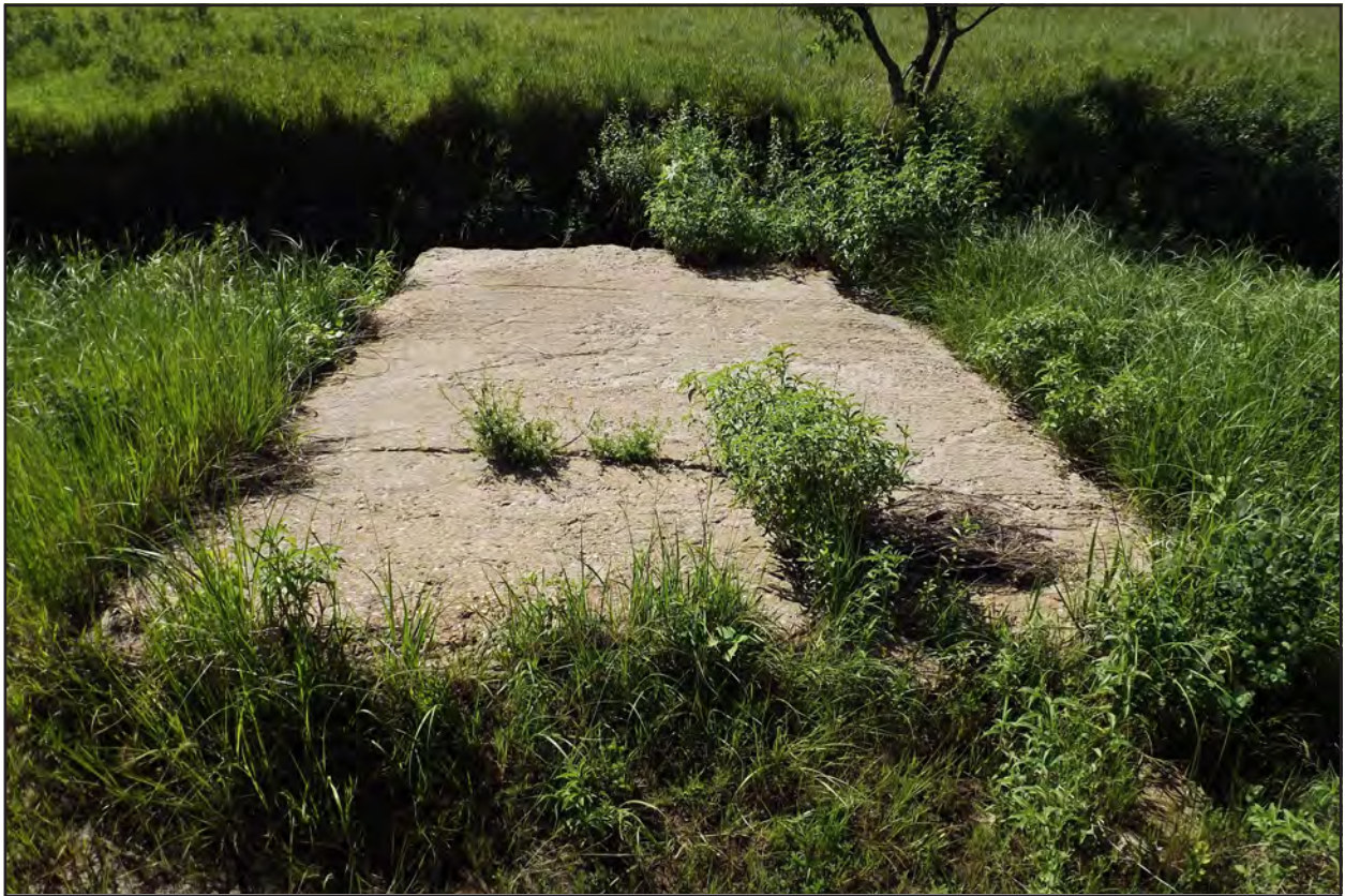
Figure 58. 32MZ3151, Feature 1, bridge detail, view to the south.
