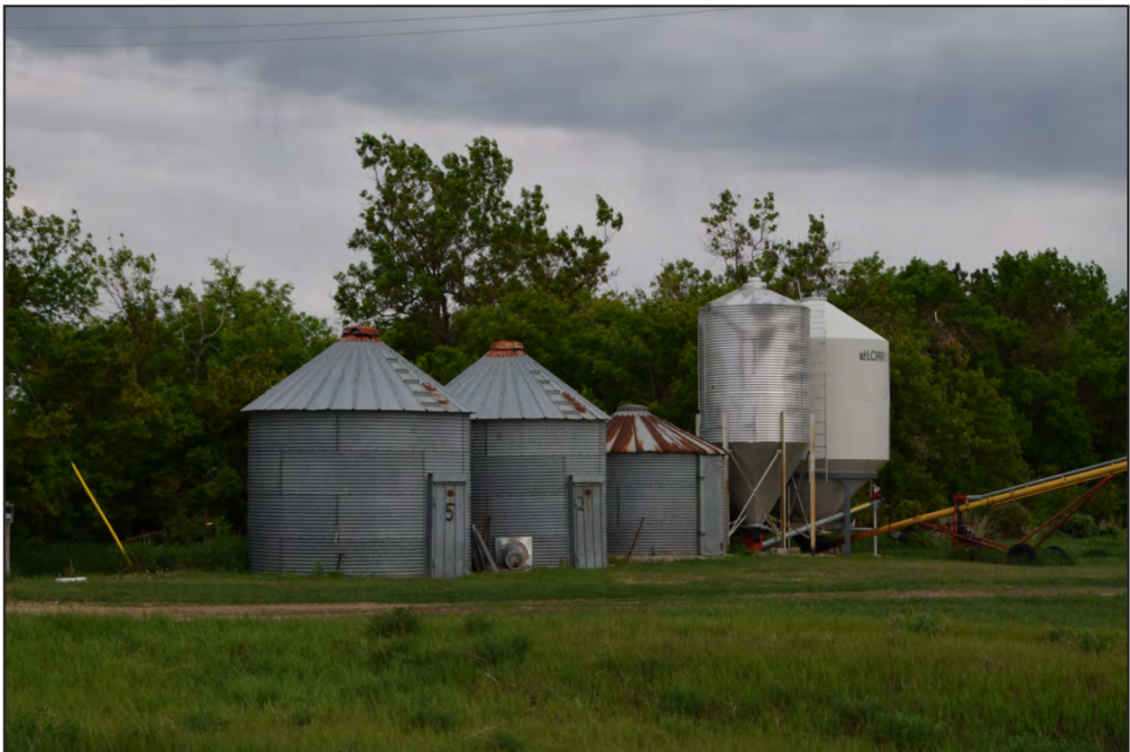
Figure 7. 32BK293, Features 5 and 6, south and east elevations, view to the northwest.
