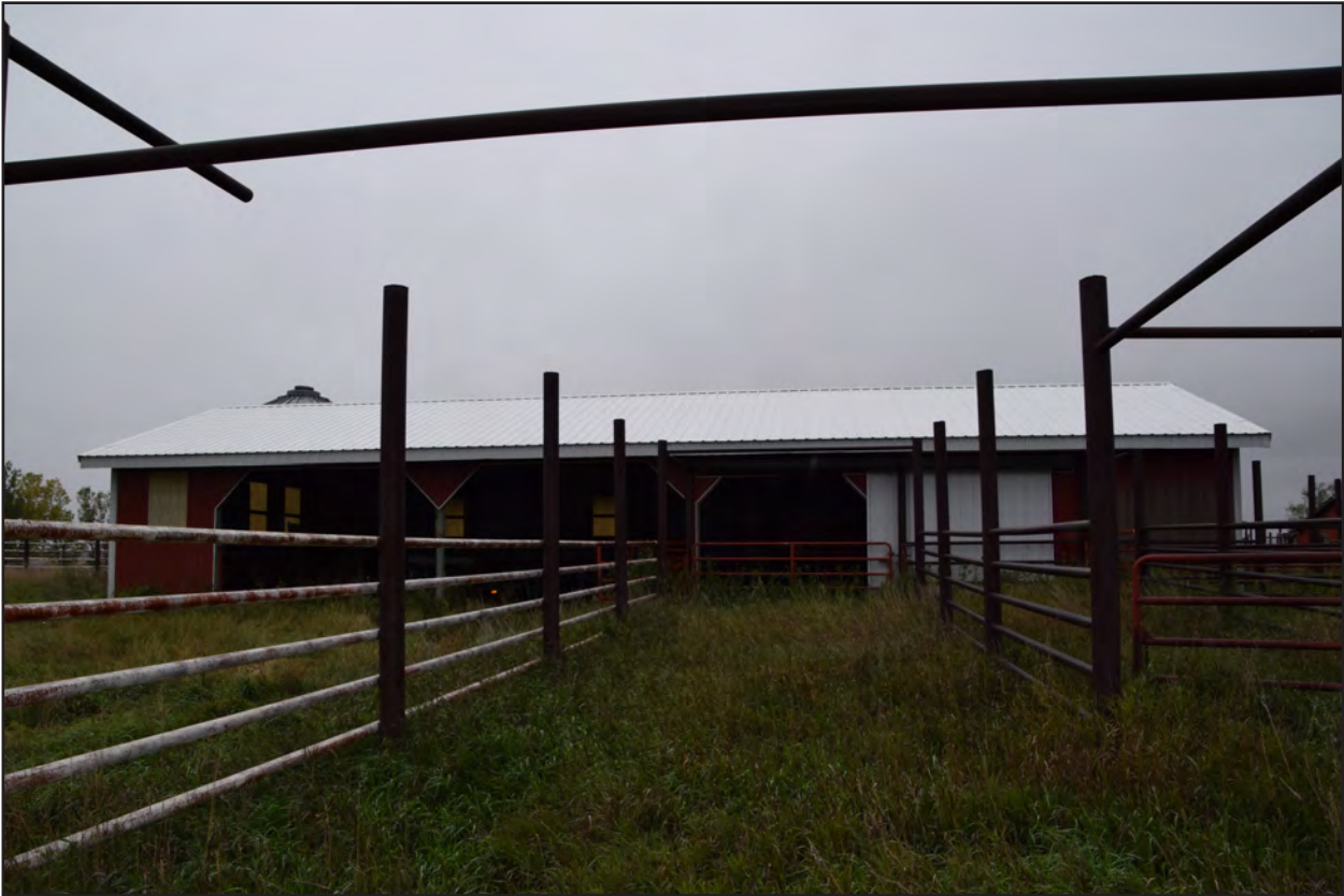
Figure 76. 32MZ3337, Feature 12, east elevation, view to the west.
