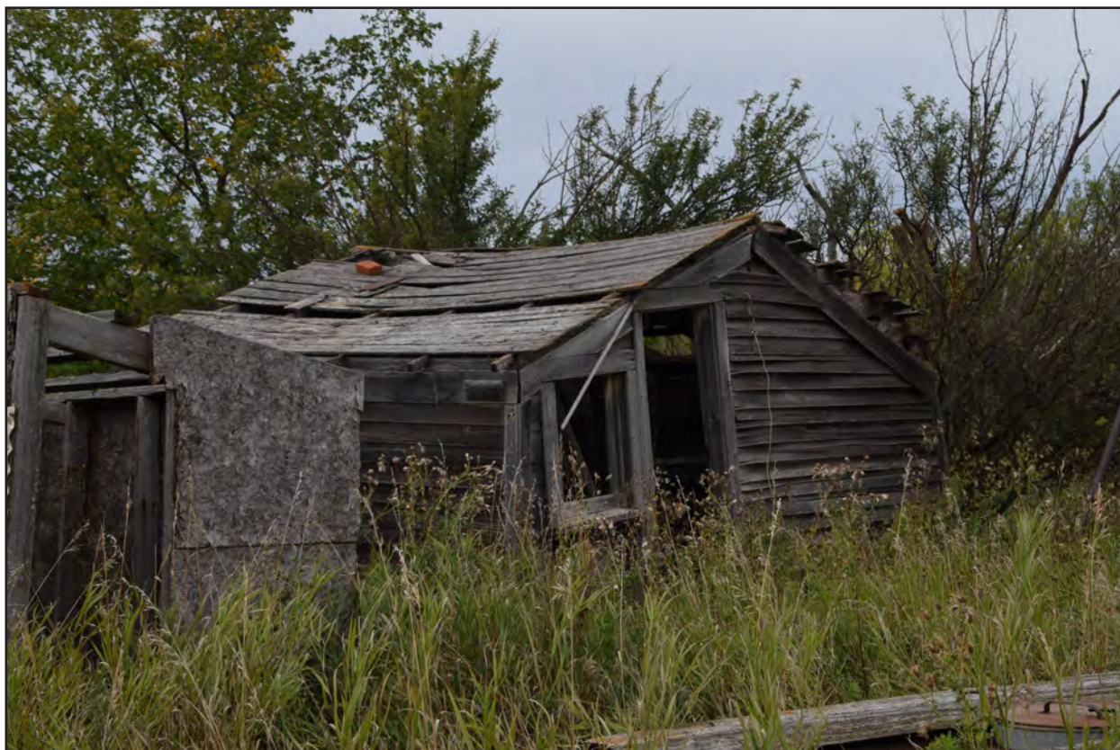
Figure 93. 32WI2411, Feature 6, east and south elevations, view to the northwest.
