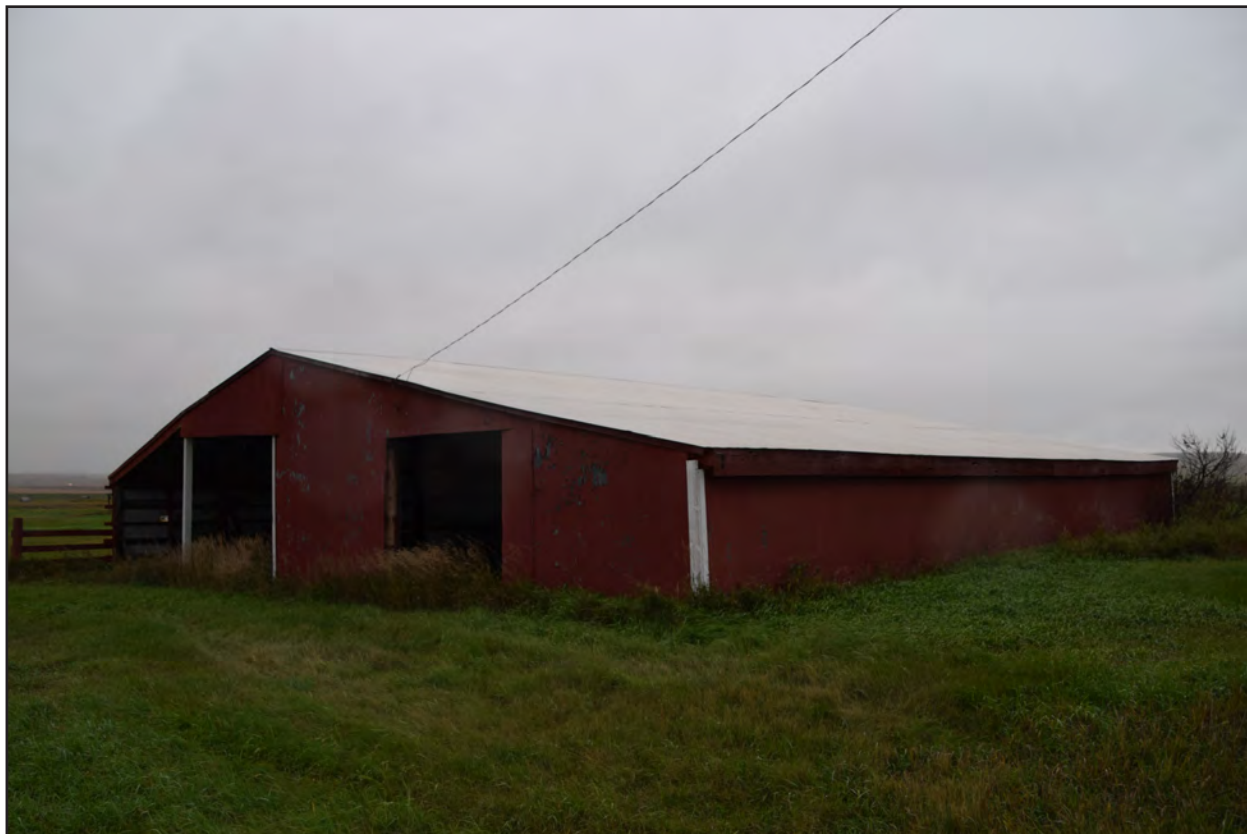
Figure 70. 32MZ3337, Feature 6, south and east elevations, view to the northwest.
