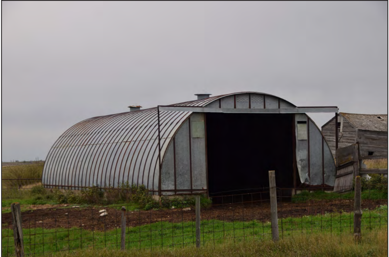
Figure 106. 32WI2411, Feature 22, east and south elevations, view to the northwest.
