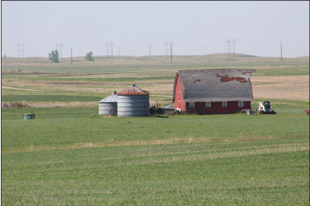
Figure 46. 32MN1584, (from left to right) Feature 3, Feature 2, and Feature 1, north and east elevations, view to the southwest.
