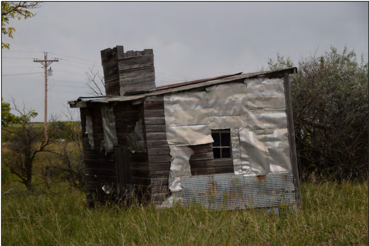
Figure 89. 32WI2411, Feature 2, northeast and southeast elevations, view to the west.
