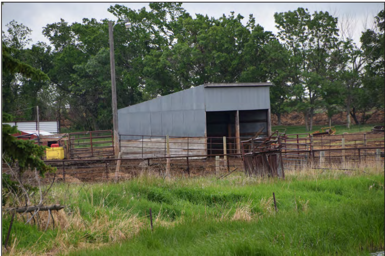
Figure 33. 32BK297, Feature 5, west and south elevations, view to the northeast.
