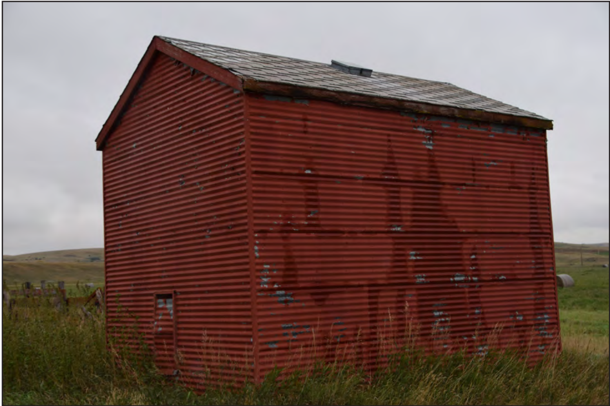
Figure 71. 32MZ3337, Feature 7, north and west elevations, view to the southeast.
