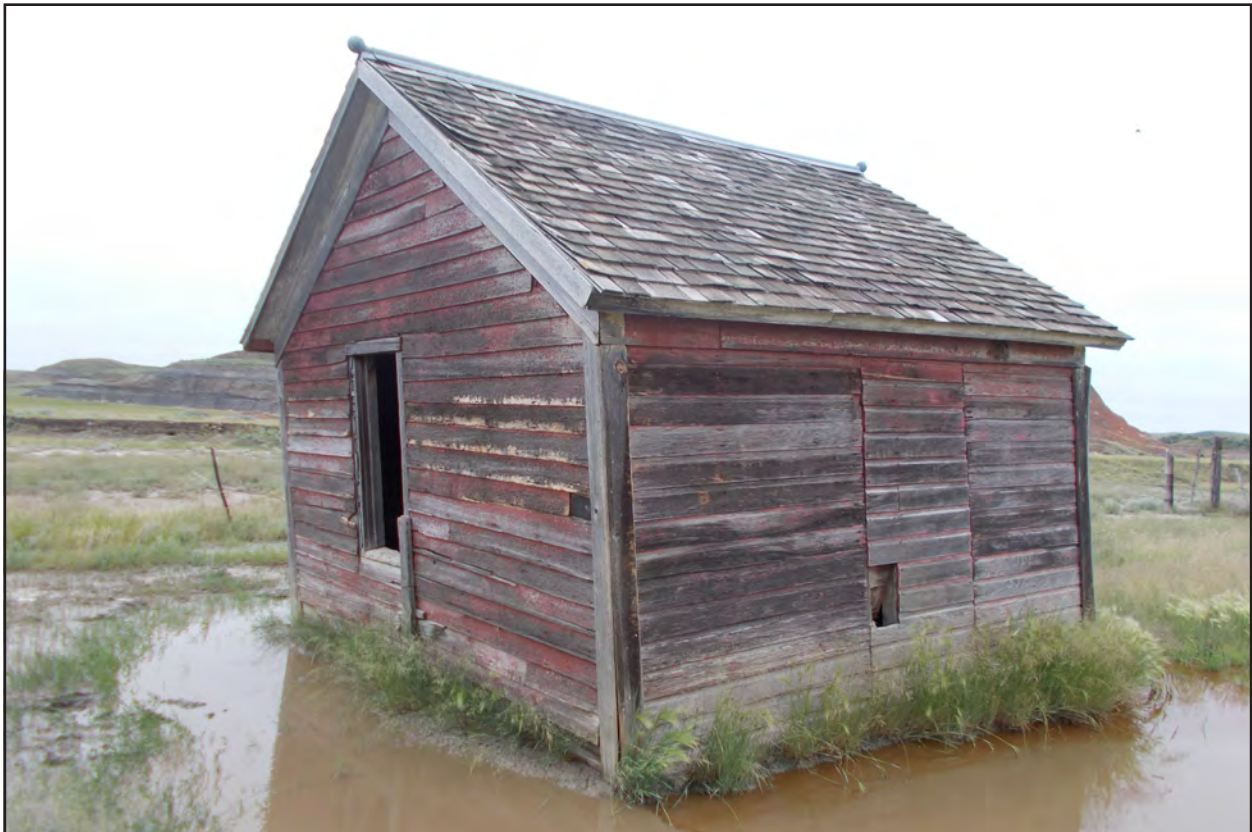
Figure 62. 32MZ3336, Feature 1, north and west elevations, view to the southeast.
