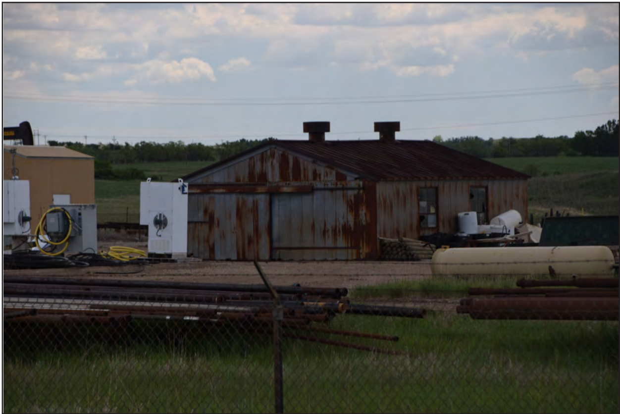
Figure 13. 32BK295, Feature 1, north and west elevations, view to the southeast.
