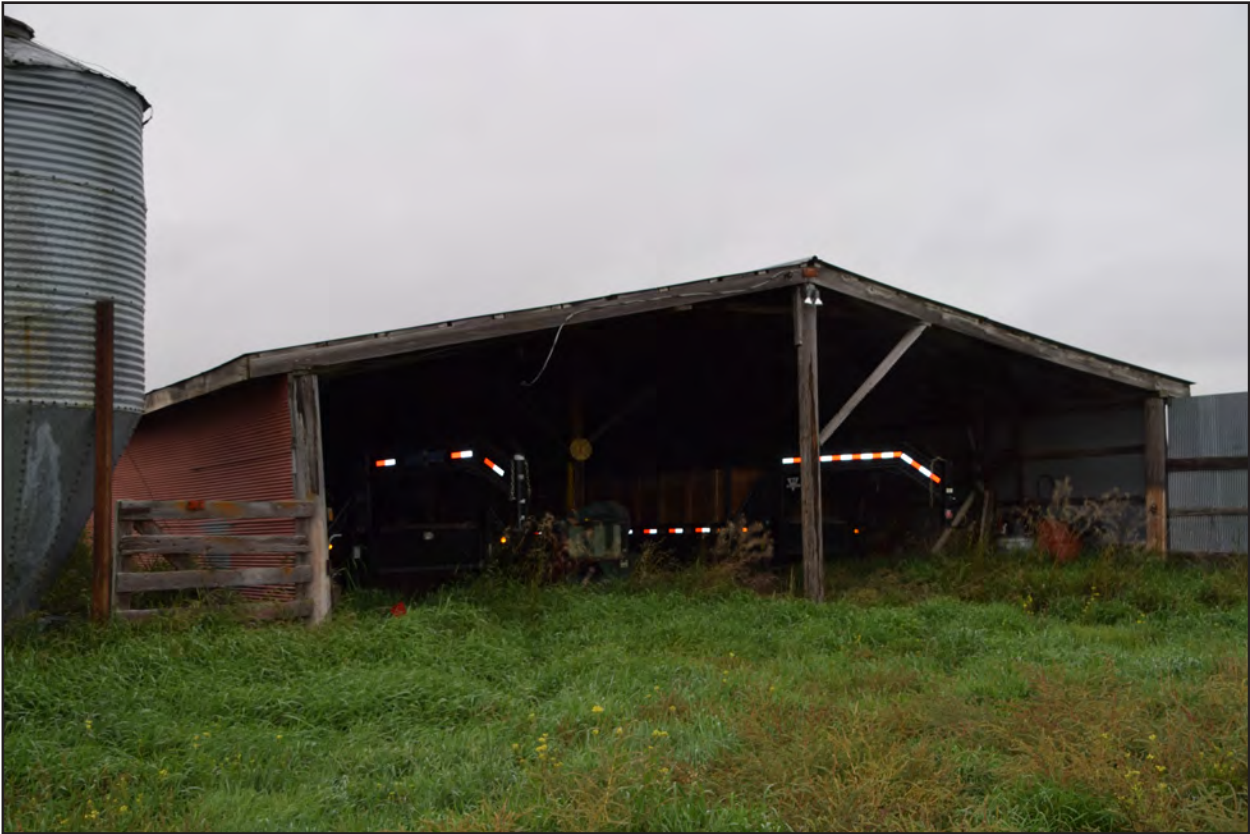
Figure 78. 32MZ3337, Feature 14, east and south elevations, view to the northwest.
