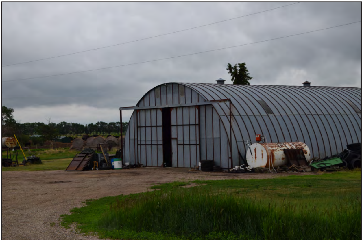
Figure 34. 32BK297, Feature 6, north and west elevations, view to the southeast.
