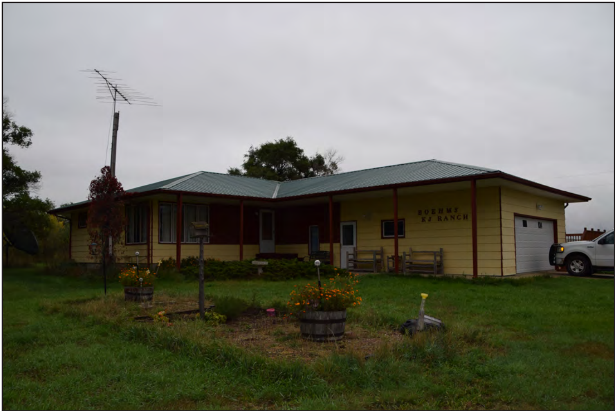
Figure 65. 32MZ3337, Feature 1, north and west elevations, view to the southeast.
