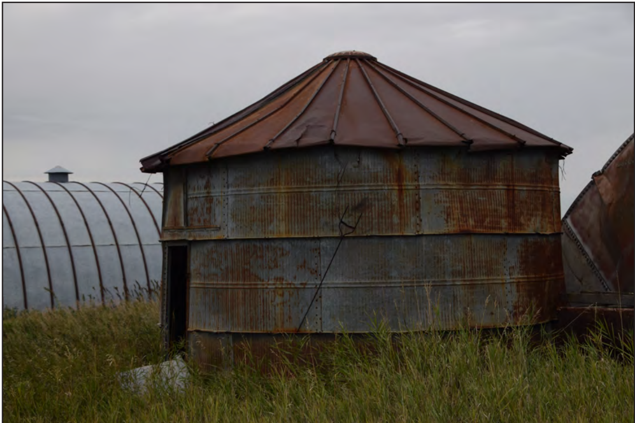
Figure 103. 32WI2411, Feature 18, east and north elevations, view to the southwest.
