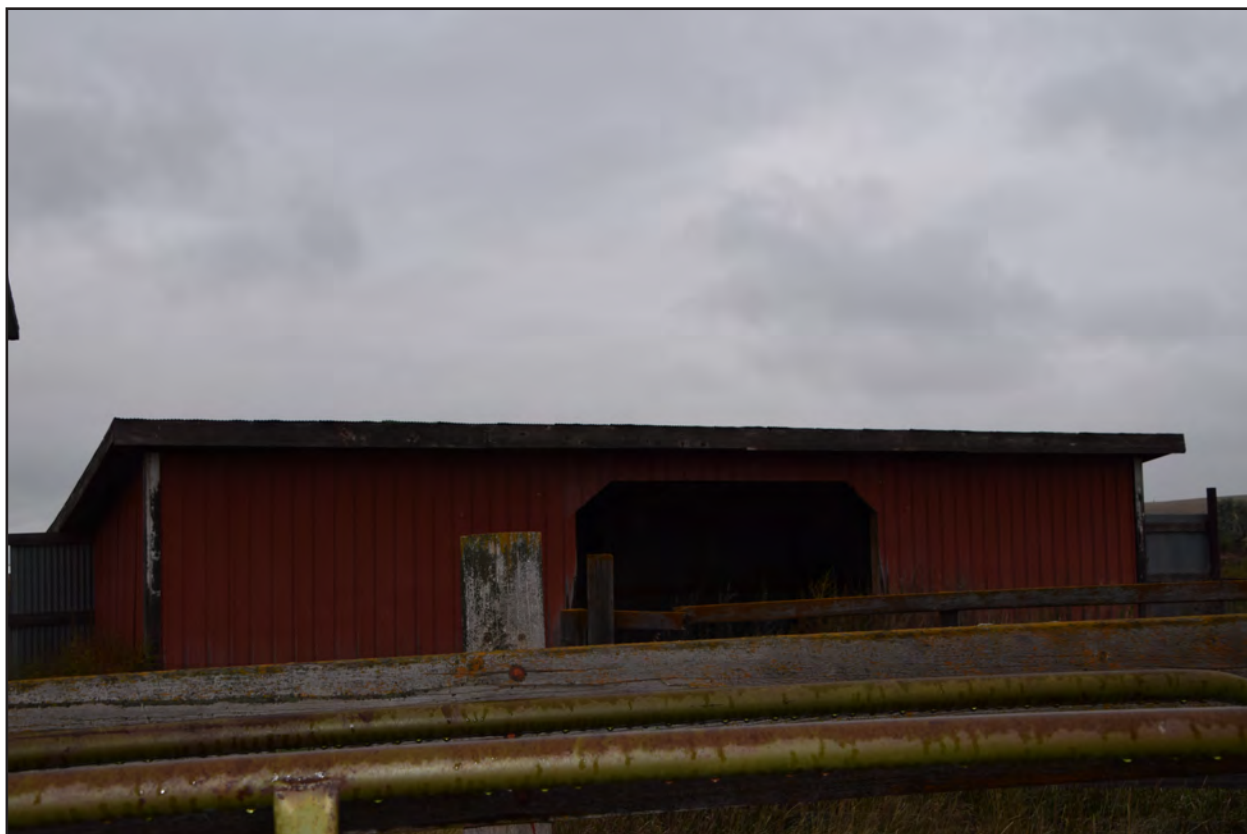
Figure 74. 32MZ3337, Feature 10, south and west elevations, view to the northeast.
