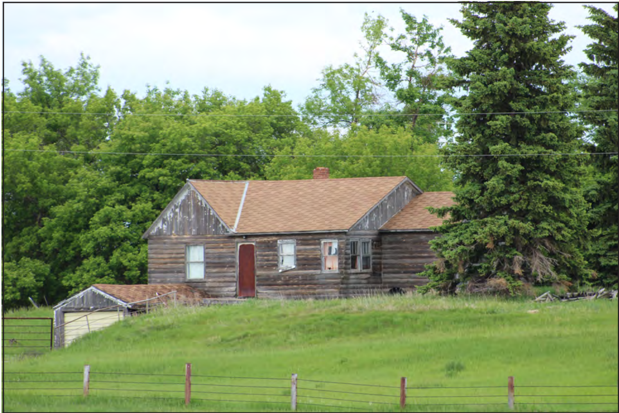
Figure 21. 32BK296, Feature 1, view to the northwest.
