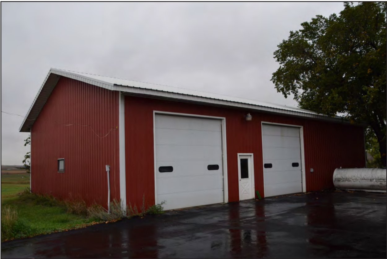
Figure 67. 32MZ3337, Feature 3, east and south elevations, view to the northwest.
