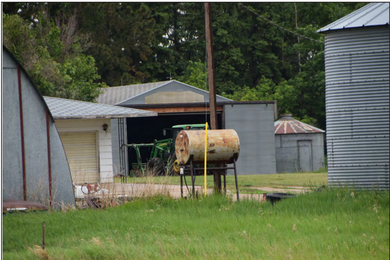
Figure 31. 32BK297, Feature 3 and Feature 7 (one of two grain bins), south elevation, view to the north-northeast.
