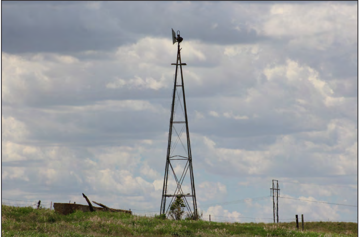
Figure 86. 32W11497, Feature 1, northeast and southeast elevations, view to the west.
