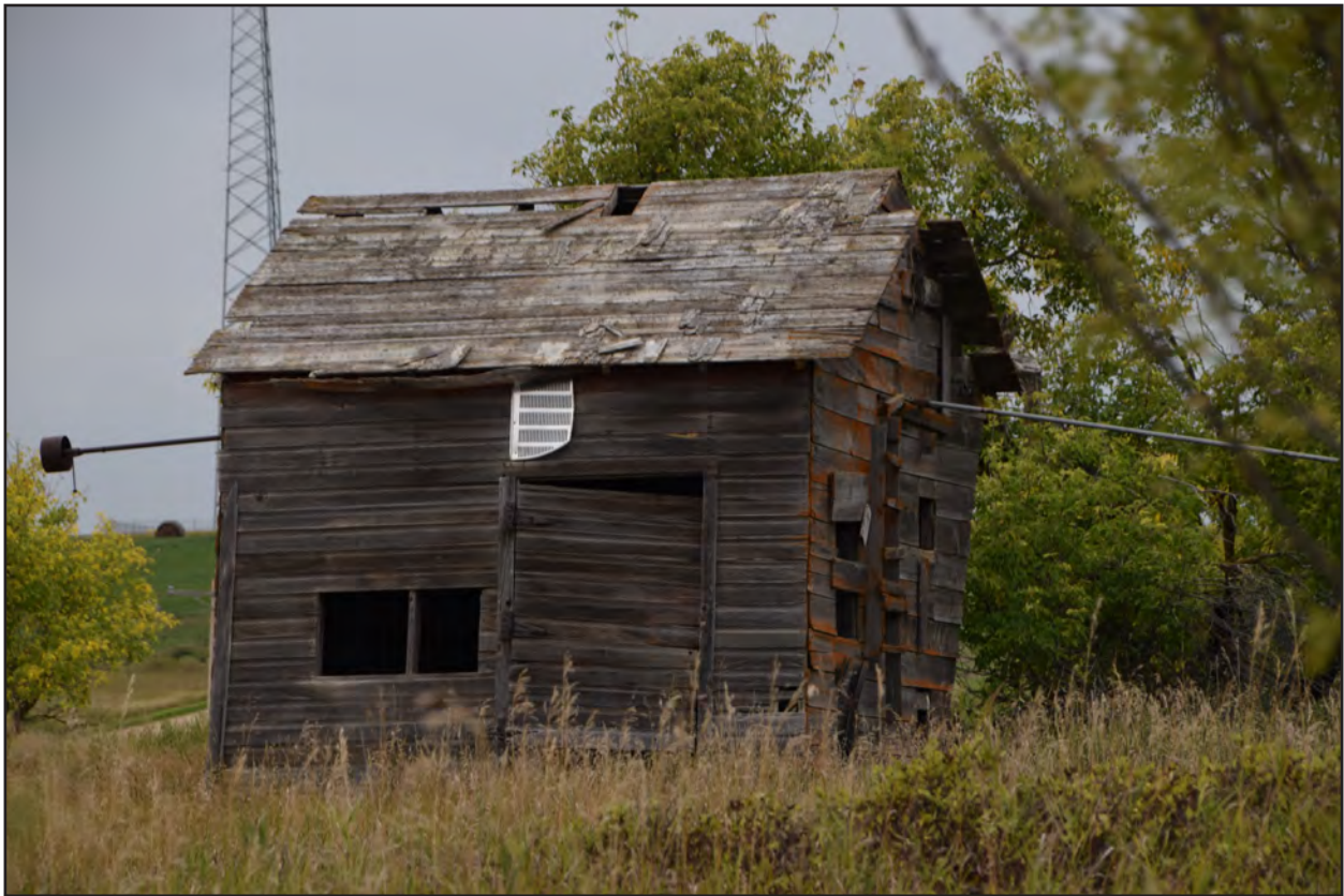
Figure 90. 32WI2411, Feature 3, south and east elevations, view to the northwest.
