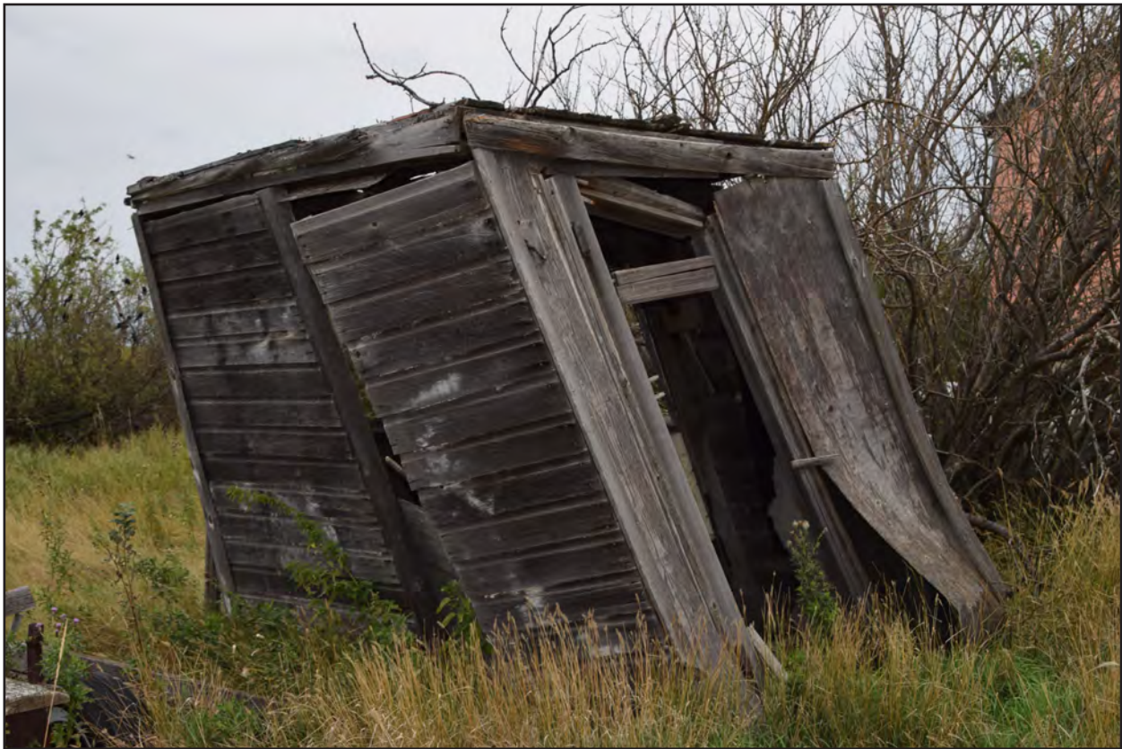
Figure 96. 32W12411, Feature 9, south and west elevations, view to the northeast.
