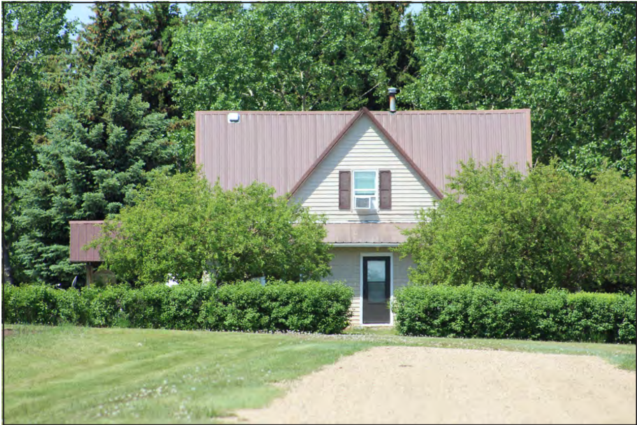
Figure 39. 32BKX1068, Feature 1, east elevation, view to the west.
