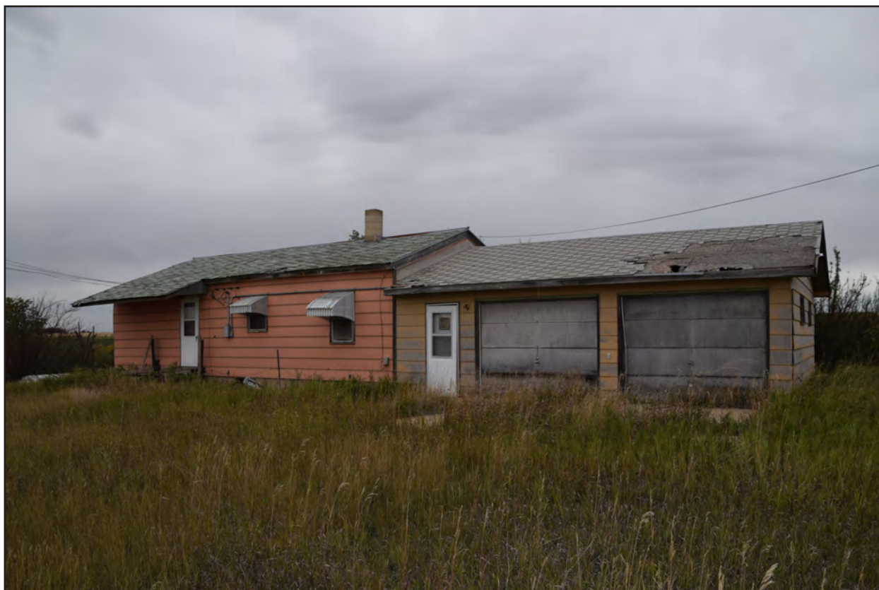
Figure 92. 32WI2411, Feature 5, south and east elevations, view to the northwest.
