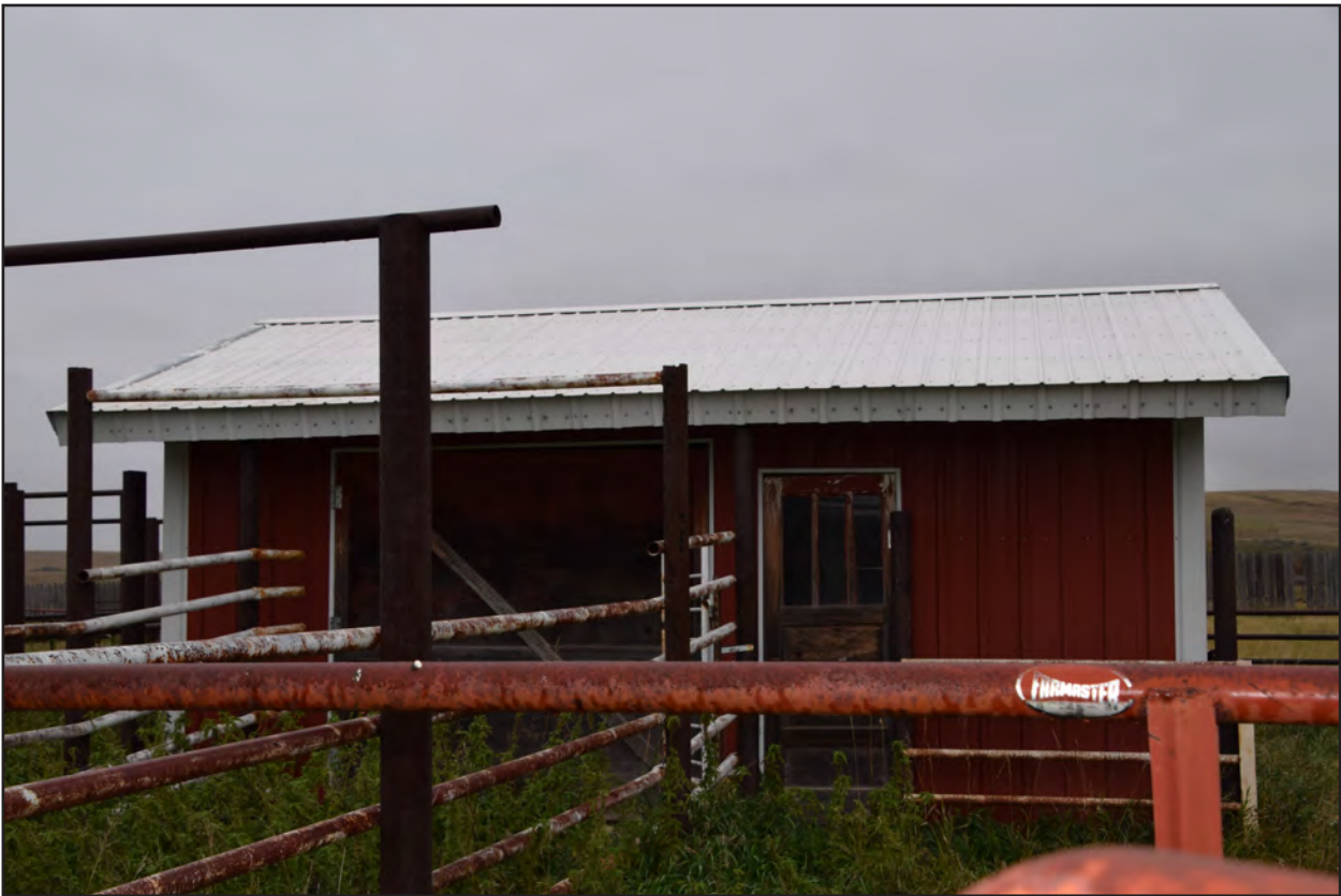
Figure 75. 32MZ3337, Feature 11, west elevation, view to the east.
