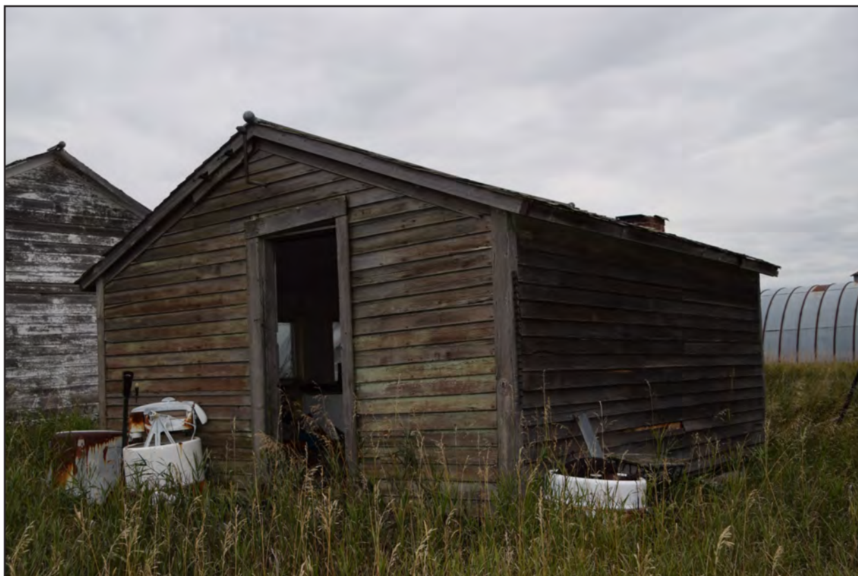
Figure 98. 32WI2411, Feature 13, north and west elevations, view to the southeast.
