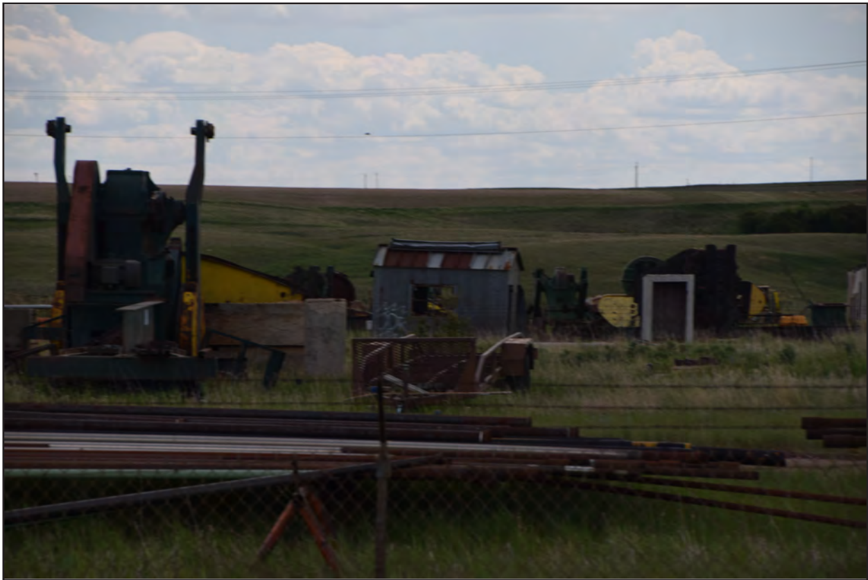
Figure 17. 32BK295, Feature 3, north elevation, view to the south.
