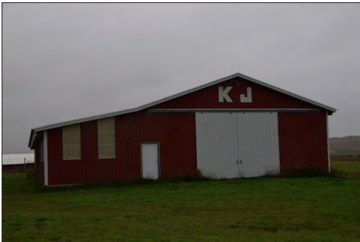
Figure 69. 32MZ3337, Feature 5, east elevation, view to the west.
