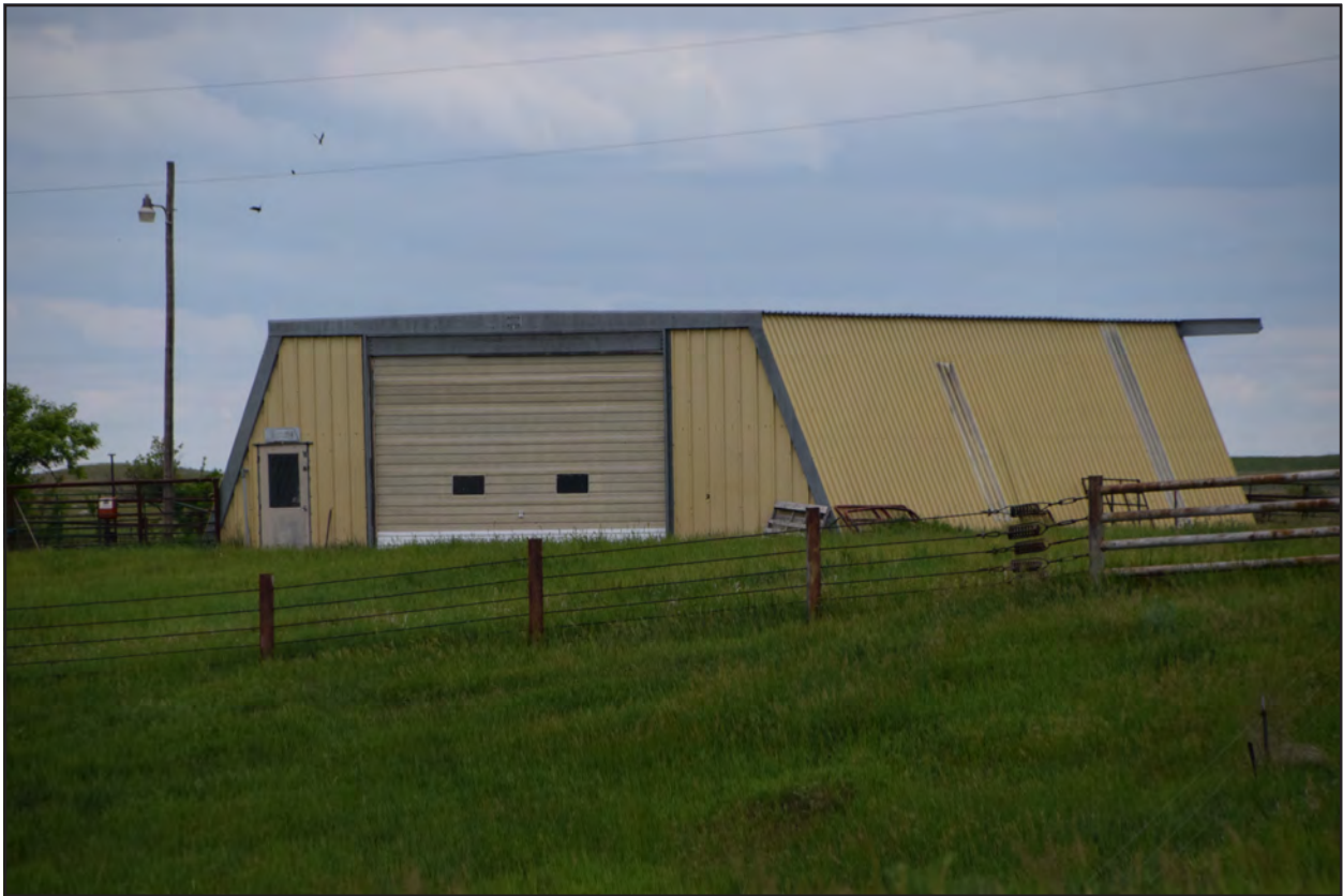
Figure 23. 32BK296, Feature 2, view to the northwest.
