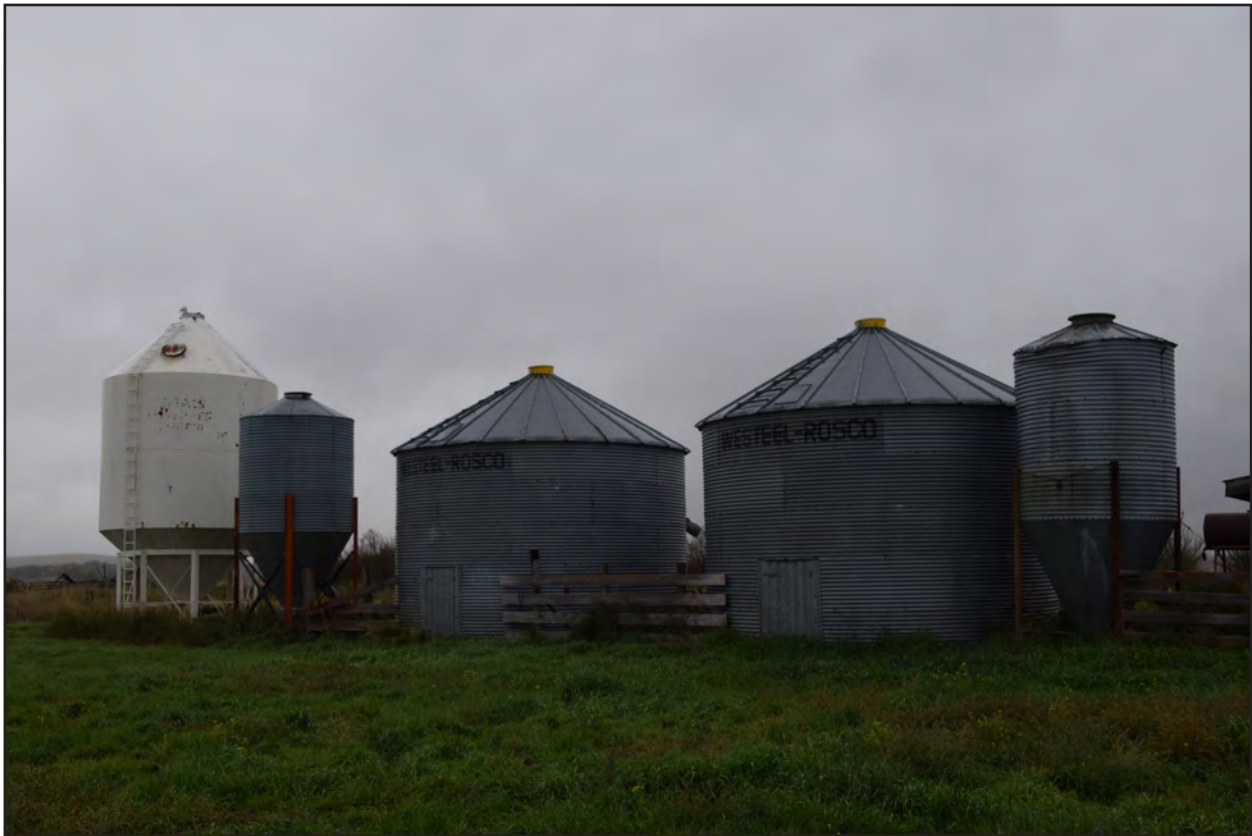
Figure 79. 32MZ3337, Feature 15, north and east elevations, view to the southwest.
