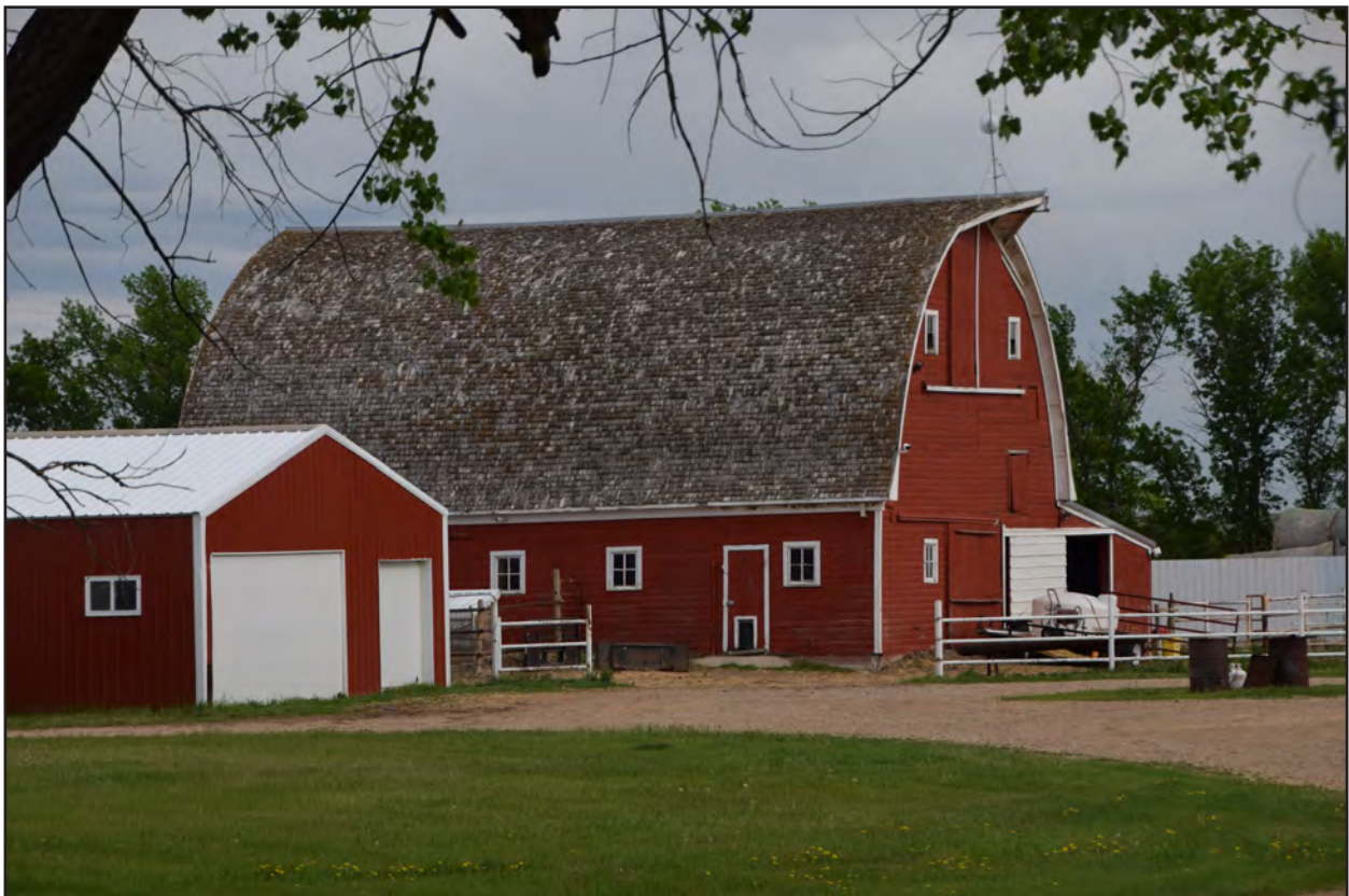
Figure 5. 32BK293, Feature 3, south and east elevations, view to the northwest.
