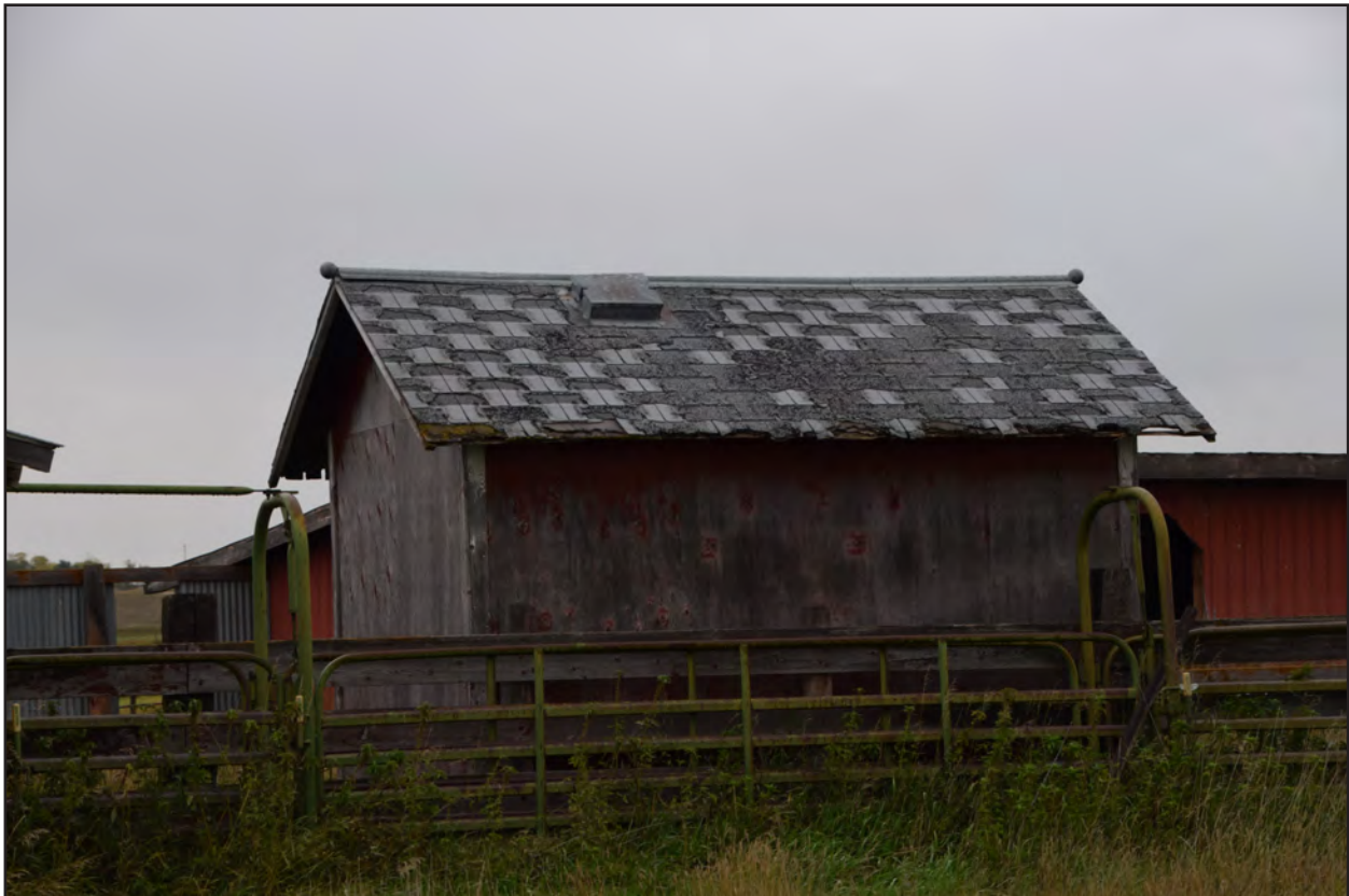
Figure 72. 32MZ3337, Feature 8, southwest and northwest elevations, view to the east.
