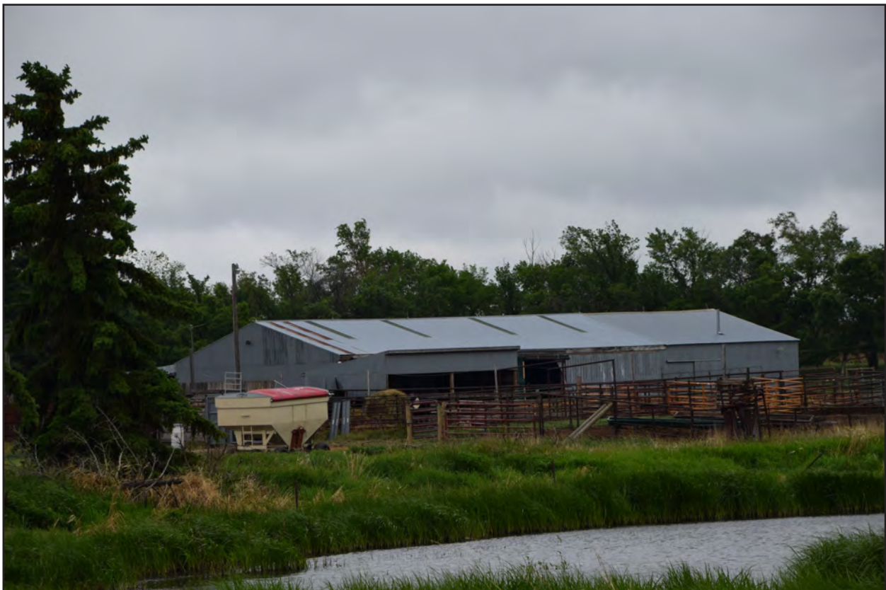
Figure 32. 32BK297, Feature 4 and Feature 13, east and south elevations, view to the northwest.
