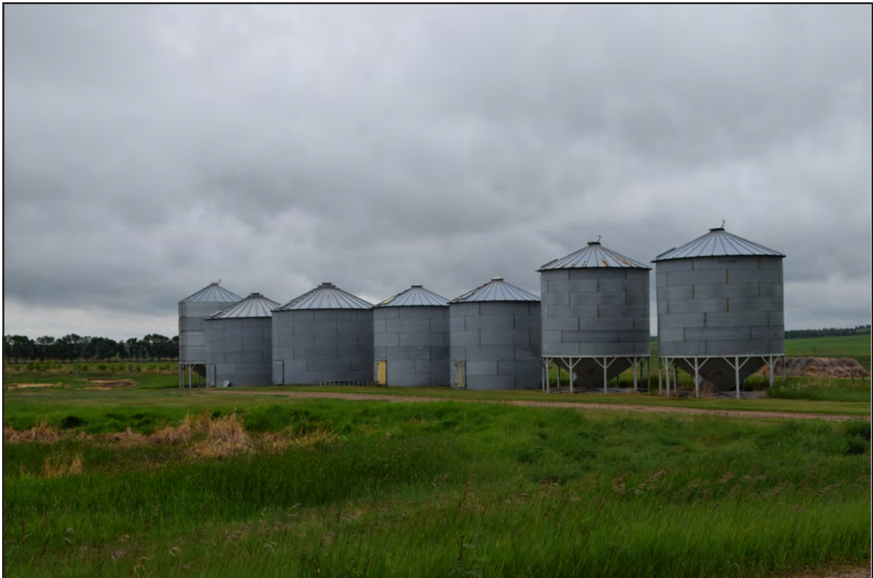
Figure 36. 32BK297, (from left to right) Feature 12 (grain feeder), Feature 9 (2 grain bins), Feature 10 (2 grain bins), and Feature 11 (2 grain feeders), view to the southeast.
