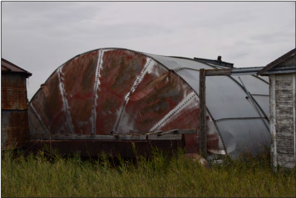
Figure 102. 32WI2411, Feature 17, east and north elevations, view to the southwest.
