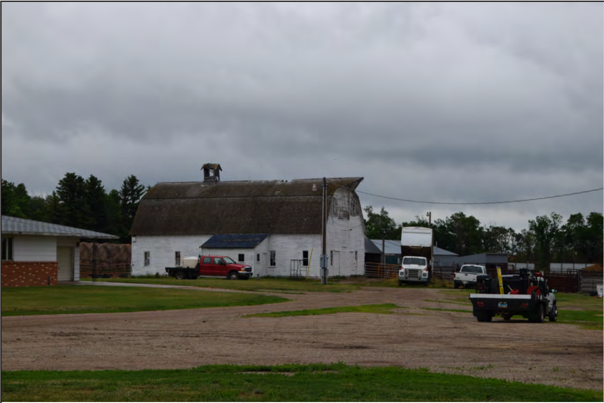
Figure 30. 32BK297, Feature 2, south and west elevations, view to the northeast.
