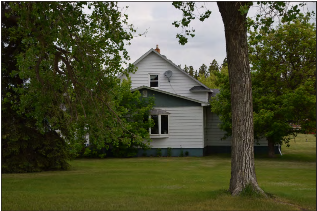
Figure 2. 32BK293, Feature 1 and south addition, south elevation, view to the north.
