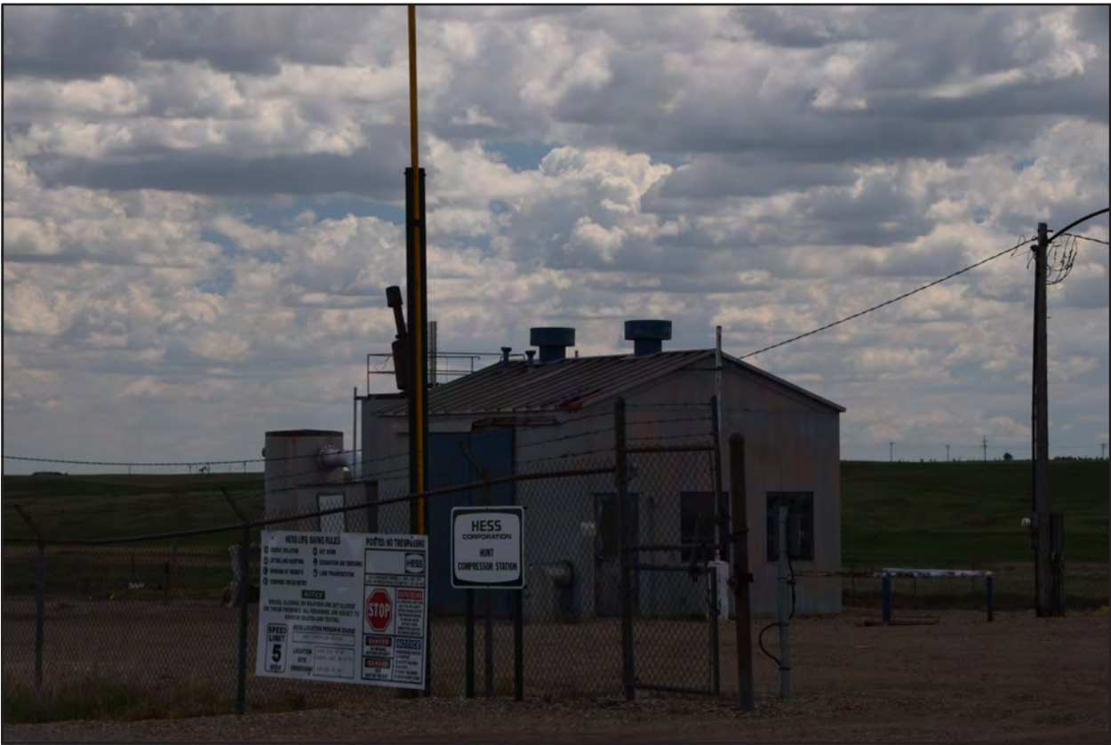
Figure 15. 32BK295, Feature 2, north and west elevations, view to the southeast.
