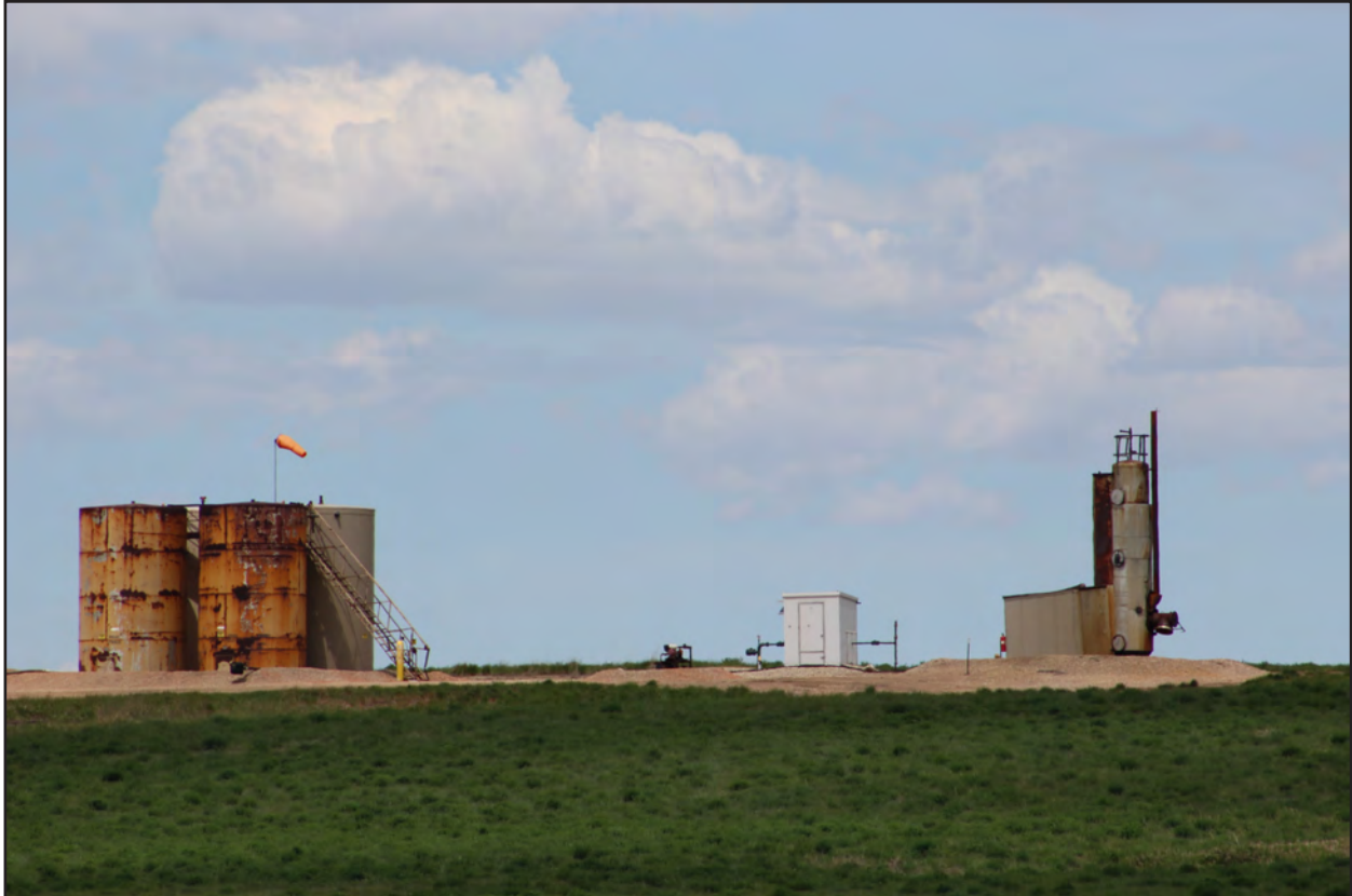
Figure 10. 32BK294, Feature 1, modern oil tanks, modern mechanical shed, and Feature 2, south and east elevations, view to the north.
