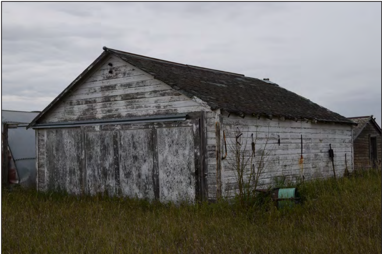
Figure 101. 32WI2411, Feature 16, east and north elevations, view to the southwest.
