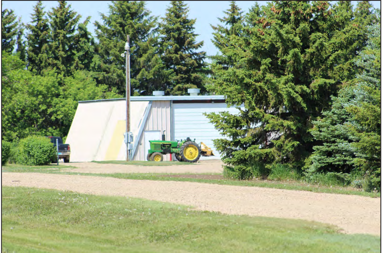
Figure 41. 32BKX1068, Feature 3, east and south elevations, view to the northwest.
