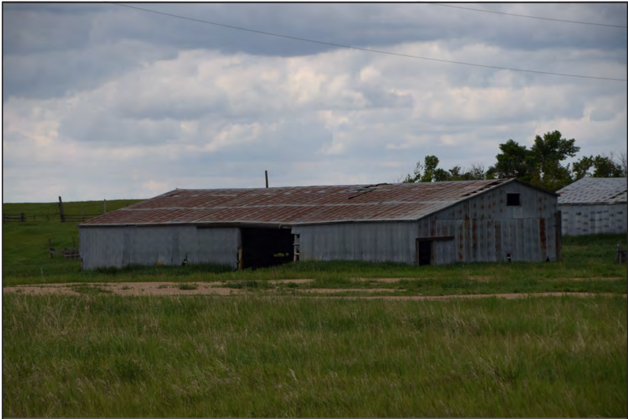
Figure 25. 32BK296, Feature 4, view to the southwest.
