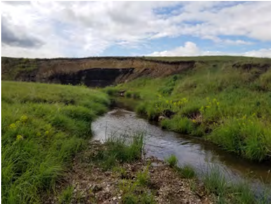
Photo 2 s-wm-eb-002p looking downstream, South
