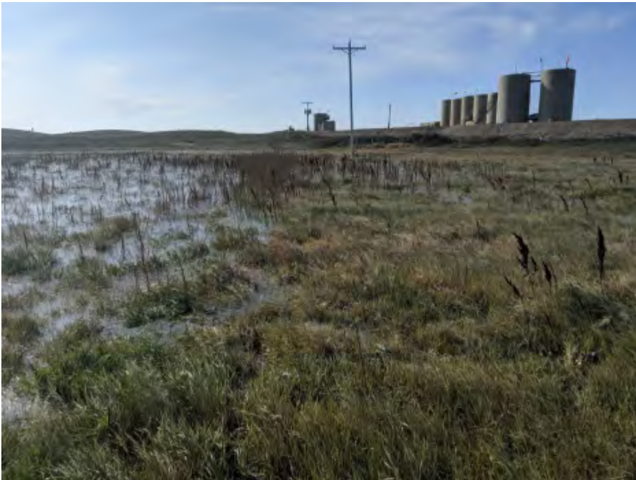
Photo 2 w-wm-ee-004e_w looking Northeast
