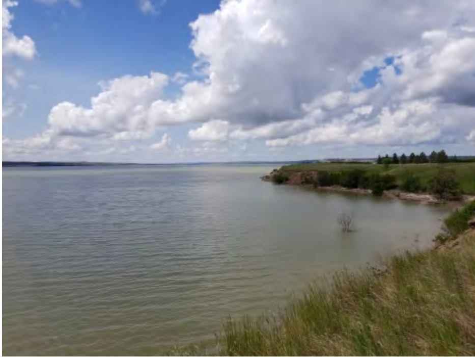
Photo 3 s-wm-eb-003p looking upstream West.
