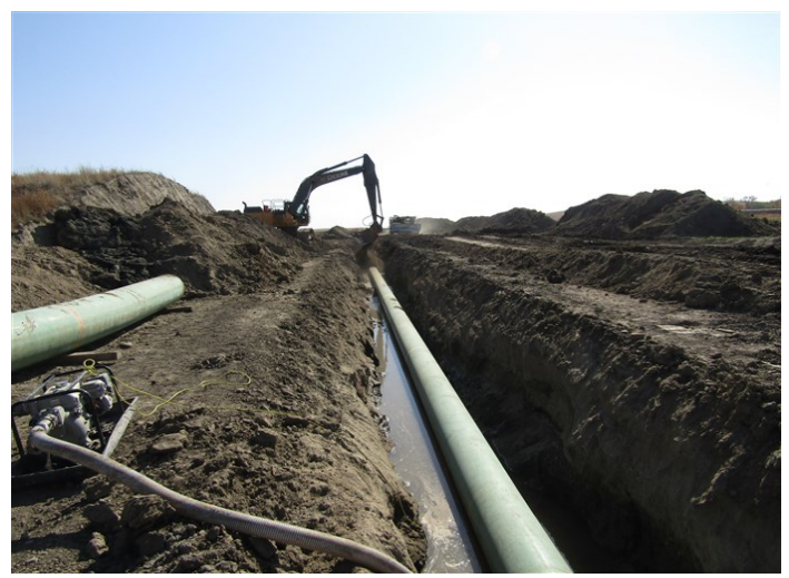
Tioga Elkhorn Creek PL Spread 2 – Small engine inside secondary containment used to pump groundwater from the open ditch (September 28, 2021) – Acceptable – MP 30.8
