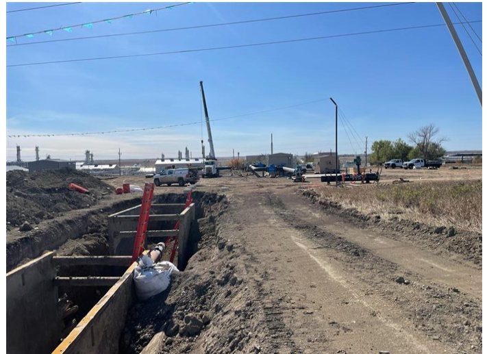
Tioga Plant Receipt Station – Ongoing installation of meter building and meter run piping (September 30, 2021) – Acceptable – MP 0.0
