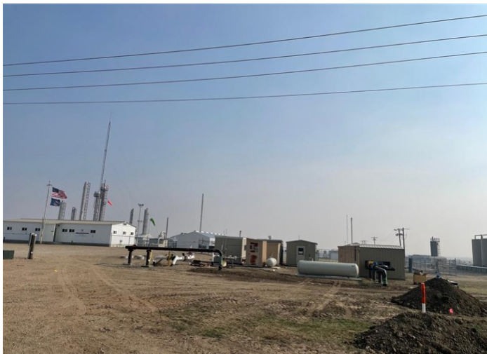
Lignite Plan Receipt and Town Border Station – Ongoing installation of the new facility meter building and piping (October 2, 2021) – Acceptable – MP 0.0
