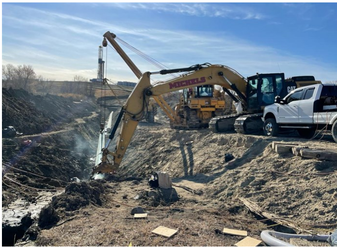
Tioga Elkhorn Creek PL Spread 1 – Bore installation is complete under 60 th Street NW and tie-in to mainline is underway (October 1, 2021) – Acceptable – MP 12.2
