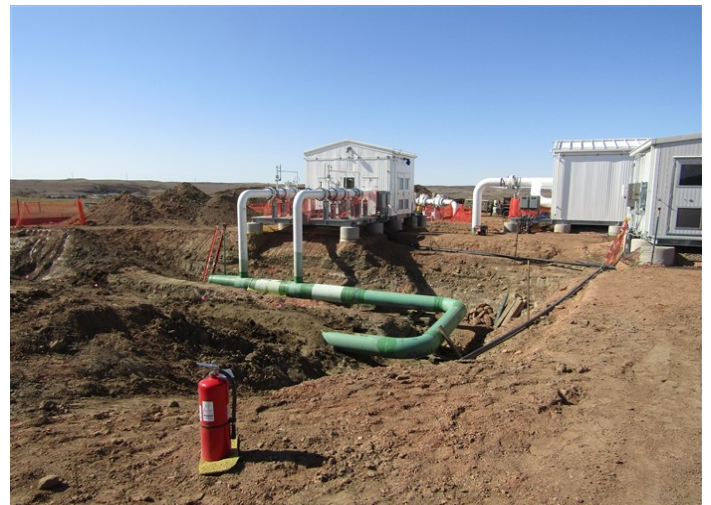
Northern Border Interconnect – Bell hole excavated and pipe installed, welded, sandblasted, and painted at the meter station (October 2, 2021) – Acceptable – MP 0.3
