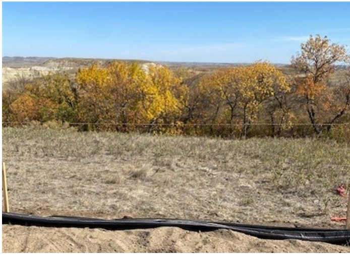
Silt fence down on the east side of the right-of-way (September 27, 2021) – Communication – MP 58.1
