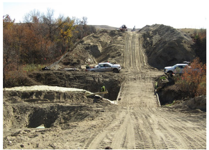
Tioga Elkhorn Creek PL Spread 2 – Mat bridge with associated erosion control devices installed crossing stream s-mk-eb-001 (October 1, 2021) – Acceptable – MP 27.1
