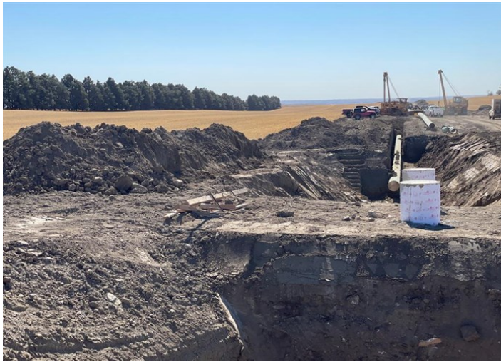
Tioga Elkhorn Creek PL Spread 1 – Concrete supports for the new 56 th Street NW block valve (October 2, 2021) – Acceptable – MP 16.2
