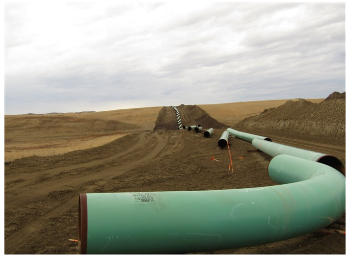
Tioga Elkhorn Creek PL Spread 2 – The right-of-way was graded and topsoil stored on the western side of the limits of disturbance. Pipe stored and strung on skids (September 29, 2021) – Acceptable – MP 53.4
