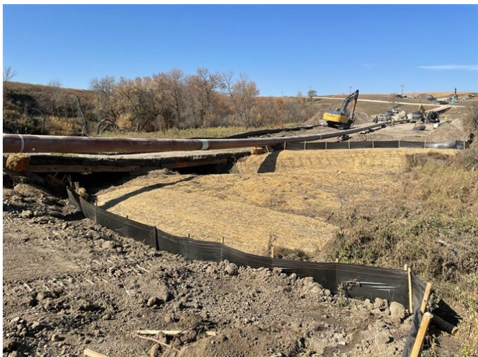
Tioga Elkhorn Creek PL Spread 1 – Restored waterbody s-wm-ee-001 after installation across the channel (September 28, 2021) – Acceptable – MP 12.3
