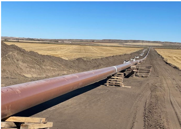
Lake Sakakawea HDD North – Assembly of pull-back section staged along the false right-of-way (September 25, 2021) – Acceptable – MP 19.8
