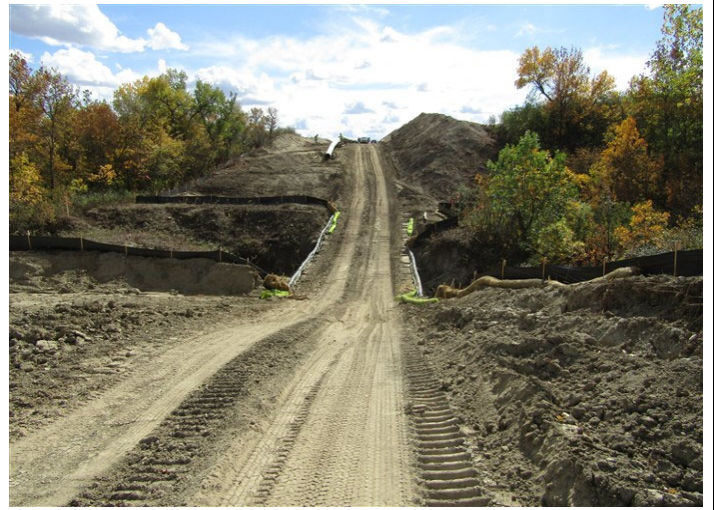
Tioga Elkhorn Creek PL Spread 2 – Mat bridge installed crossing stream s-mk-eb-001. Erosion control devices were installed (September 20, 2021) – Acceptable – MP 27.1
