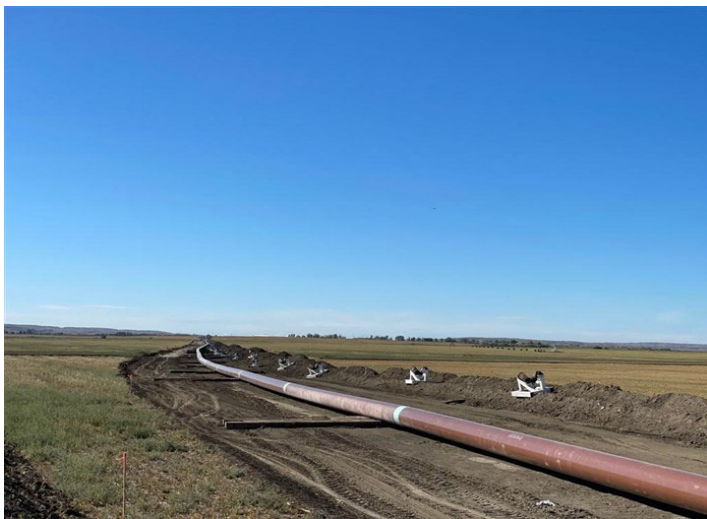
Lake Sakakawea HDD North – Pull-back section of pipeline for the Lake Sakakawea HDD (September 21, 2021) – Acceptable – MP 20.8
