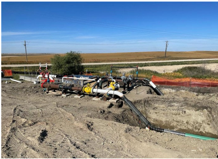
Line Section 30 Loop – New Line Section 30 Loop pipeline tied-in to the launcher and receiver setting at MP 0.0 (September 23, 2021) – Acceptable – MP 0.0
