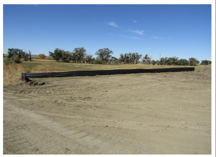
Tioga Elkhorn Creek PL Spread 2 – Erosion control devices installed at the limits of disturbance where access road AR-27 enters the right-of-way. (September 21, 2021) – Acceptable – MP 38.3
