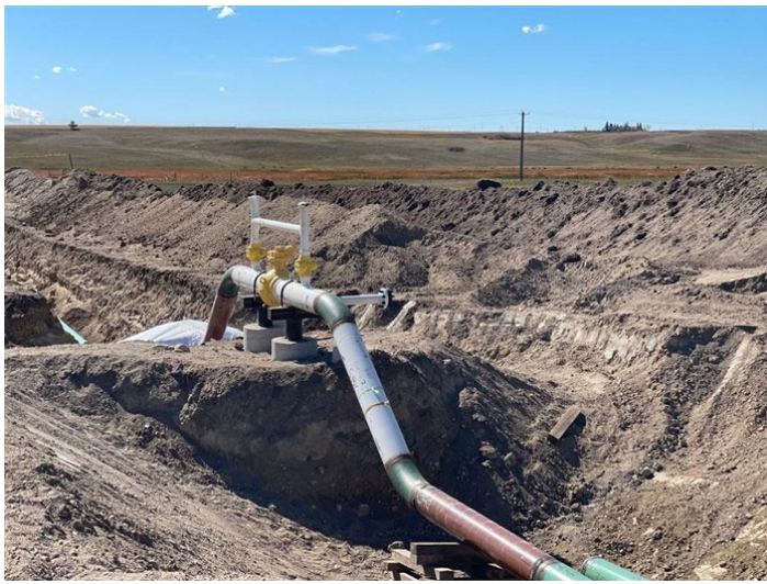
Line Section 25 Loop – Block Valve No. 13.6 of the Line Section 25 Loop (September 23, 2021) – Acceptable – MP 13.6
