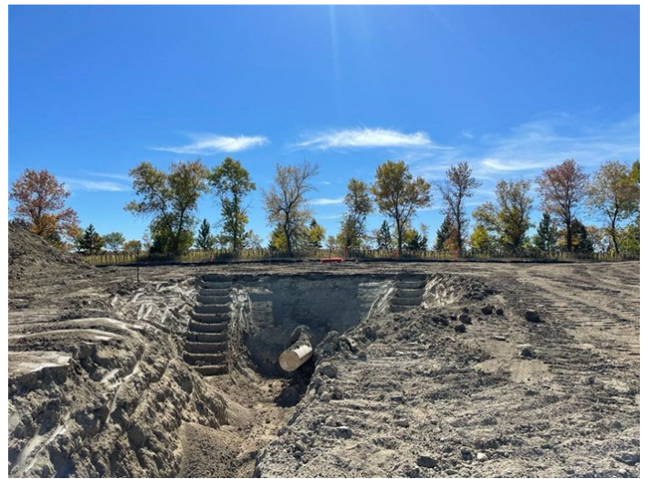
Tioga Elkhorn Creek PL Spread 1 – Completed bore under tree line and private driveway pending tie-in to the mainline (September 24, 2021) – Acceptable – MP 5.0
