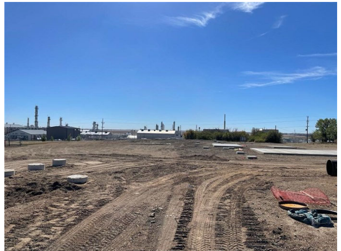
Tioga Compressor Lateral – Concrete pads and supports for the Tioga Plant Receipt Station (September 23, 2021) – Acceptable – MP 0.0
