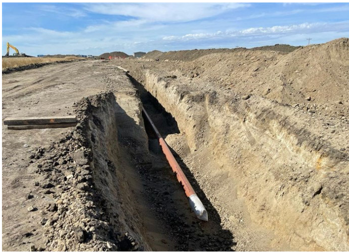
Norse Plant Receipt Station – Newly installed 8-inch-diameter pipeline through the relocation route (September 24, 2021) – Acceptable – MP 0.2
