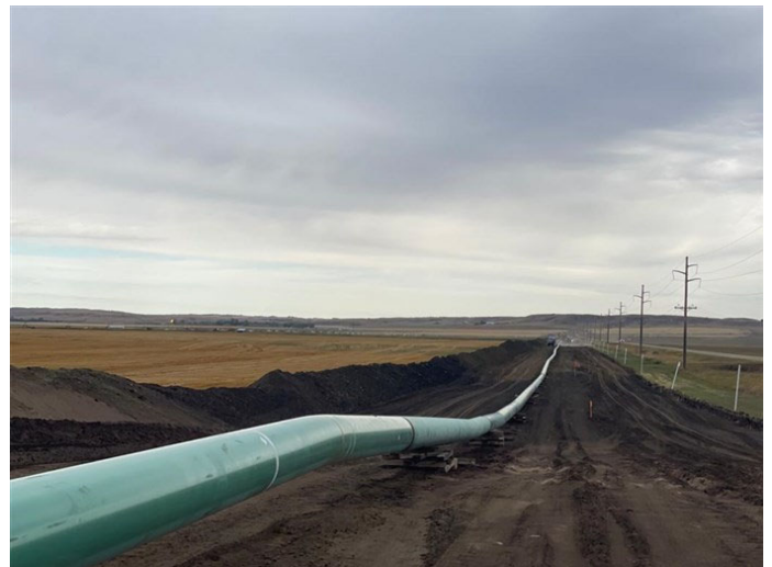
Tioga Elkhorn Creek PL Spread 1 – Assembly phase of the 24-inch diameter pipeline for the Spread is complete (September 16, 2021) – Acceptable – MP 21.6
