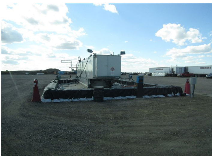
Laydown Yard – Laydown Yard (Southern Spread) – Fuel storage tank with adequate secondary containment (September 14, 2021) – Acceptable – MP 0.0
