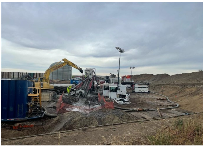
Lake Sakakawea HDD North – Initial pilot bore under Lake Sakakawea nearing completion (September 16, 2021) – Acceptable – MP 23.2
