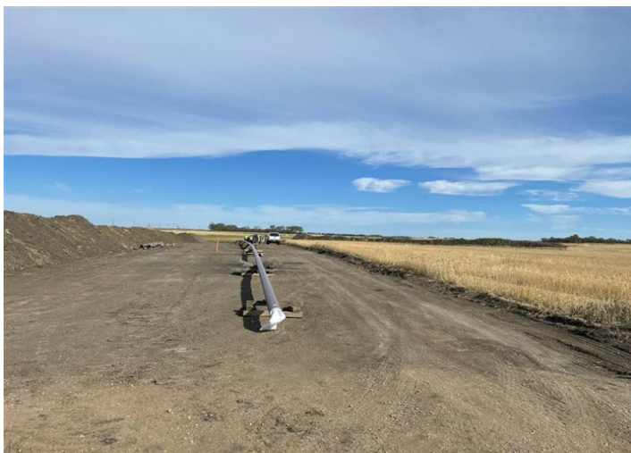
Lignite Plant Receipt and Town Border Station – 8-inch diameter pipeline for the Lignite-McGregor relocation (September 18, 2021) – Acceptable – MP 0.0
