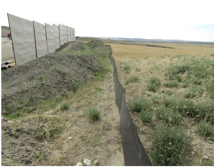
Lake Sakakawea HDD South – Erosion control devices installed at the limits of disturbance behind sound barrier adjacent to topsoil storage (September 15, 2021) – Acceptable – MP 25.9
