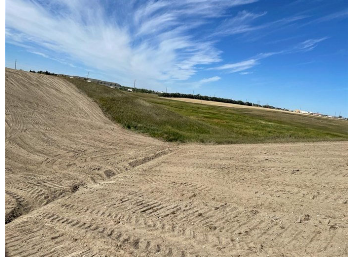
Line Section 30 Loop – Permanent slope breakers (September 15, 2021) – Acceptable – MP 6.6
