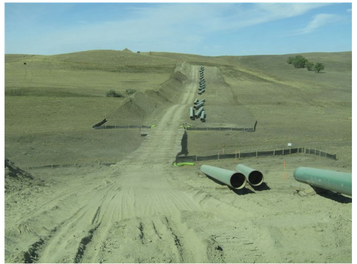
Tioga Elkhorn Creek PL Spread 2 – Right-of-way graded and topsoil stored at the limits of disturbance with pipe strung (September 17, 2021) – Acceptable – MP 54.5
