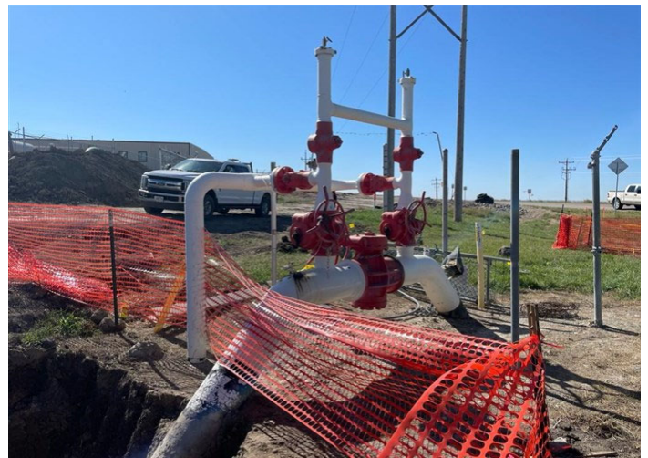
Temple Valve Setting – Old Temple Valve to be removed after installation of new valve setting with greater capacity (September 8, 2021) – Acceptable – MP 0.0
