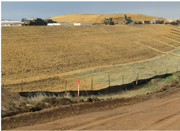
Elkhorn Compressor Station – Site limits of disturbance hydro-mulched along with erosion control devices installed at the steep drop (September 11, 2021) – Acceptable – MP 61.7
