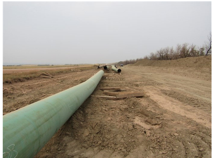
Tioga Elkhorn Creek PL Spread 2 – Pipe was strung and stacked on skids in preparation for welding activities. (September 10, 2021) – Acceptable – MP 26.7
