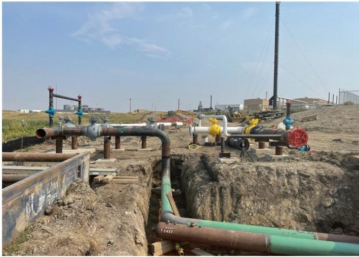
Other – Temple Valve piping and launcher and receiver at the Line Section 30 Loop (September 10, 2021) – Acceptable – MP 0.0
