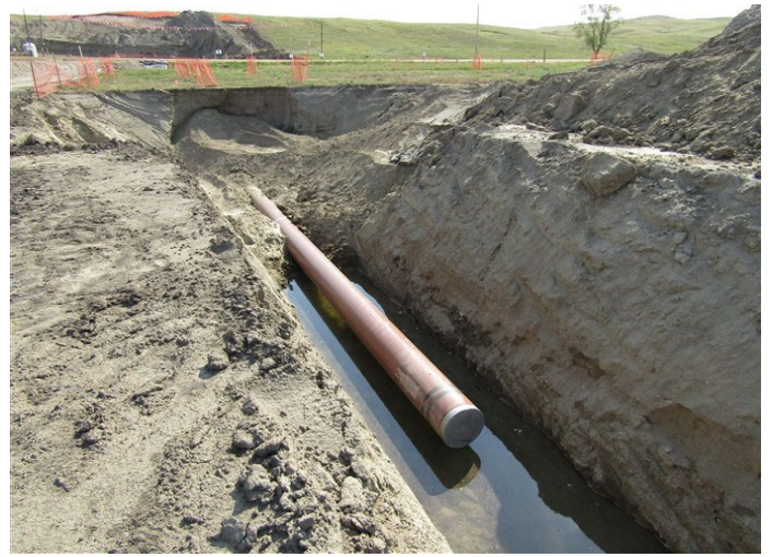
Tioga Elkhorn Creek PL Spread 2 – Bore pipe pulled under County Highway 43. Pipe capped and ditch left open for pending tie-in (September 7, 2021) – Acceptable – MP 29.8
