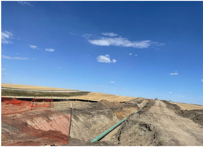
Line Section 25 Loop – Pipeline installation under two existing foreign pipelines (September 7, 2021) – Acceptable – MP 5.8
