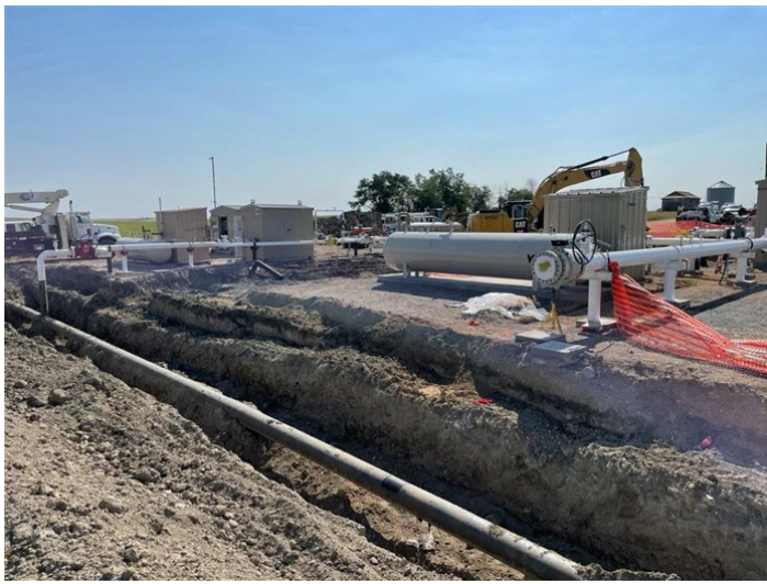
Robinson Lake Plant Receipt Station – New header piping and valve pending final installation of control valve tie-in (September 9, 2021) – Acceptable – MP 0.0
