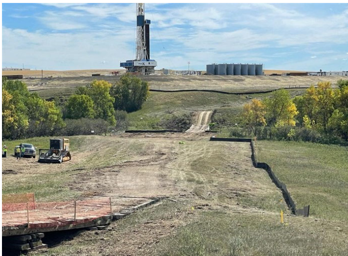
Tioga Elkhorn Creek PL Spread 1 – Temporary erosion controls and equipment bridge over wetland s-wm-ee-001 (September 8, 2021) – Acceptable – MP 12.3
