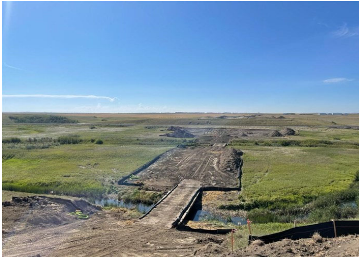
Line Section 30 Loop – Maintained erosion controls and stabilized banks of waterbody S-WM-EA-001-P (August 30, 2021) – Acceptable – MP 8.9
