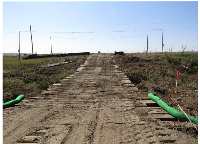
Tioga Elkhorn Creek PL Spread 2 – Mat bridge installed crossing wetland W-MK-EA-004E. Erosion control devices installed at both sides of the mat bridge. (August 30, 2021) – Acceptable – MP 46.6
