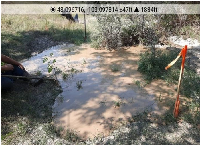
Tioga Elkhorn Creek PL Spread 2 – Inadvertent release of approximately 200 gallons of water, mud, and bentonite occurred in the dry stream bed of stream S-MK-ea-001 (Photo courtesy the Lead Environmental Inspector) (September 2, 2021) – Communication – MP 27.5
