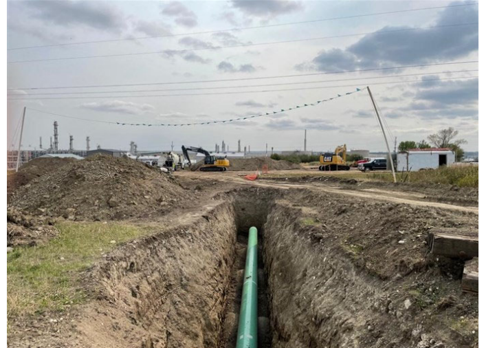
Tioga Compressor Lateral – Installation of 20-inch diameter pipeline to the new WBI Tioga Compressor Station (September 2, 2021) – Acceptable – MP 0.0
