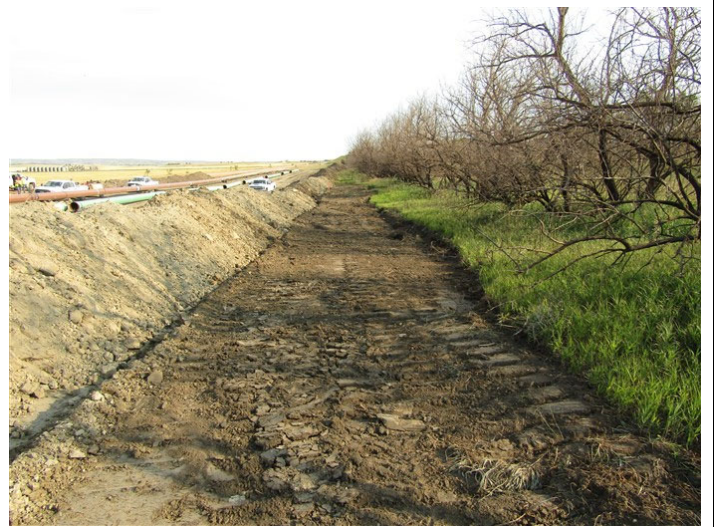
Tioga Elkhorn Creek PL Spread 2 – 9-foot x 340-foot section of right-of-way that was cleared and graded outside the limits of disturbance by the contractor (September 3, 2021) – Communication – MP 26.7
