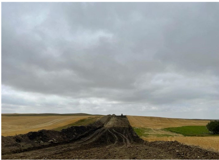
Line Section 30 Loop – Backfill and rough clean-up operations in progress (August 24, 2021) – Acceptable – MP 0.6
