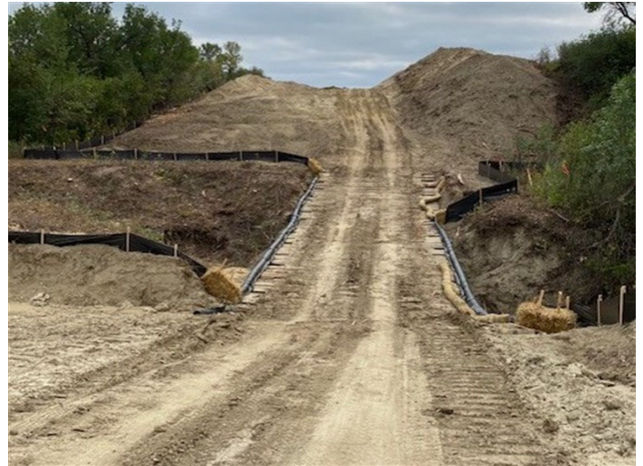
Tioga Elkhorn Creek PL Spread 2 – Mat bridge along with associated erosion control devices installed at stream S-MK-eb-001 (August 26, 2021) – Acceptable – MP 27.1
