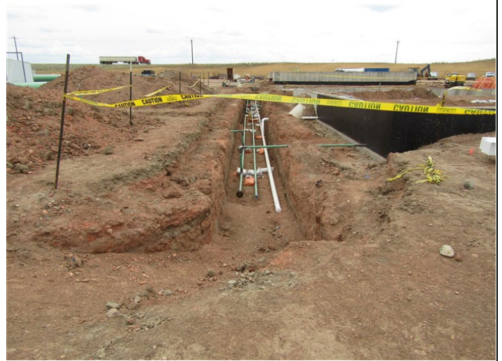
Elkhorn Compressor Station – Small pipes installed at the Elkhorn Compressor Station (August 28, 2021) – Acceptable – MP 61.7
