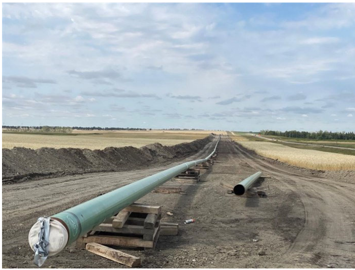
Line Section 25 Loop – Long segments of pipeline assembled, coated, and inspected (August 25, 2021) – Acceptable – MP 17.0
