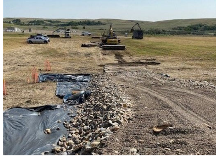
Tioga Elkhorn Creek PL Spread 2 – Rock and associated erosion control devices installed on the south side of the road crossing at State Highway 23. Mats being installed beyond the rock entrance for vehicle and equipment travel (August 23, 2021) – Acceptable – MP 50.9
