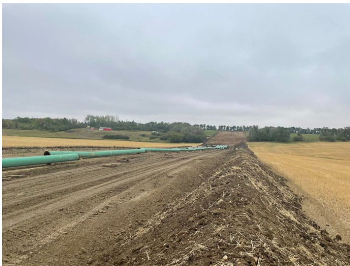
Tioga Elkhorn Creek PL Spread 1 – Pipe segments strung (August 28, 2021) – Acceptable – MP 4.7
