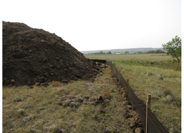
Tioga Elkhorn Creek PL Spread 2 – Topsoil pile removed from bore pad stored and erosion control devices installed at the limits of disturbance (August 27, 2021) – Acceptable – MP 27.4
