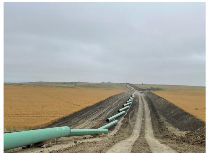
Tioga Elkhorn Creek PL Spread 1 – Pipeline joints strung through cultivated fields (August 24, 2021) – Acceptable – MP 14.6
