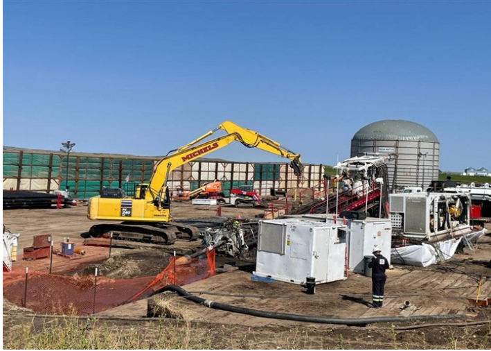
Tioga Elkhorn Creek PL Spread 1 – On-going drilling activities on the north side of Lake Sakakawea (August 23, 2021) – Acceptable – MP 23.0
