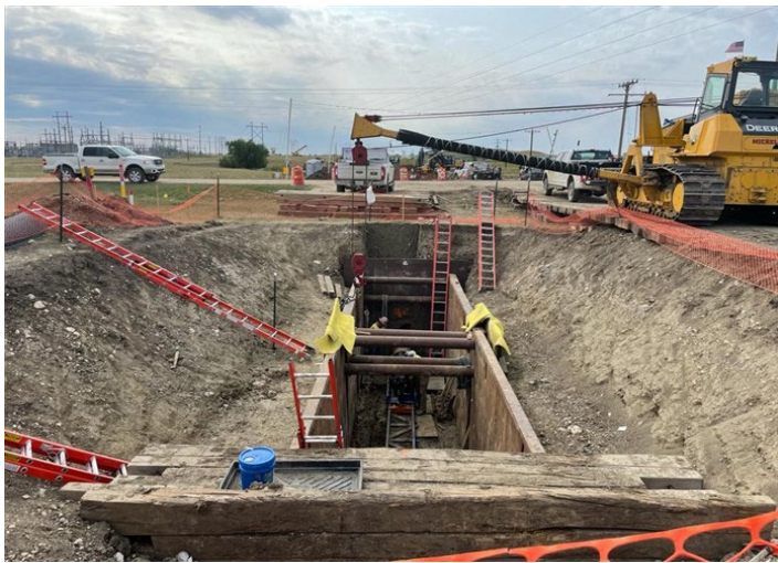
Tioga Compressor Lateral – Guided bore installation process under 103 rd Avenue NW for the Tioga Compressor Lateral (August 27, 2021) – Acceptable – MP 0.4
