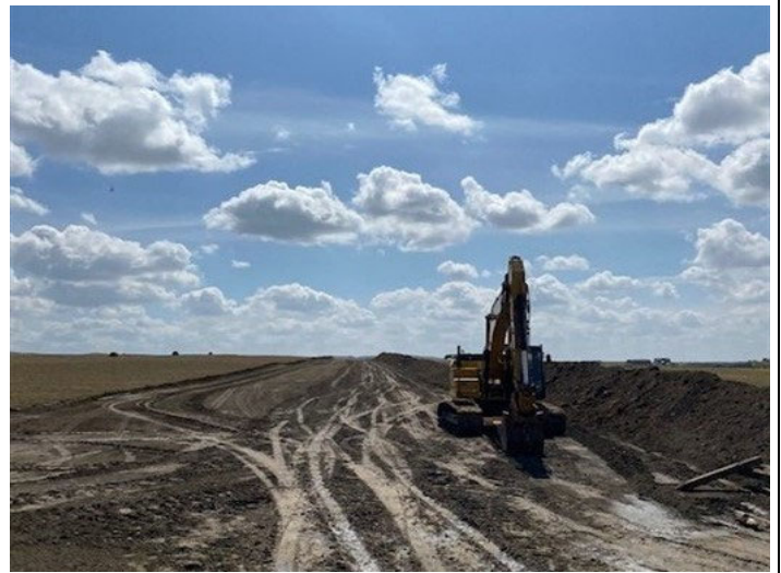
Tioga Elkhorn Creek Pipeline Spread 2 – Right-of-way graded from Station No. 1464+10 to Station No. 1470+00. Equipment properly parked overnight, 100 feet from any resource (August 21, 2021) – Acceptable – MP 27.7
