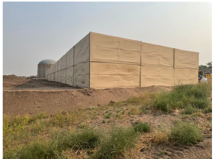
Tioga Elkhorn Creek Pipeline Spread 1 – Temporary sound-limiting wall (August 16, 2021) – Acceptable – MP 23.0
