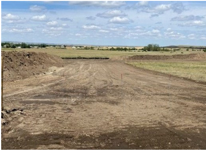
Tioga Elkhorn Creek Pipeline Spread 2 – Right-of-way has been graded and topsoil stored in the limits of disturbance. Erosion control devices were installed for stormwater run-off protection and filtration (August 21, 2021) – Acceptable – MP 27.7
