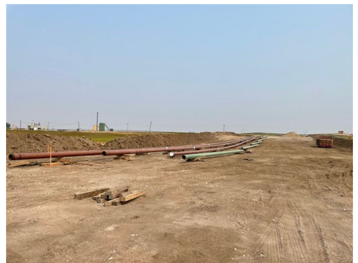
Line Section 25 Loop – Topsoil segregated and adequately stored within the approved work areas (August 17, 2021) – Acceptable – MP 14.0
