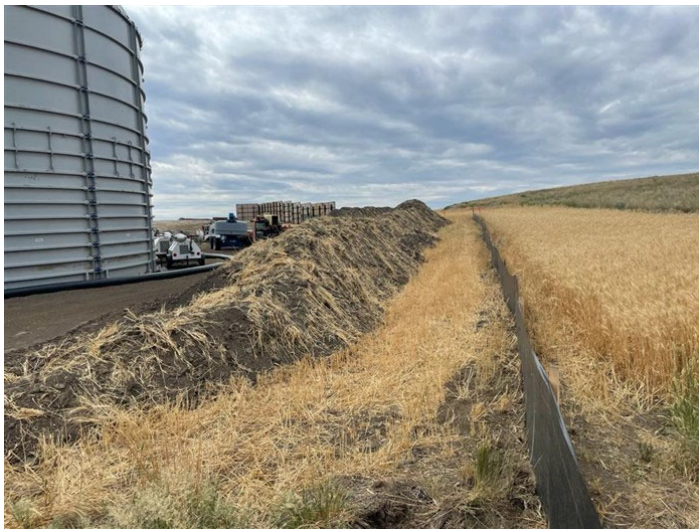
Tioga Elkhorn Creek PL Spread 2 – Topsoil segregated and stored within the approved workspace (August 11, 2021) – Acceptable – MP 25.9
