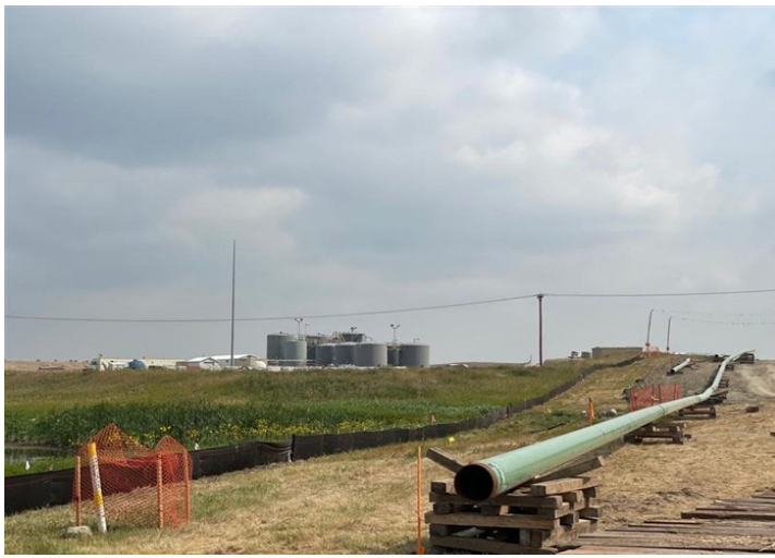
Line Section 30 Loop – On-going process of pipeline assembly at the Section Line 30 Loop (August 9, 2021) – Acceptable – MP 0.3
