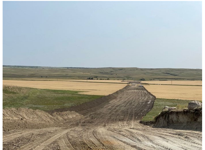
Tioga Elkhorn Creek PL Spread 1 – Topsoil stripped and segregated through cultivated fields (August 9, 2021) – Acceptable – MP 18.9
