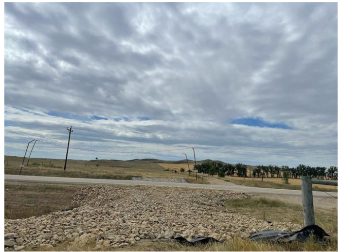
Tioga Elkhorn Creek PL Spread 2 – Rip-rap rock over synthetic fabric at rock construction entrance (August 11, 2021) – Acceptable – MP 36.3
