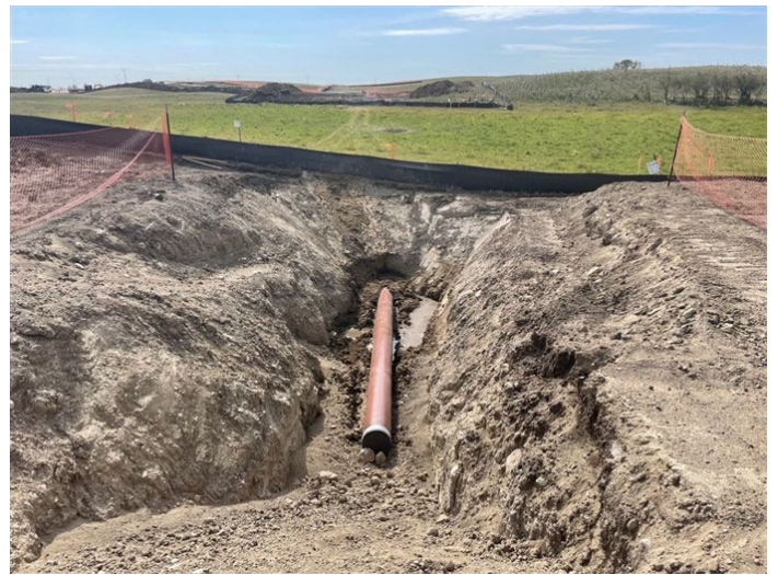
Line Section 25 Loop – Section of abrasion-resistant coated pipeline (August 13, 2021) – Acceptable – MP 0.4
