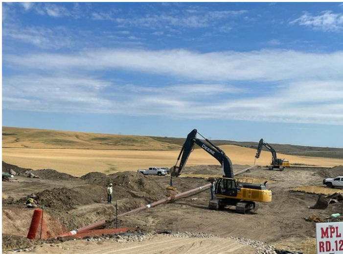
Line Section 25 Loop – Installation process under 73 rd Street NW and 103 rd Avenue NW (August 14, 2021) – Acceptable – MP 2.1
