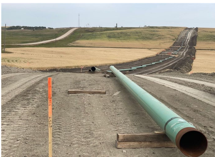
Tioga Elkhorn Creek PL Spread 1 – Joints of pre-coated pipe secured along the right-of-way (August 10, 2021) – Acceptable – MP 2.1
