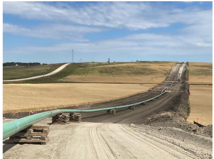
Line Section 25 Loop – Assembled extensive section of pipeline of Line Section 25 Loop (August 14, 2021) – Acceptable – MP 2.2
