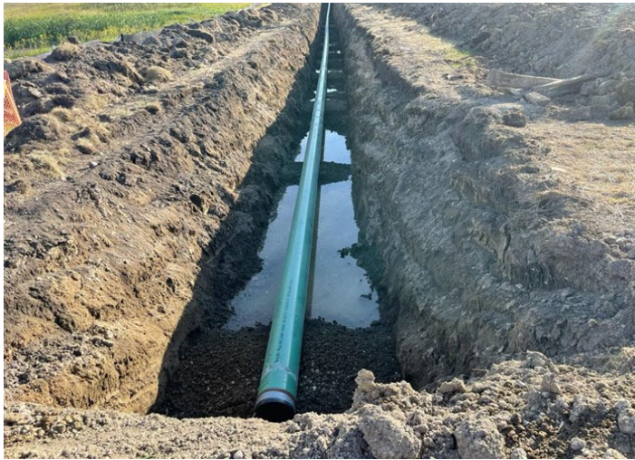
Line Section 30 Loop – Pipeline lowered-in over padded trench spoil (August 13, 2021) – Acceptable – MP 0.2
