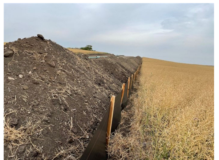
Tioga Elkhorn Creek Spread 1 – Topsoil and adequately installed silt fence (August 10, 2021) – Acceptable – MP 2.6
