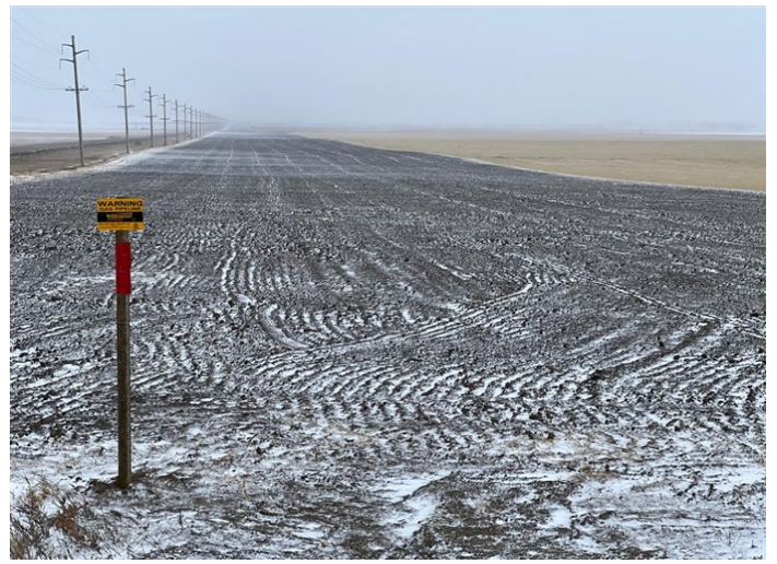
Tioga Elkhorn Creek PL Spread 1 – Topsoil replaced through hayfields utilized for pullback assembly (November 11, 2021) – Acceptable – MP 20.1
