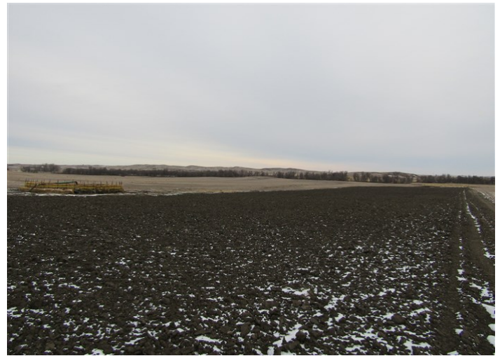
Tioga Elkhorn Creek PL Spread 2 – Right-of-way with final clean-up activities completed, both sides blended in, and contours restored. Hydro-testing dewatering structure with all associated erosion control devices installed for dewatering activities (November 12, 2021) – Acceptable – MP 44.3
