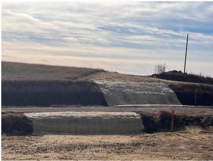
Uprates Line to Section 25 – Permanent erosion controls on both sides of the uprates bore pipeline crossing of 92 nd Street NW (November 9, 2021) – Acceptable – MP 0.0
