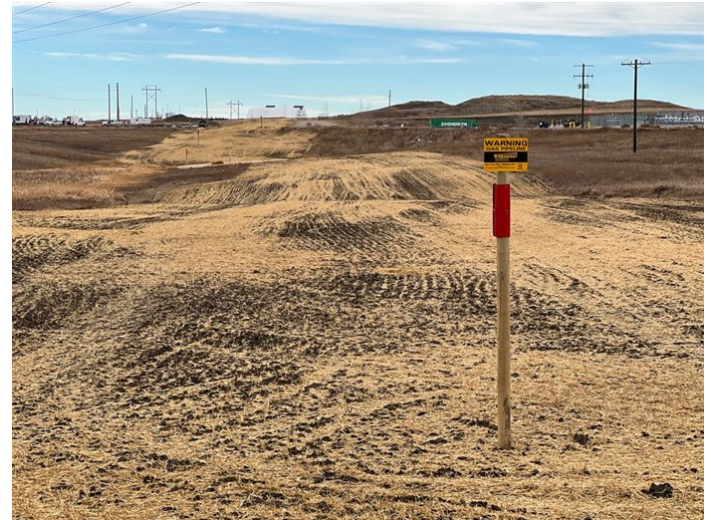
Tioga Compressor Lateral – Cleaned, restored, seeded, and mulched construction right-of-way (November 9, 2021) – Acceptable – MP 0.4
