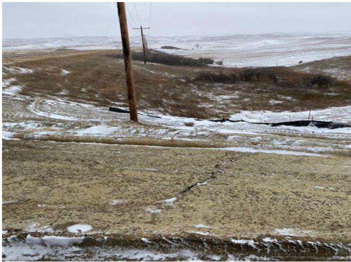
Northern Border Interconnect – Erosion control devices installed at the slope on the northern side of the access road into the Northern Border Interconnect site (November 11, 2021) – Acceptable – MP 0.3
