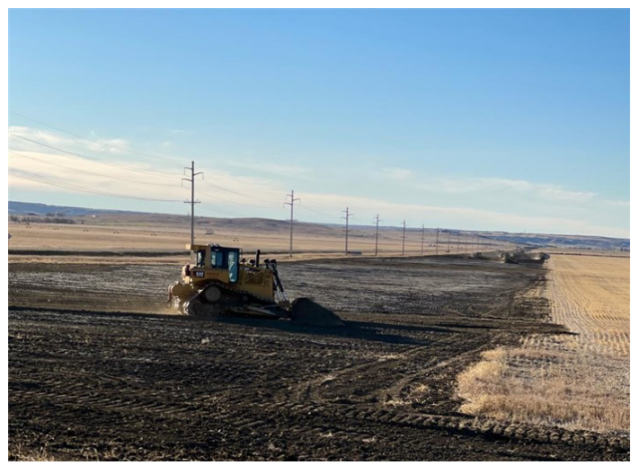
Lake Sakakawea HDD North – Topsoil replacement through temporary workspaces on the false right-of-way (November 8, 2021) – Acceptable – MP 22.0
