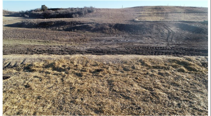
Tioga Elkhorn Creek PL Spread 2 – Final clean-up conducted on the right-of-way. The right-of-way has been seeded and mulched (November 3, 2021) – Acceptable – MP 54.5
