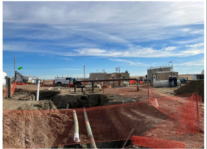
Uprates to Line Section 25 – Pig launcher at Lignite Receipt Plant yet to be completed (November 4, 2021) – Communication – MP 0.0
