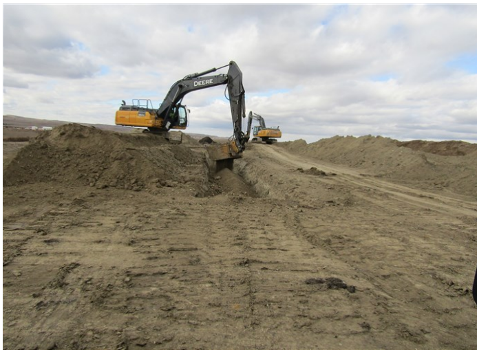
Elkhorn Creek Compressor Station – Lowering-in and backfilling pipe between the Elkhorn Creek Compressor Station and the Northern Border (November 1, 2021) – Acceptable – MP 0.1
