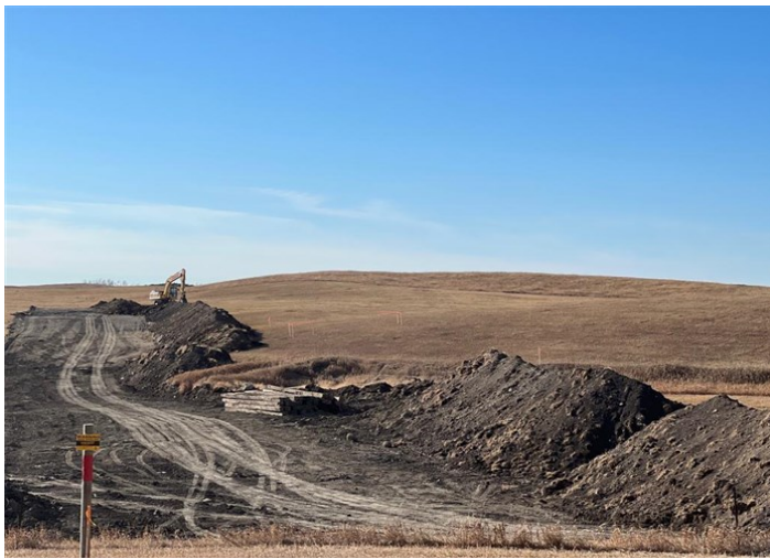
Uprates to Line Section 25 – Topsoil replacement on-going on the south side of State Highway 40 (November 6, 2021) – Acceptable – MP 0.0
