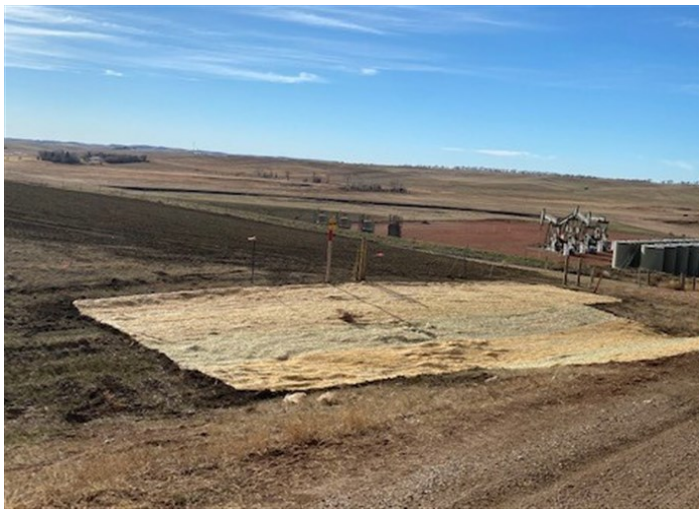
Tioga Elkhorn Creek PL Spread 2 – Curlex installed on the south side of 25 th Avenue N bar ditch for stabilization (November 5, 2021) – Acceptable – MP 53.5
