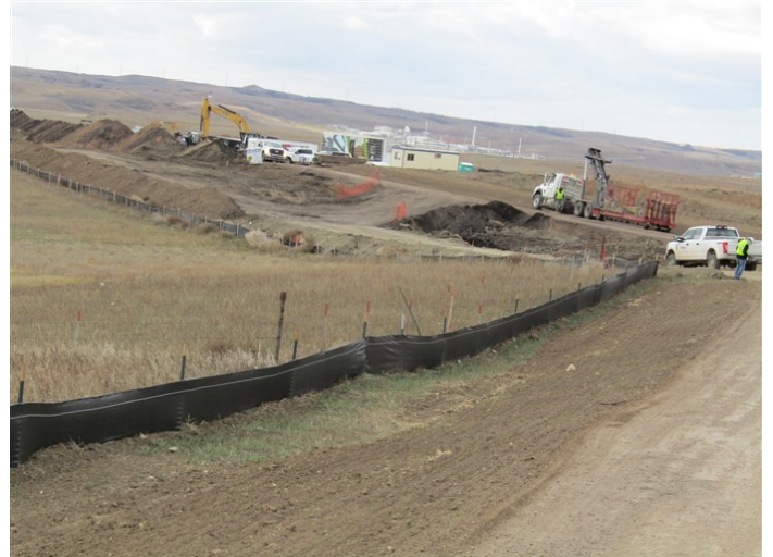
Elkhorn Creek Compressor Station – Erosion control devices installed on the west side of access road into the Northern Border site (November 1, 2021) – Acceptable – MP 0.3
