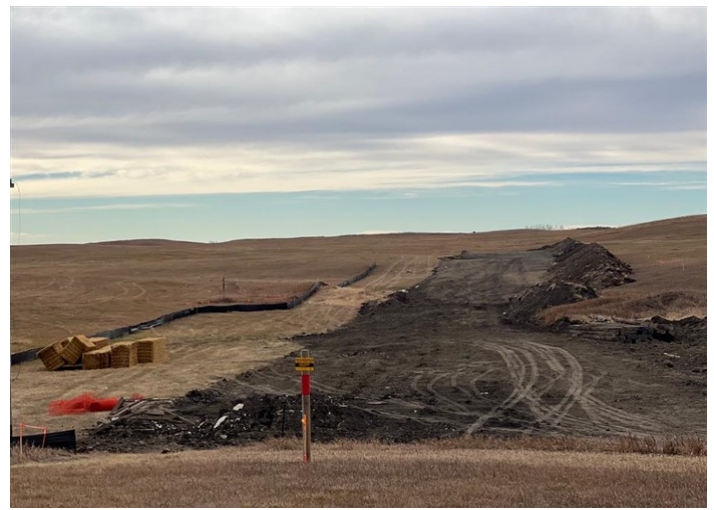
Uprates to Line Section 25 – Backfill process completed at the bore crossing of State Highway 40 (November 5, 2021) – Communication – MP 0.0
