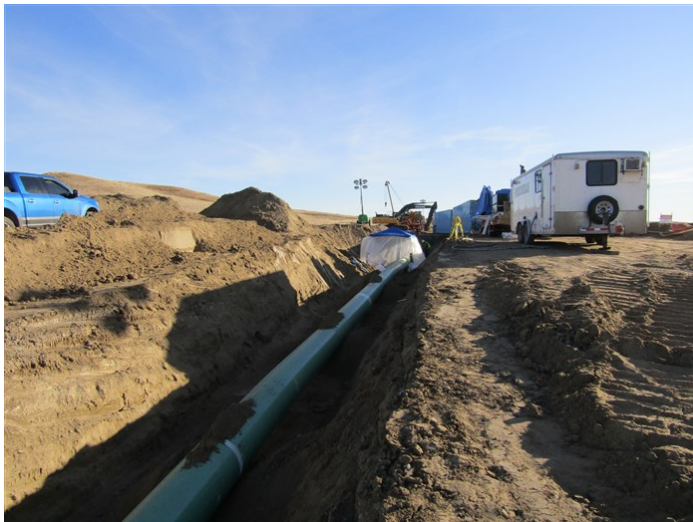
Lake Sakakawea HDD South – Open ditch with pipe test header installed and used for hydro-testing (November 2, 2021) – Acceptable – MP 25.9
