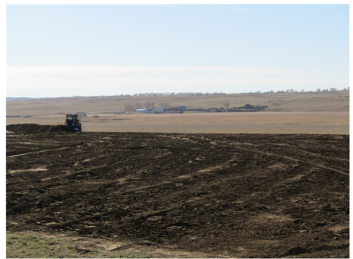
Tioga Elkhorn Creek PL Spread 2 – Topsoil put back across the right-of-way on the south side of 121 st Avenue NW (November 2, 2021) – Acceptable – MP 49.1
