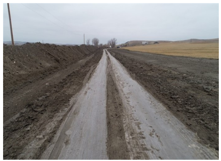
Tioga Elkhorn Creek PL Spread 2 – Pipe has been lowered-in and backfilled from this area of the right-of-way at the 121st Avenue NW road crossing to the private drive ahead (October 30, 2021) – Acceptable – MP 38.8
