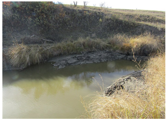
Tioga Elkhorn Creek PL Spread 2 – Buckle in the stream bed and at both sides of the stream banks at stream crossing S-IBT-001A (October 29, 2021) – Communication – MP 51.9
