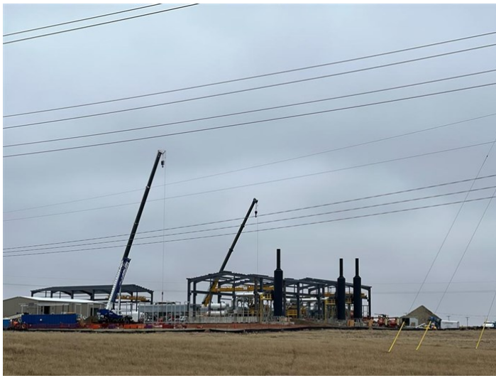
Tioga Compressor Station – Ongoing installation of the compressor buildings (October 26, 2021) – Acceptable – MP 0.0
