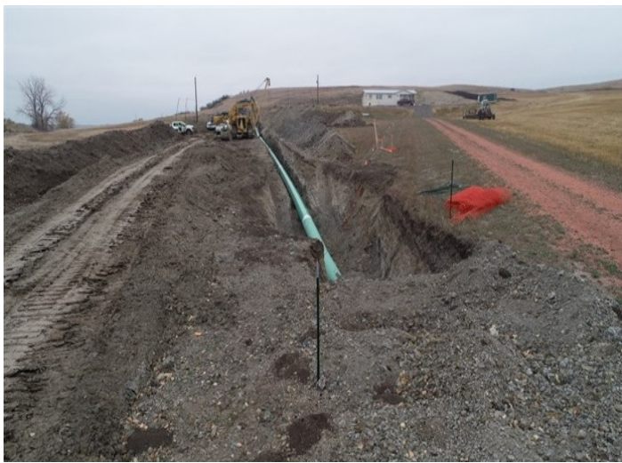
Tioga Elkhorn Creek PL Spread 2 – Pipe has been tied in and lowering-in activities conducted. This pipe section is connected to the wetland w-mk-ea-003e bore section (October 30, 2021) – Acceptable – MP 38.4
