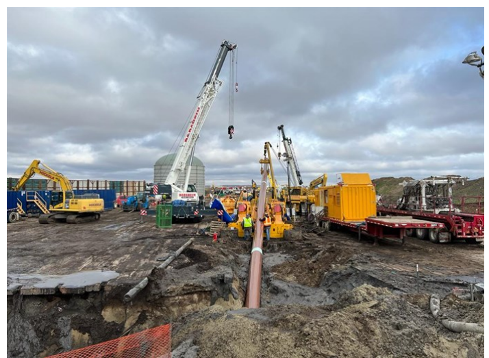
Lake Sakakawea HDD North – Completed pull-back and approximately 130 feet of additional pipeline to be cut off (October 25, 2021) – Acceptable – MP 23.1
