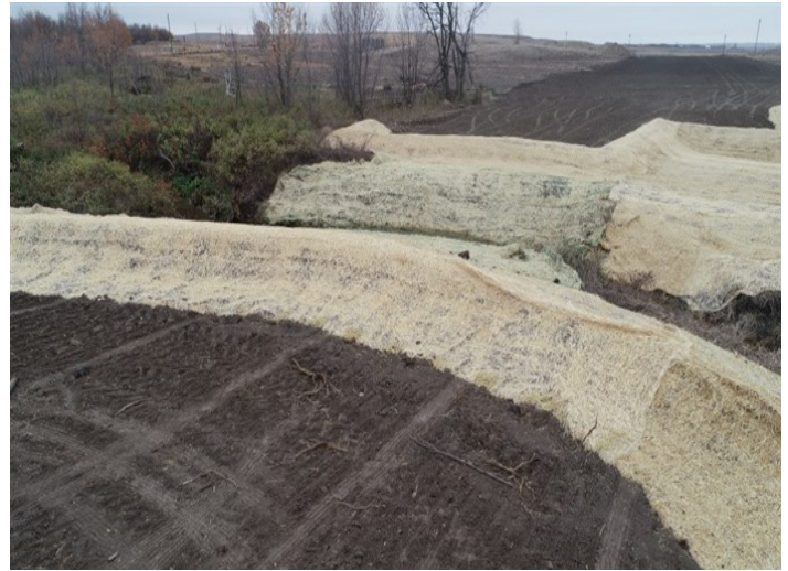
Tioga Elkhorn Creek PL Spread 2 – Banks and contours of stream s-mk-ea-002 restored. Curlex installed on the banks for stabilization (October 26, 2021) – Acceptable – MP 39.0
