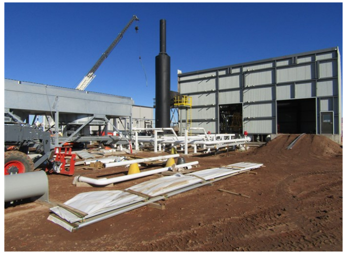
Elkhorn Creek Compressor Station – Piping being installed, sandblasted, and coated at the compressor building area (October 27, 2021) – Acceptable – MP 61.7
