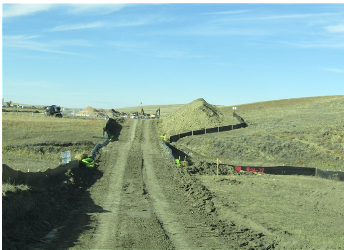
Tioga Elkhorn Creek PL Spread 2 – Mat bridge with associated erosion control devices installed crossing stream s-mk-eb-005 (October 29, 2021) – Acceptable – MP 51.1
