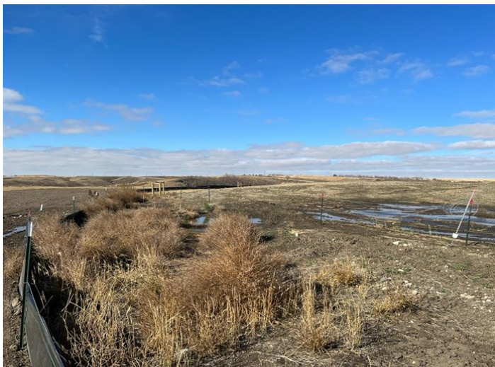
Tioga Elkhorn Creek PL Spread 1 – Faulty erosion controls at an adjacent non-Project area (October 19, 2021) – Communication – MP 12.3
