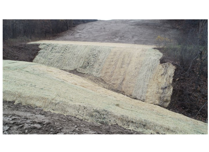
Tioga Elkhorn Creek PL Spread 2 – Curlex installed on the slope breaker at stream s-mk-eb-001. Banks of stream put back and contours restored to the original condition (October 19, 2021) – Acceptable – MP 27.1
