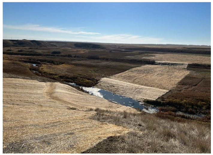
Tioga Elkhorn Creek PL Spread 1– Slope breakers and erosion blankets on both sides of stream s-wm-ea-001p (October 18, 2021) – Acceptable – MP 3.3
