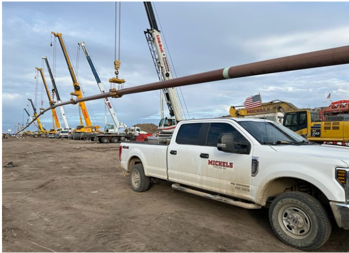
Lake Sakakawea HDD North – Elevated pipeline ready for pullback (October 23, 2021) – Acceptable – MP 23.0
