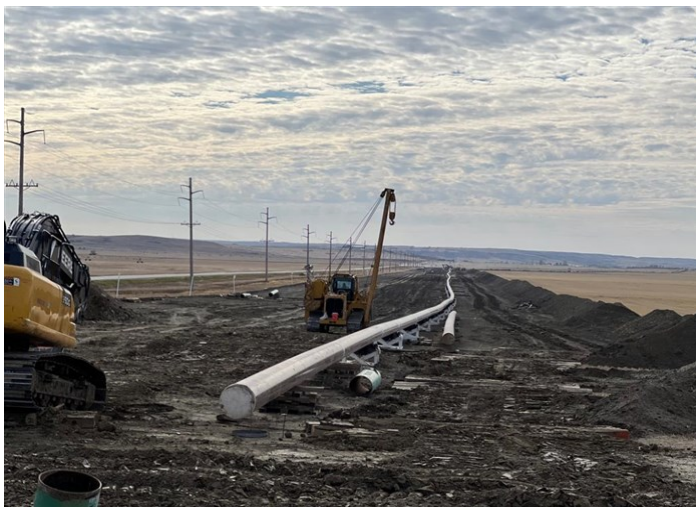
Lake Sakakawea HDD North – 235 joints of abrasion-resistant pipe welded together ready for installation (October 23, 2021) – Acceptable – MP 19.9
