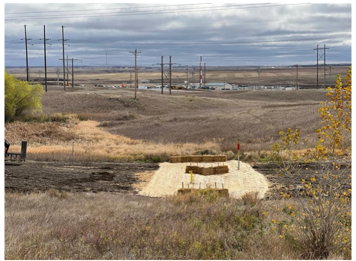
Tioga Compressor Lateral – Permanent erosion controls over a drainage swale across the Tioga Lateral right-of-way (October 21, 2021) – Acceptable – MP 0.3
