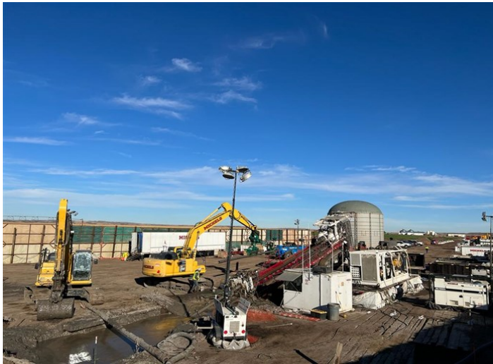
Lake Sakakawea HDD North – Ongoing drilling operations with a swab head along the pipeline pad at the Lake (October 18, 2021) – Acceptable – MP 23.0
