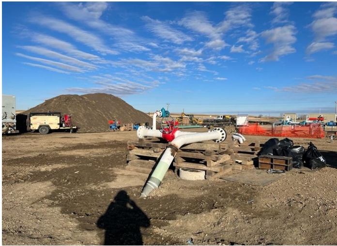
Norse Plant Receipt Station – 8-inch diameter piping headers to replace the existing 6-inch diameter pipeline to increase capacity and transmission (October 22, 2021) – Communication – MP 0.0
