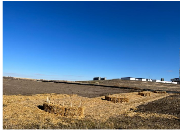
Tioga Elkhorn Creek PL Spread 1 – Environmental crews implemented corrective actions and additional measures to control erosion caused by non-Project sources (October 22, 2021) – Acceptable – MP 12.3
