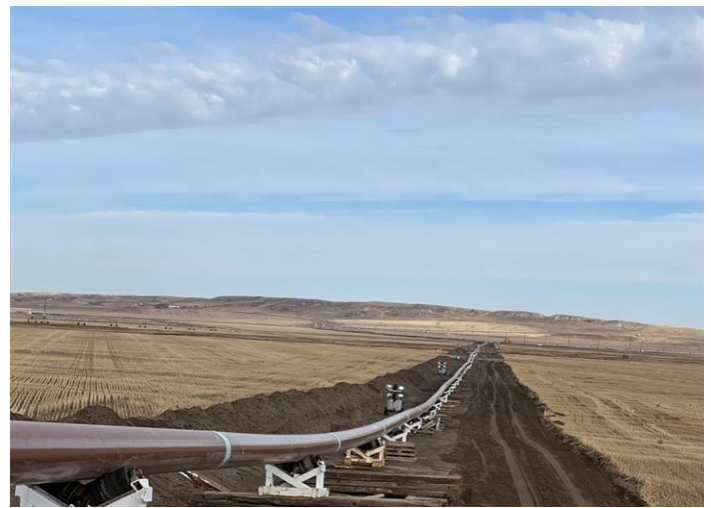
Lake Sakakawea HDD North – Approximately 600 rubber-roller skids supporting the pre-fabricated segments of pipeline (October 23, 2021) – Acceptable – MP 19.9
