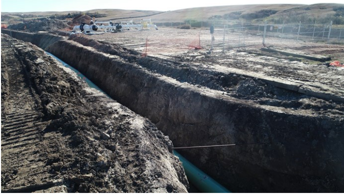
Tioga to Elkhorn Creek Spread 2 – Pipe lowered into trench (October 16, 2021) – Acceptable – MP 51.0
