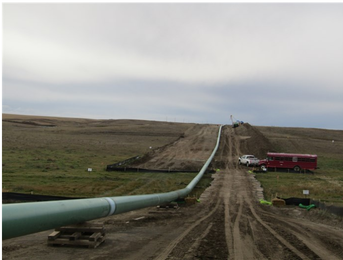
Tioga to Elkhorn Creek Spread 2 – Mat bridge and welded pipe at wetland w-mk-wa-002e (October 12, 2021) – Acceptable – MP 53.2
