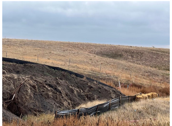
Lake Sakakawea HDD North – Erosion control devices installed (October 14, 2021) – Acceptable – MP 23.2
