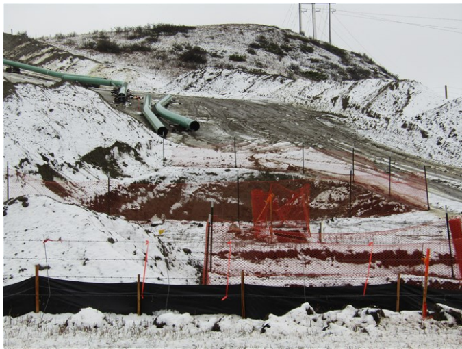
Tioga to Elkhorn Creek Spread 2 – Pipe welded, erosion control devices installed. Snowy conditions (October 13, 2021) – Acceptable – MP 58.1
