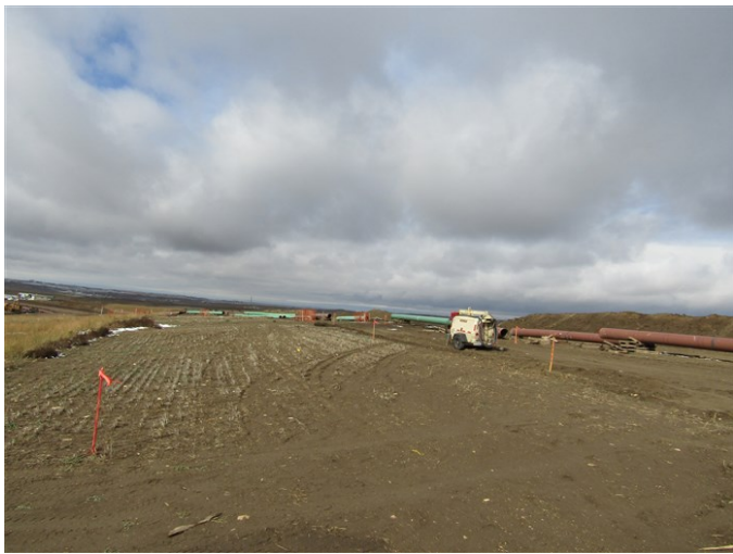
Northern Border Interconnect – Right-of-way graded and topsoil segregated. Pipe stored on skids and prepared for welding (October 14, 2021) – Acceptable – MP 0.2
