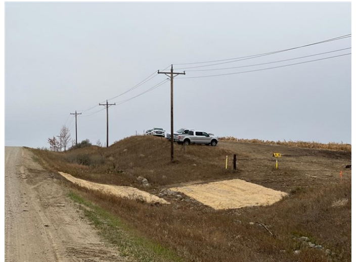
Tioga to Elkhorn Creek Spread 1 – Restoration and installation of erosion control blankets at bar ditch (October 12, 2021) – Acceptable – MP 11.9
