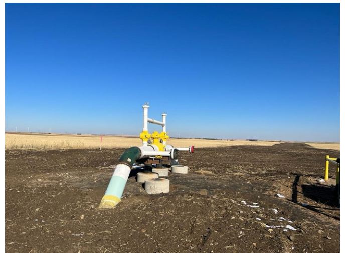
Line Section 25 Loop – Mainline valve 6.8 is installed (October 16, 2021) – Acceptable – MP 6.8
