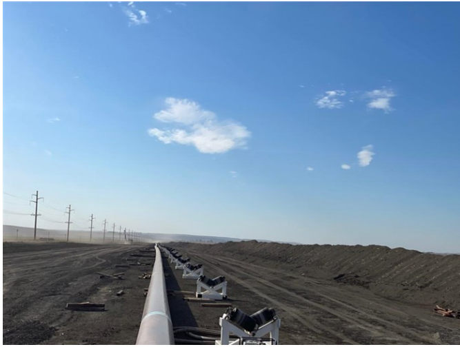
Lake Sakakawea HDD North - Pipe welded and ready to be placed on rollers (October 11, 2021) – Acceptable – MP 19.9
