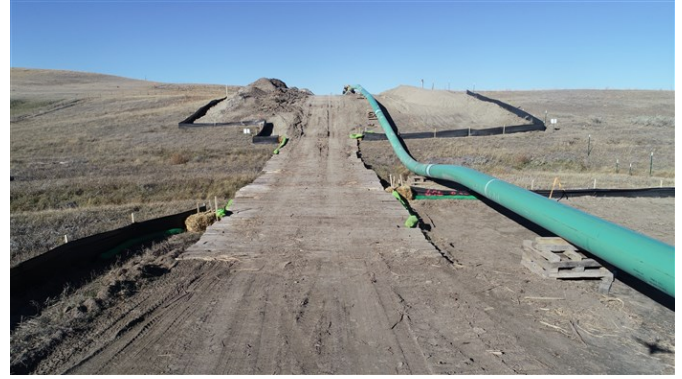
Tioga to Elkhorn Creek Spread 2 – Equipment bridge installed at wetland w-mk-eb-006e. Pipe welded and erosion control devices installed (October 16, 2021) – Acceptable – MP 55.2
