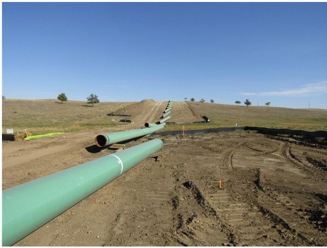
Tioga Elkhorn Creel PL Spread 2 - Pipe strung and erosion control devices protecting wetland (October 4, 2021) – Acceptable – MP 58.1
