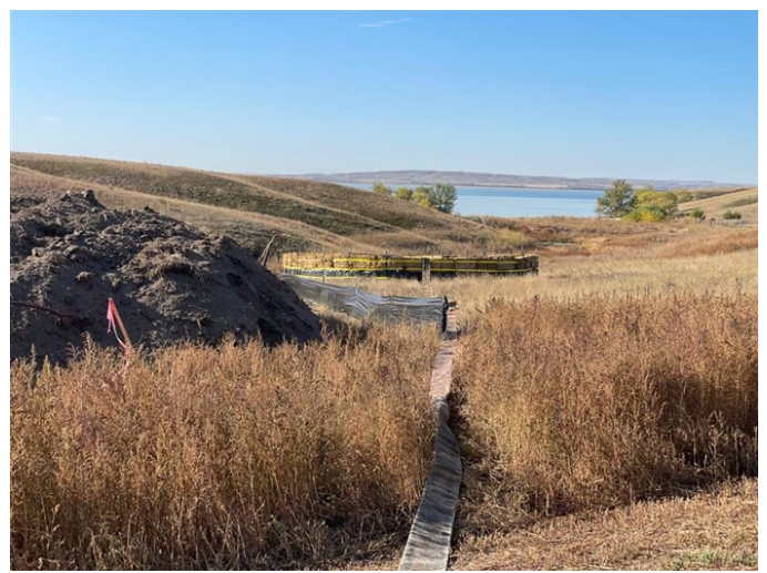
Lake Sakakawea HDD North – Layflat hose leading to dewatering structure with Lake in the background (October 5, 2021) – Acceptable – MP 23.2
