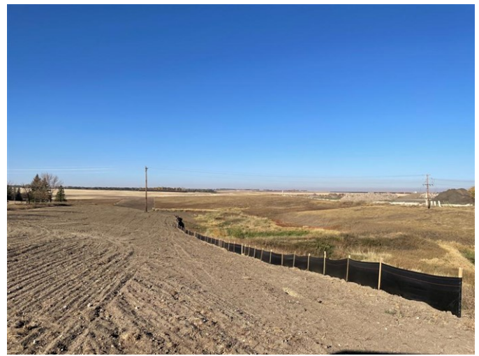
Line section 30 Loop – Restoration underway, erosion control devices installed (October 8, 2021) – Acceptable – MP 6.0
