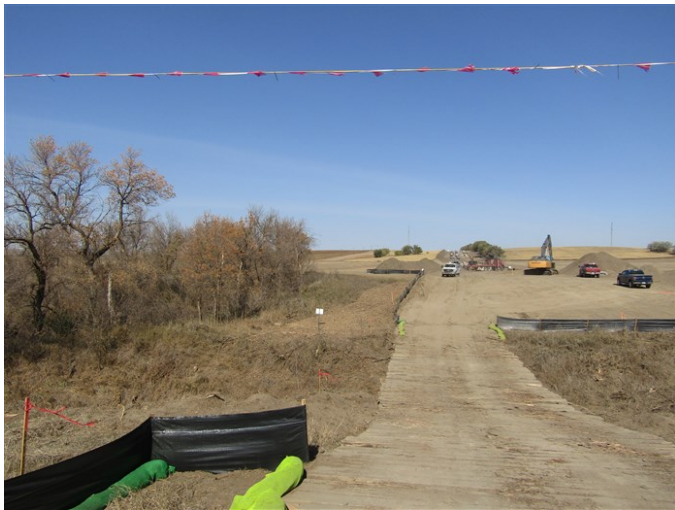
Tioga Elkhorn Creek PL Spread 2 – Mat bridge at wetland, erosion control devices in place (October 6, 2021) – Acceptable – MP 46.6
