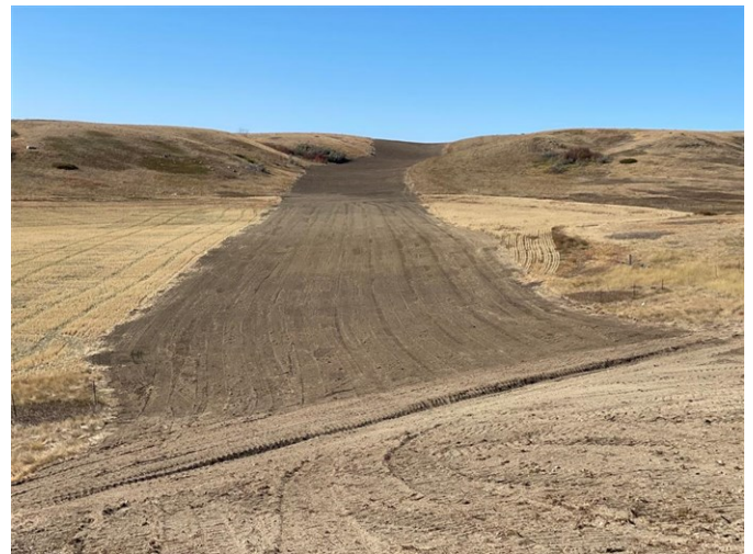
Tioga Elkhorn Creel Spread 1 – Restored right-of-way with slope breaker installed (October 8, 2021) – Acceptable – MP 18.9
