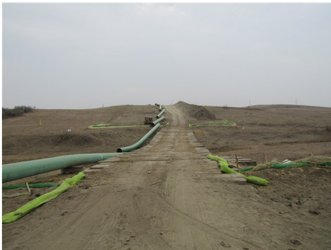
Tioga Elkhorn Creep Spread 2 – Pipe strung and mat bridge at wetland (October 8, 2021) – Acceptable – MP 54.5
