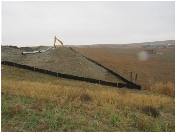
Tioga Elkhorn Creek PL Spread 2 – Pipe strung with erosion control devices installed at topsoil pile (October 9, 2021) – Acceptable – MP 54.7
