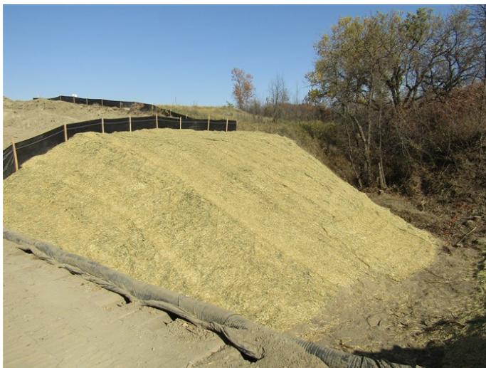
Tioga Elkhorn Creek PL Spread 2 – Erosion control devices installed and Curlex blanket on streambank (October 5, 2021) – Acceptable – MP 27.1
