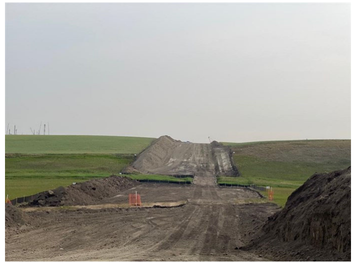
Tioga to Elkhorn Creek Pipeline Spread 1 – Equipment bridge and erosion controls at the crossing of waterbody S-WM-EA-002 (August 3, 2021) – Acceptable – MP 2.4
