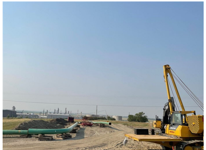
Tioga Compressor Lateral – Grading and stringing throughout the Tioga Compressor Lateral construction right-of-way is complete (August 2, 2021) – Acceptable – MP 0.0
