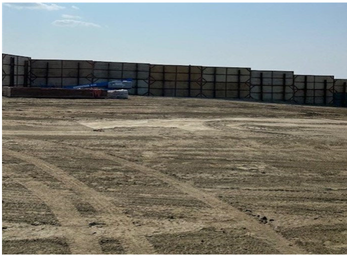
Lake Sakakawea HDD – Sound barrier curtain was installed at the Sakakawea HDD pad to minimize the noise level of HDD operations (August 5, 2021) – Acceptable – MP 25.9
