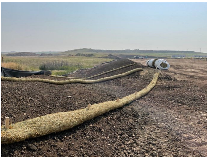
Elkhorn Compressor Station – Filter socks and silt fence along the north perimeter of the new Elkhorn Compressor Station (July 30, 2021) – Acceptable – MP 61.5
