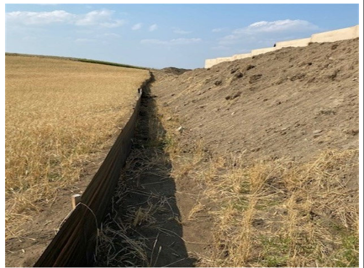
Lake Sakakawea HDD – Topsoil removed and stored at the limits of disturbance of the Sakakawea HDD (August 5, 2021) – Acceptable – MP 25.9
