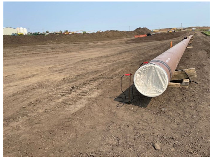
Tioga to Elkhorn Creek Pipeline Spread 1 – Abrasion resistant sections of pipeline pre-assembled for HDD installation (August 7, 2021) – Acceptable – MP 22.9
