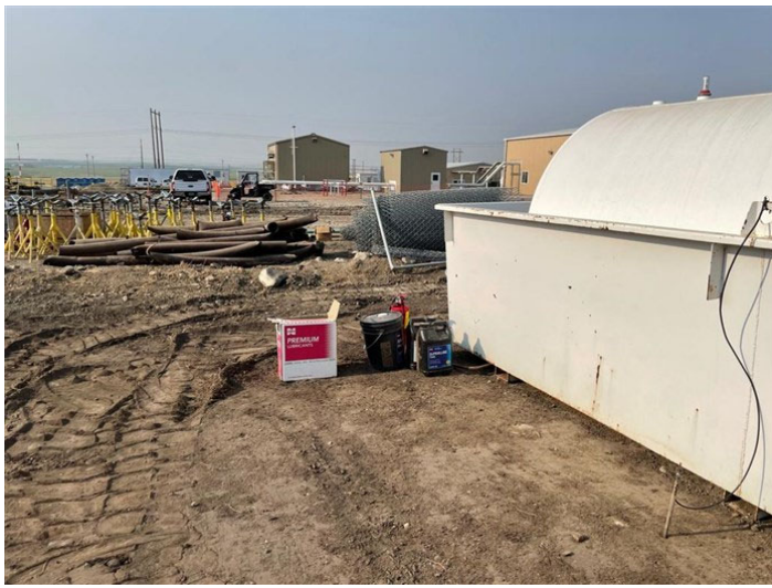
Tioga Compressor Station – Lubricants and oils stored outside of a secondary containment (July 31, 2021) – Communication – MP 0.0
