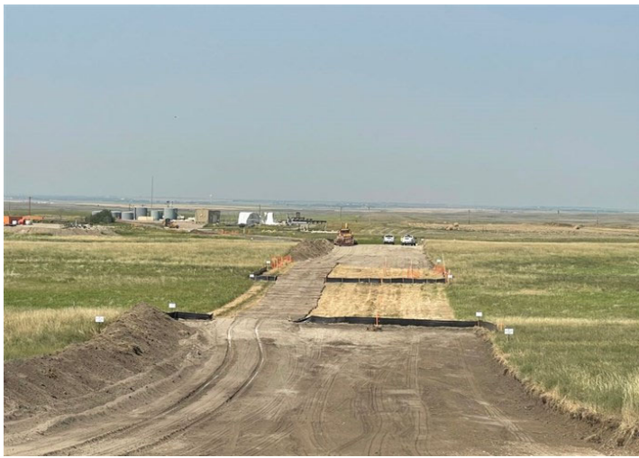
Line Section 30 Loop – Adequate erosion controls and timber mats over the travel lane at wetland W-WM-EF-004E (August 2, 2021) – Acceptable – MP 0.2
